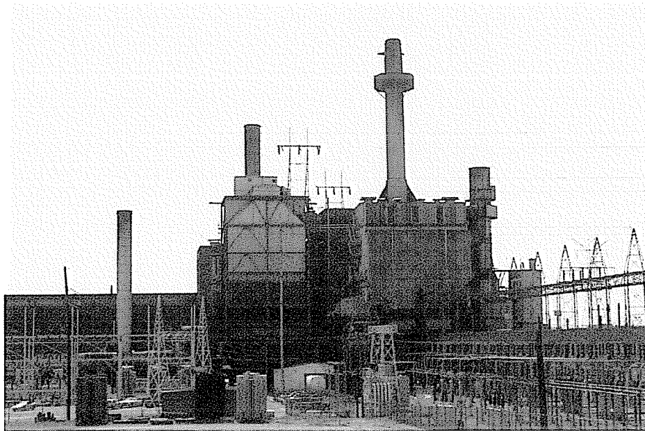
Green River Power Station (Owned by Kentucky Utilities Company)
