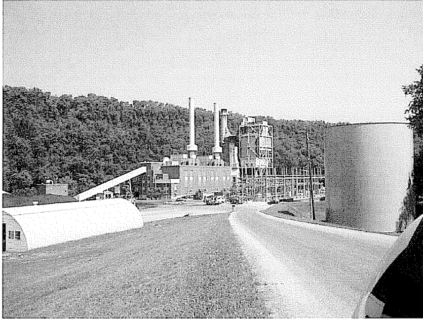
Figure 2.7-2 Tyrone Generating Station
