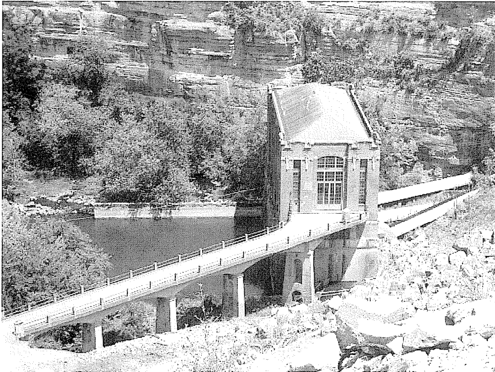
Figure 4.2-2 Dix Dam Generating Station
