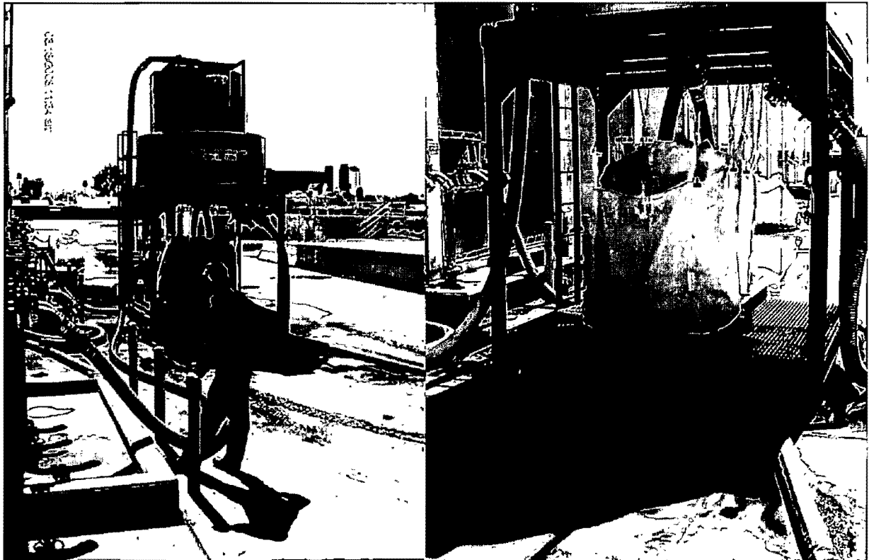
EXHIBIT 5-30 Media Removal by Eduction to Super Sacks (Provided by Calgon Carbon Corporation)
