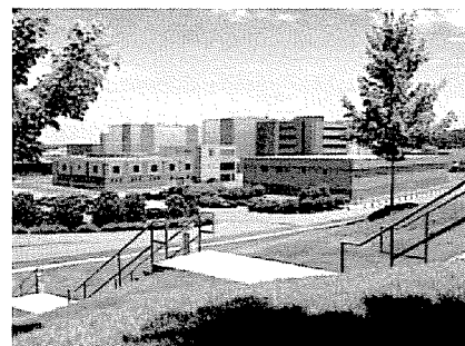
Catawba Nuclear Station in York County, S.C., set a new Duke Power reliability record in 2004, and was recognized by the U.S. Nuclear Regulatory Commission for safe operations.
