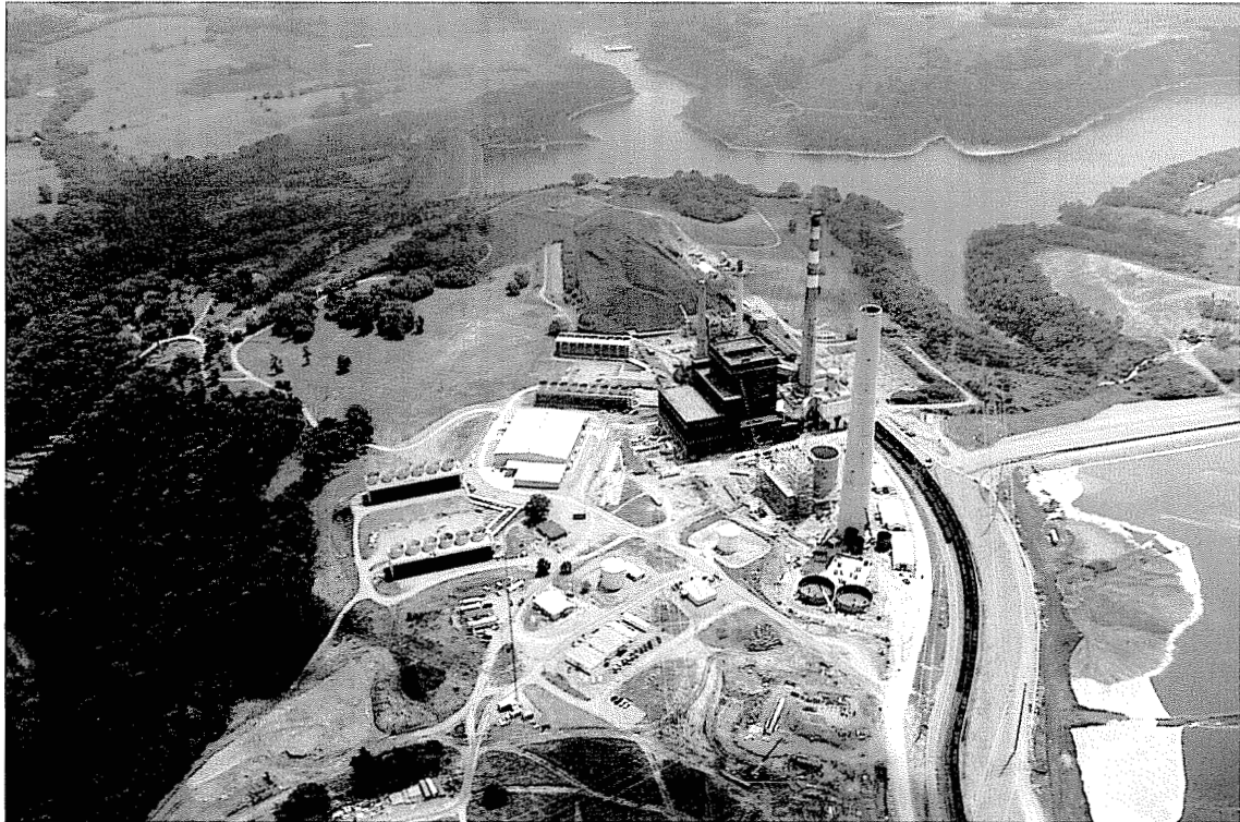
FIGURE 5-1. PHOTO WITH VIEW OF E.ON BROWN STATION LOOKING EAST SOUTHEAST
