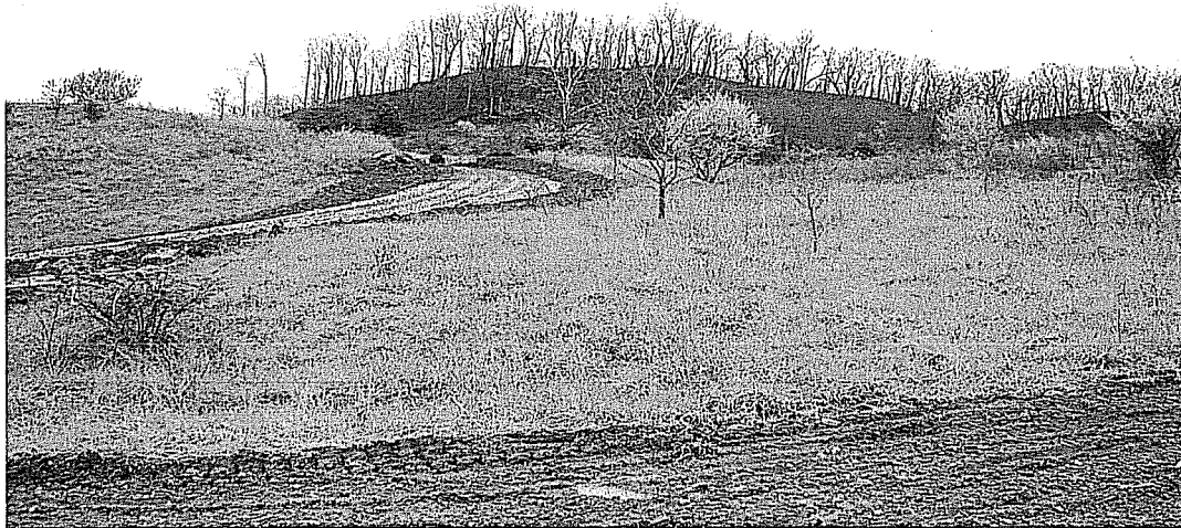
Access road to the fee tract and new road constructed through surface only tract Photo by Vance Mosley
