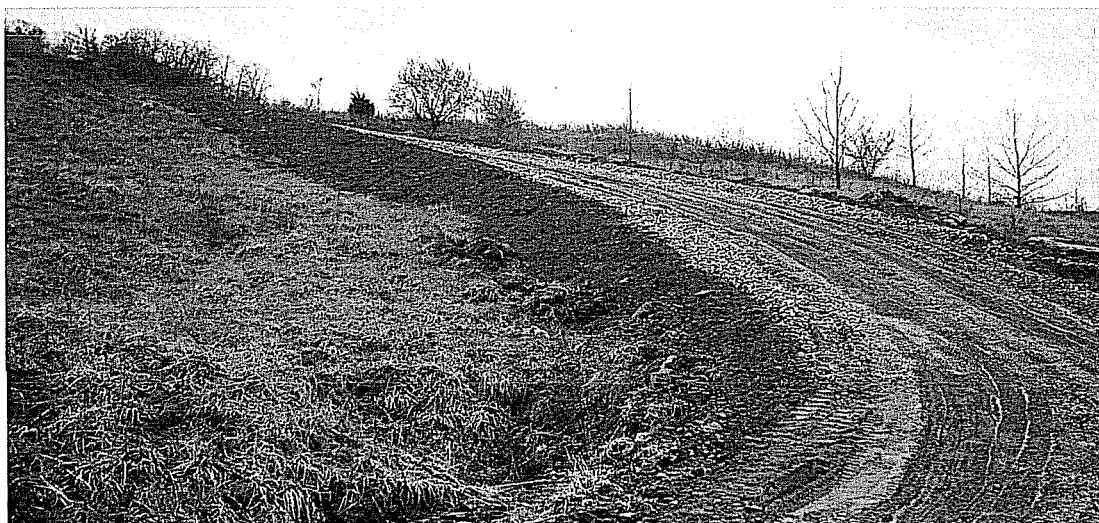
New road constructed through the subject. Photo by Vance Mosley
