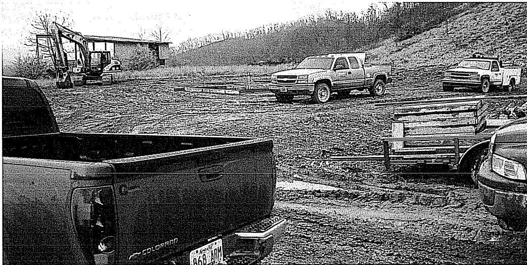
Tower site view looking Southeast. Photo by Vance Mosley
