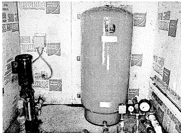
Pine Road Booster Pump Station
