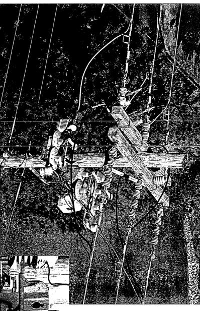
Installed digital line sensors and other equipment to create a "self-healing" network in Hendersonville, N.C.; brought online additional self-healing systems in Cincinnati Sept. 1
