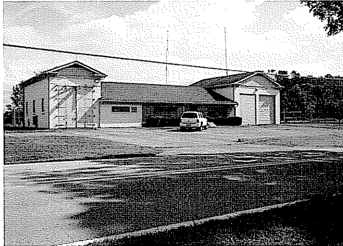
Existing Water Plant Building
