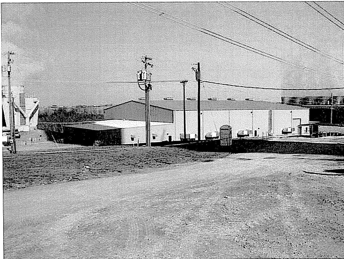
The above photo (dated 3/12/2008) shows the new warehouse.
