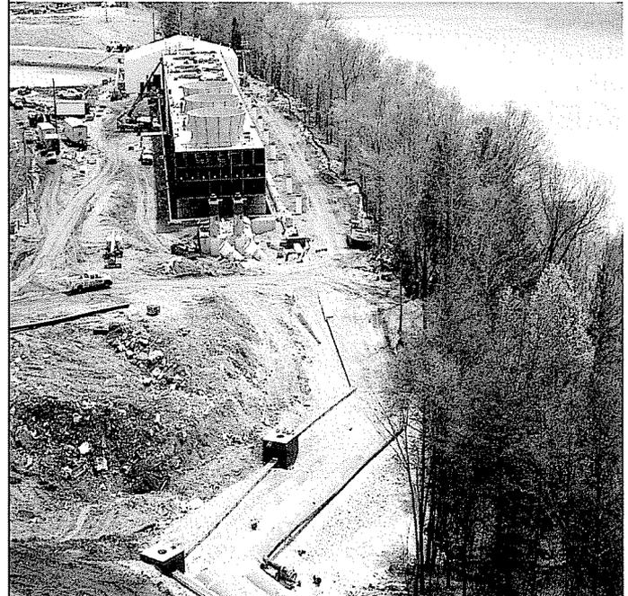
F.E. Moran has completed the installation of the sprinkler piping and the control building for the tower fire protection system. Viking will oversee the installation of the fire protection system in the service building and the supply line from the plant.
