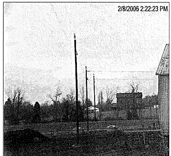
TAP LINE VICTIM WAS WORKING ON AT THE TIME OF THE ACCIDENT
