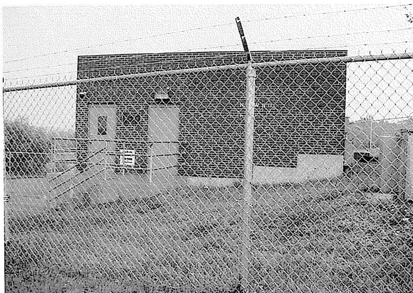
Ripple Creek Pump Station
