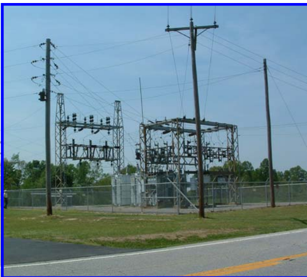
Typical distribution substation
