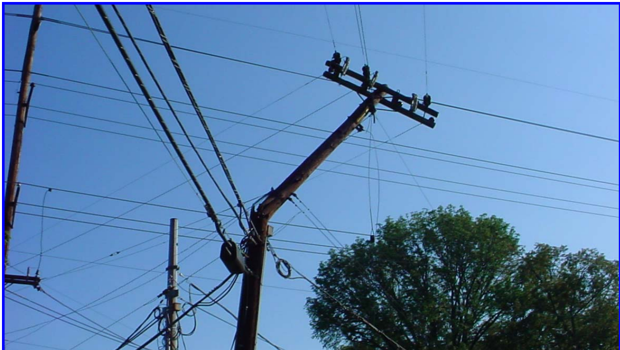
LG&E pole that snapped during 2008 wind storm. Note joint-use attachment just below break.
