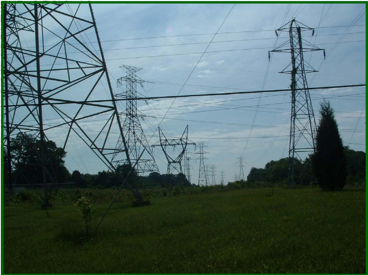
Transmission lines showing cleared right-of-way
