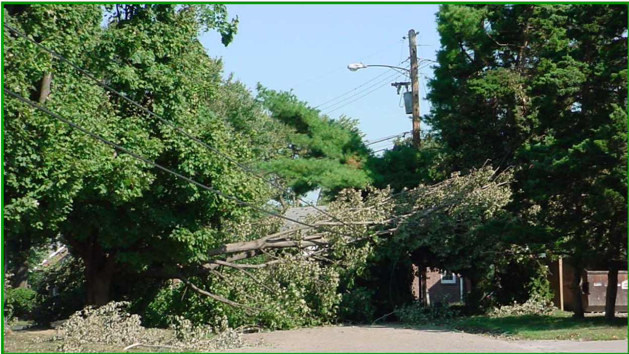
Typical damage in Louisville following the Sept. 14, 2008, wind storm. Fallen trees and limbs were the main cause of downed lines.
