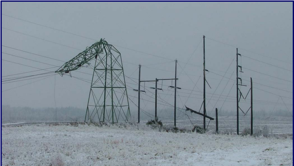
The weight of the ice, combined with strong winds, was enough to topple both metal and wooden transmission line structures in western Kentucky.
