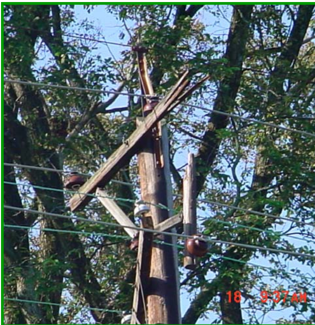
Broken crossarms on LG&E pole in Louisville After 2008 wind storm
