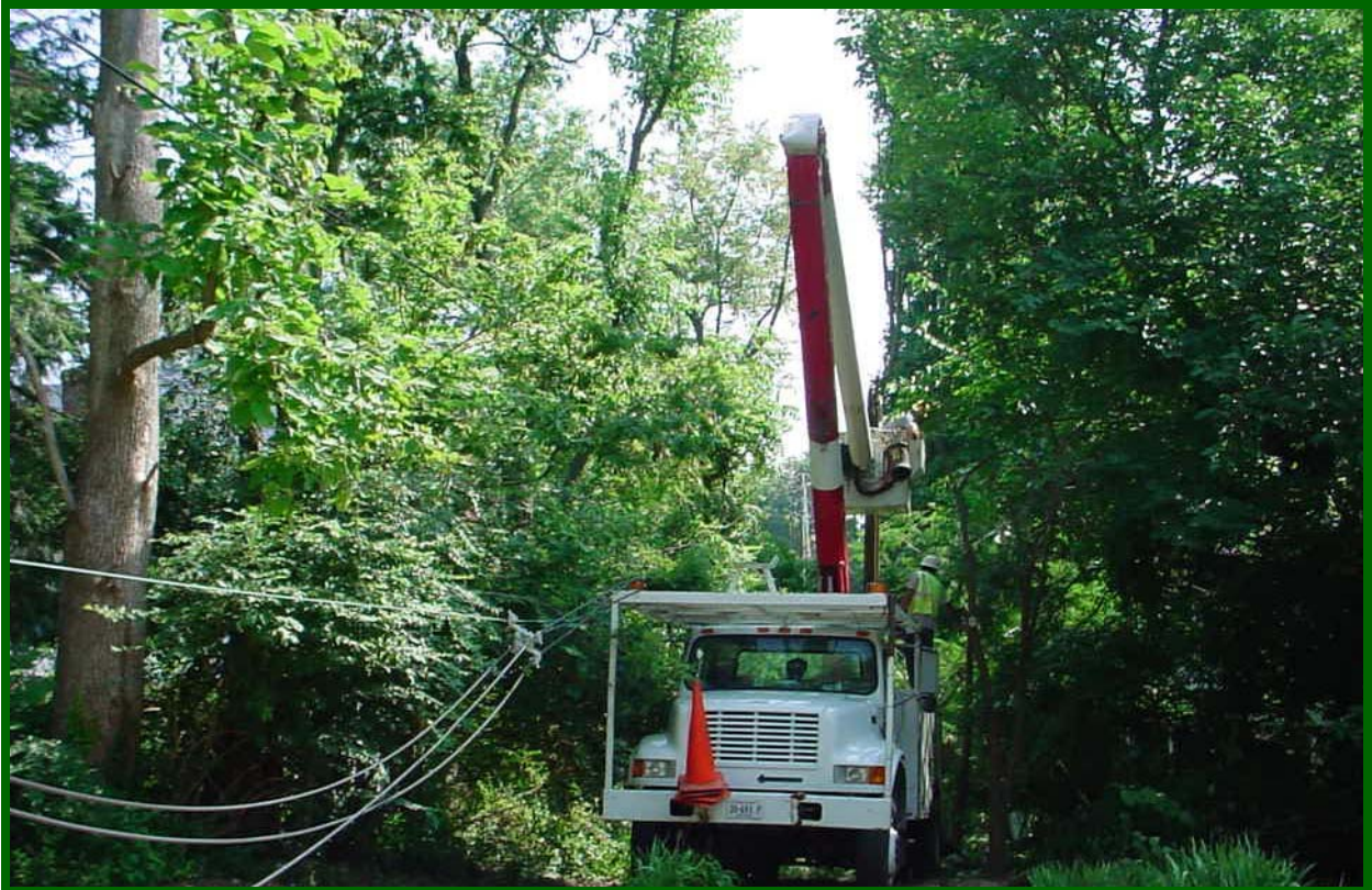
Restoration work in Jefferson County following a 2004 storm illustrates the difficulty of maintaining and restoring power in suburban areas with restrictions on vegetation management.
