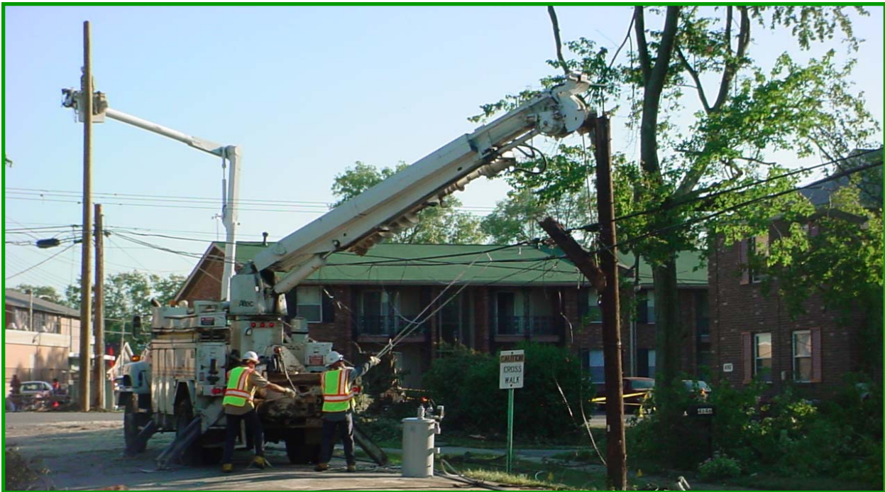
A crew from Allegheny Power works to replace a broken pole and transformer in western Louisville on Sept. 18, 2008.
