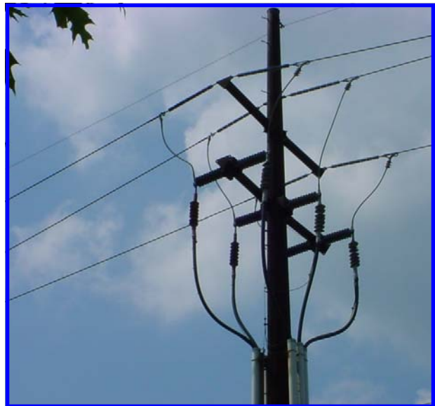
Connection from overhead lines to underground distribution system
