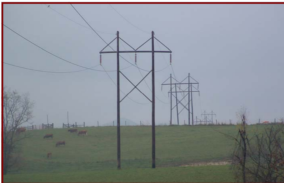
Typical wooden transmission structure
