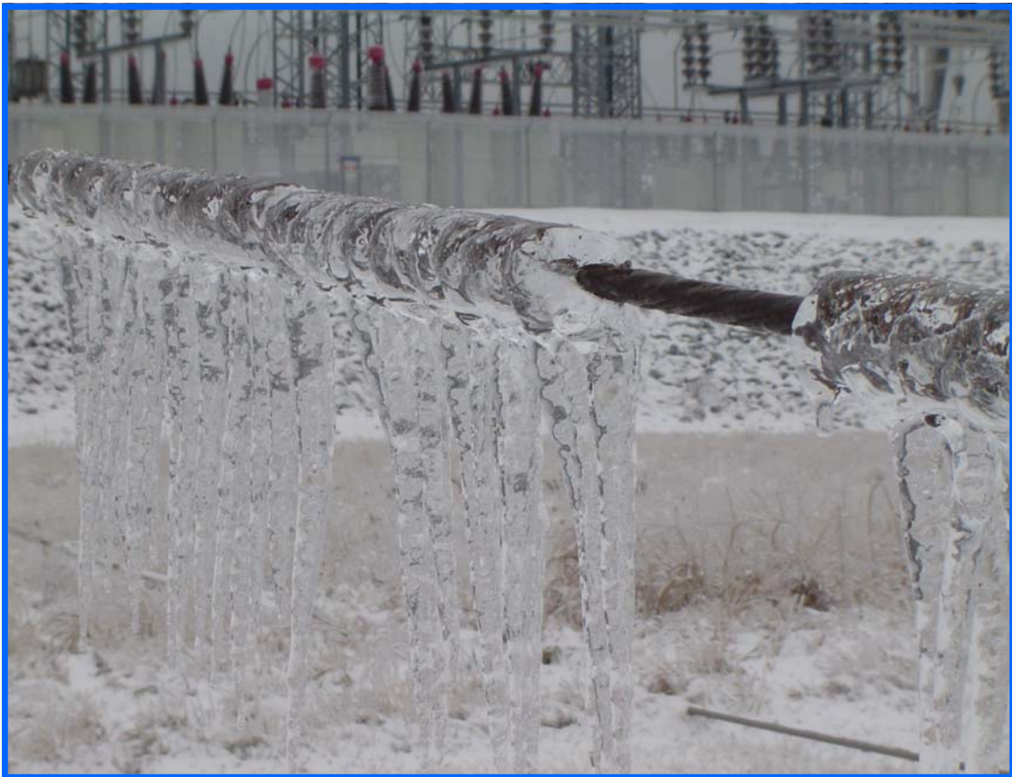
Heavy ice accumulation at Big Rivers Electric Corp.'s Barkley Lake Dam substation
