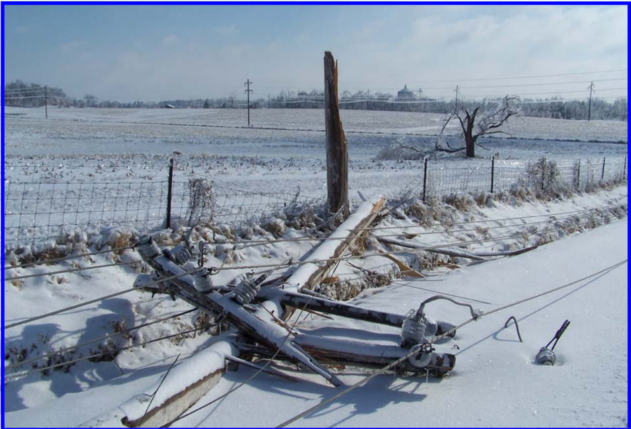
Damage to Jackson Purchase Energy distribution lines in 2009 ice storm
