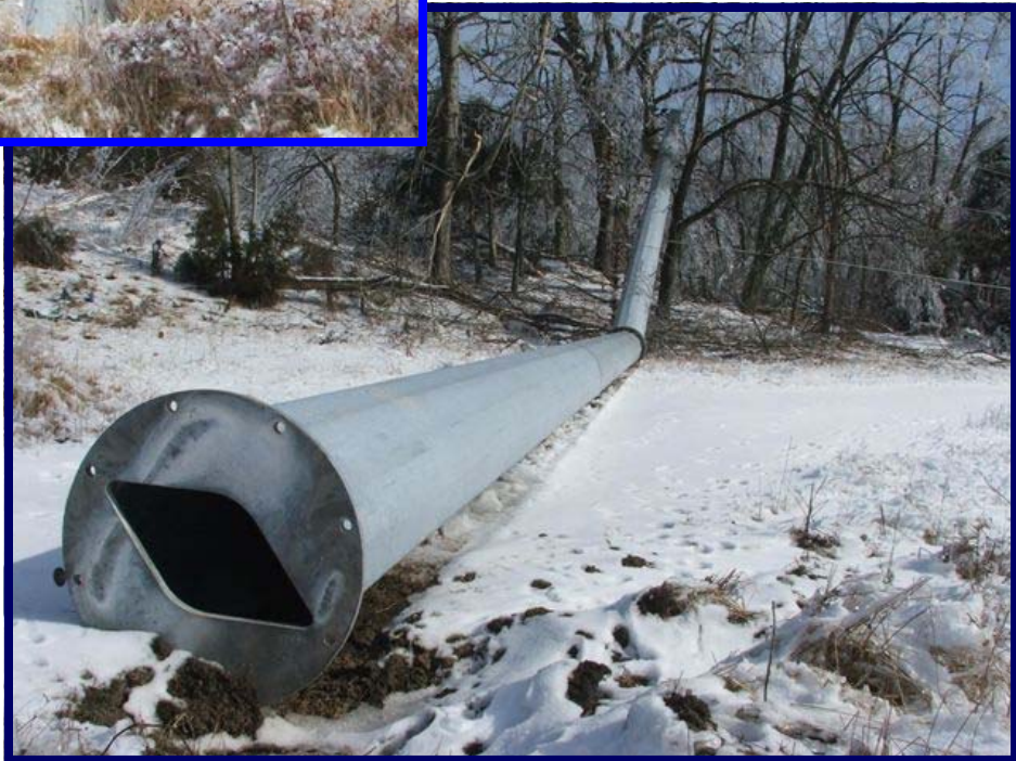
This 161-kV transmission line came down when the weight of ice combined with high winds to shear the bolts holding the middle section to the base.
