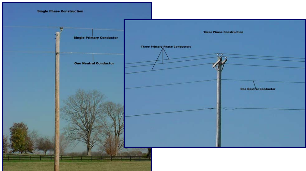
Figure 16: Single-phase and three-phase construction
