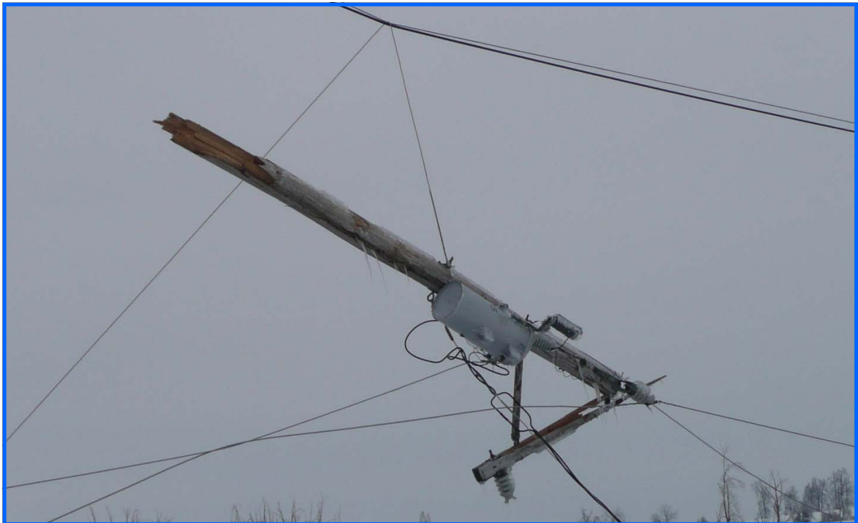
Kenergy pole with multiple failure points during 2009 ice storm
