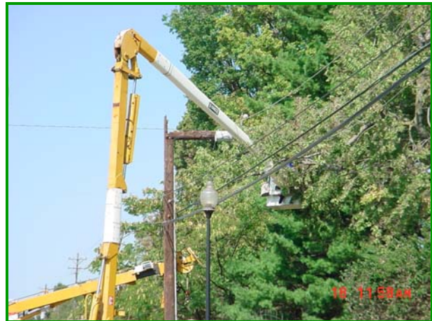
Repairing a broken distribution system pole in Louisville.
