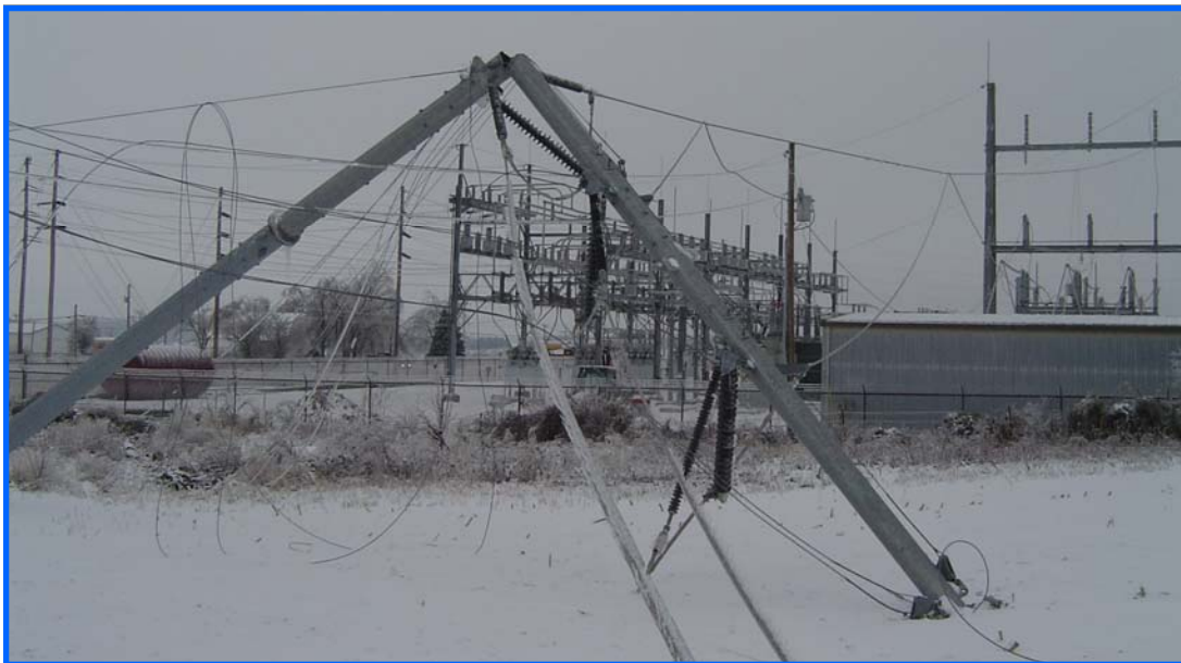
Big Rivers Electric Meade County substation after 2009 ice storm
