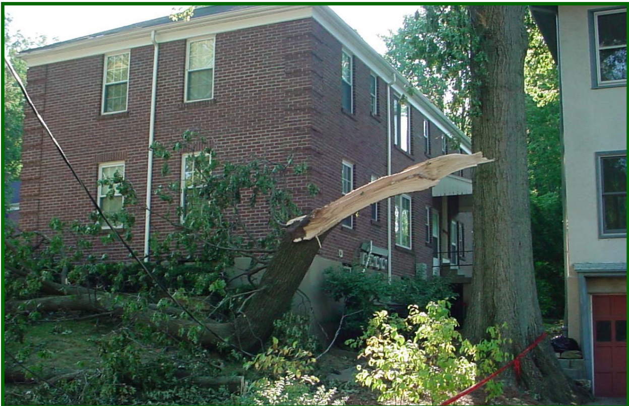
Outside service entrances are vulnerable to damage from falling limbs and trees
