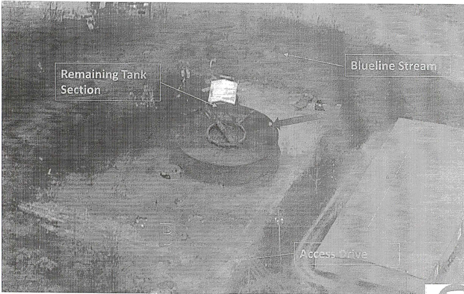
Exhibit "A" – Hunters Hollow WWTP (looking East)
