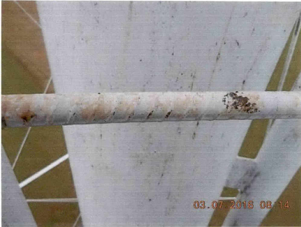
Same ladder rung
