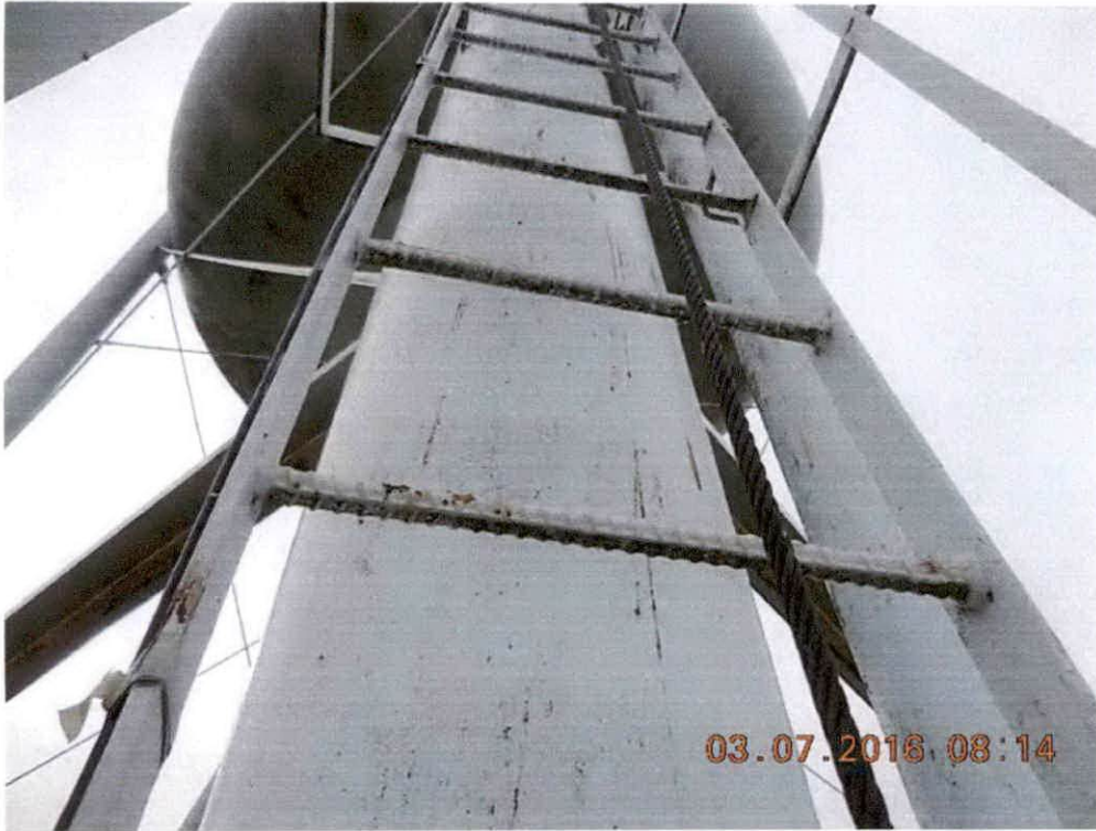
Backs of ladder rungs not painted, large amount of bird feces on leg
