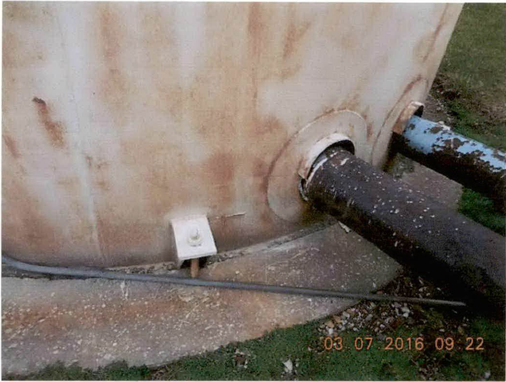
Foundation and piping
