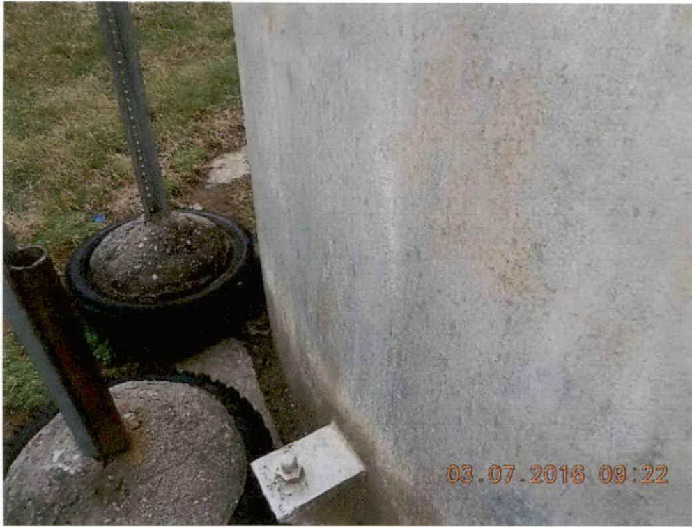
Tank sidewall to foundation
