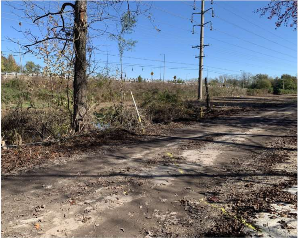
Permanent locate marker behind location of damage.
