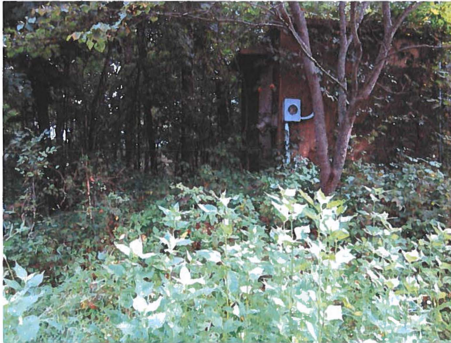
Looking North from Proposed Site at old equipment shelter
