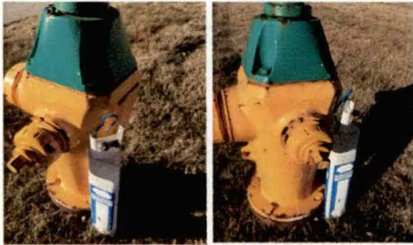
Trace wire installations gone bad
