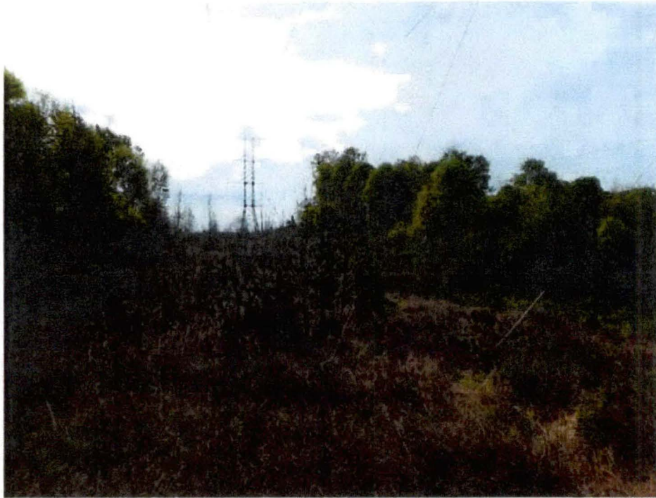
Looking south down the existing utility corridor and existing electrical transmission tower
