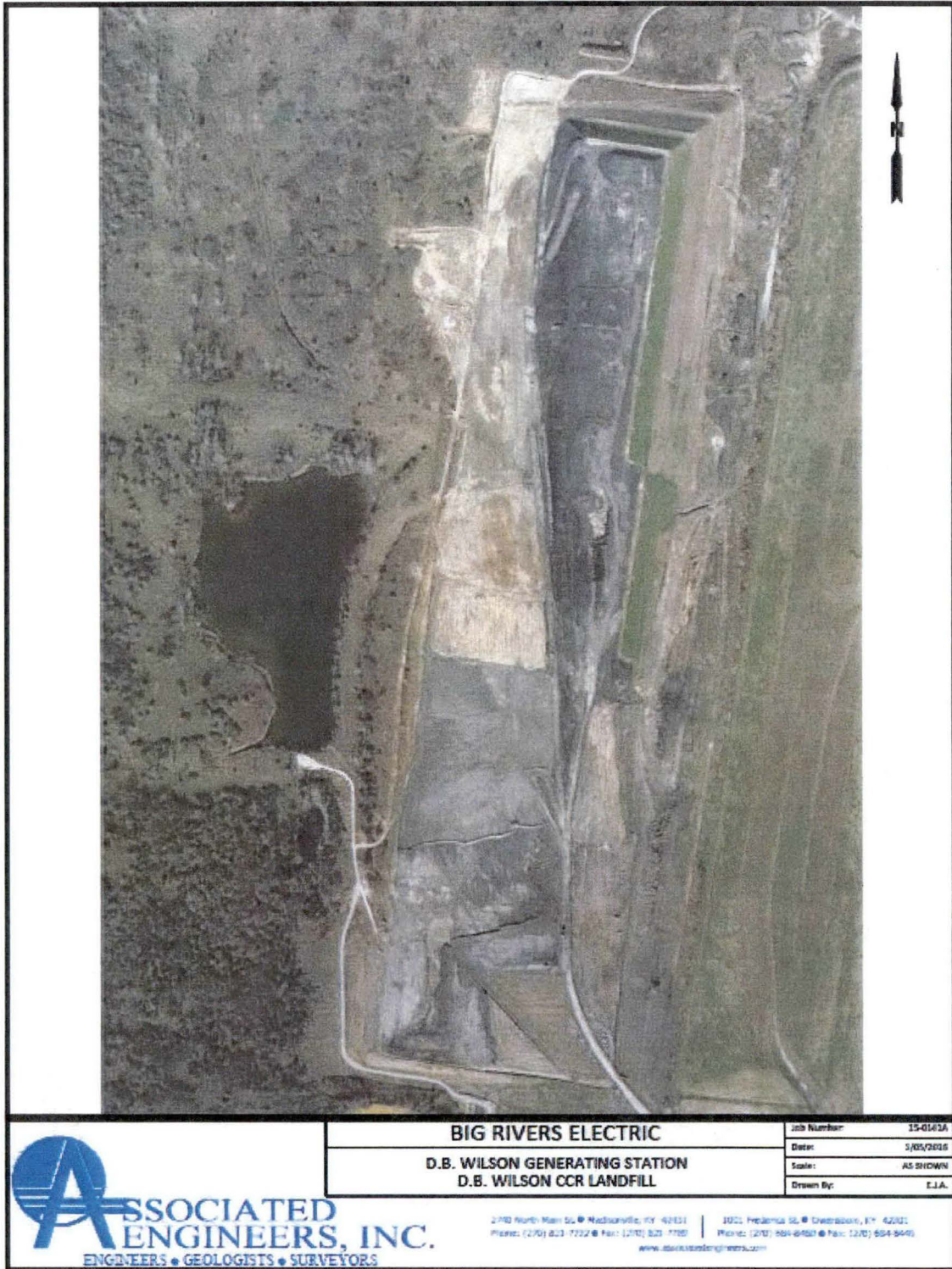
Attachment A. Aerial Photo of the D.B. Wilson CCR Landfill
