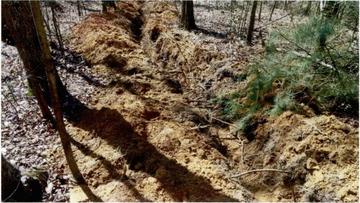
Trench At Site
