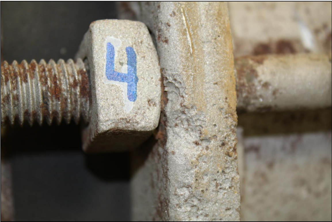
Figure 11. Image of the Bolt A4 fastener assembly which exhibited corrosion and pitting.
