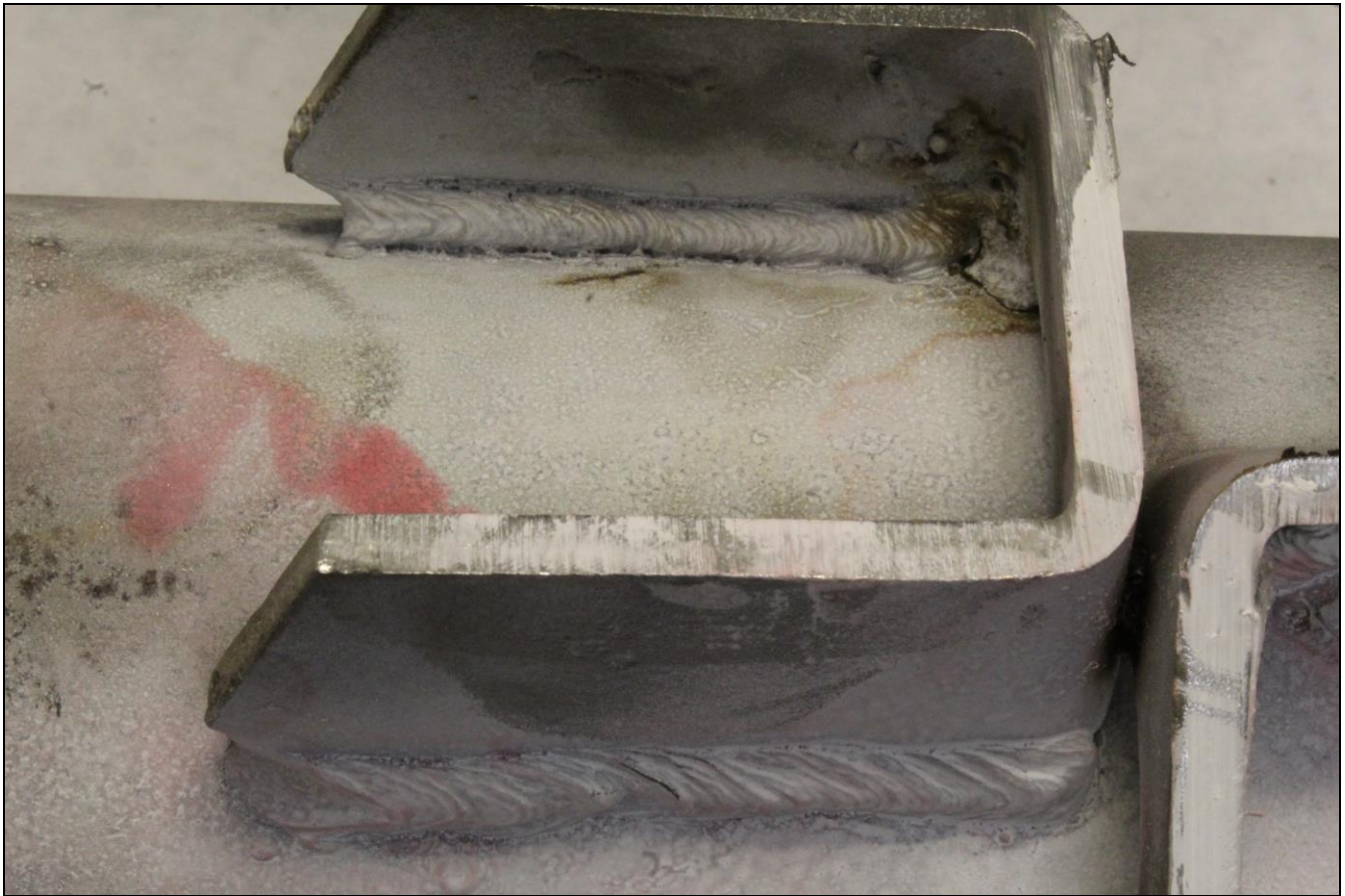
Figure 8. Image of the Lug A2 exterior top welds after dye penetrant media had been used during inspection.
