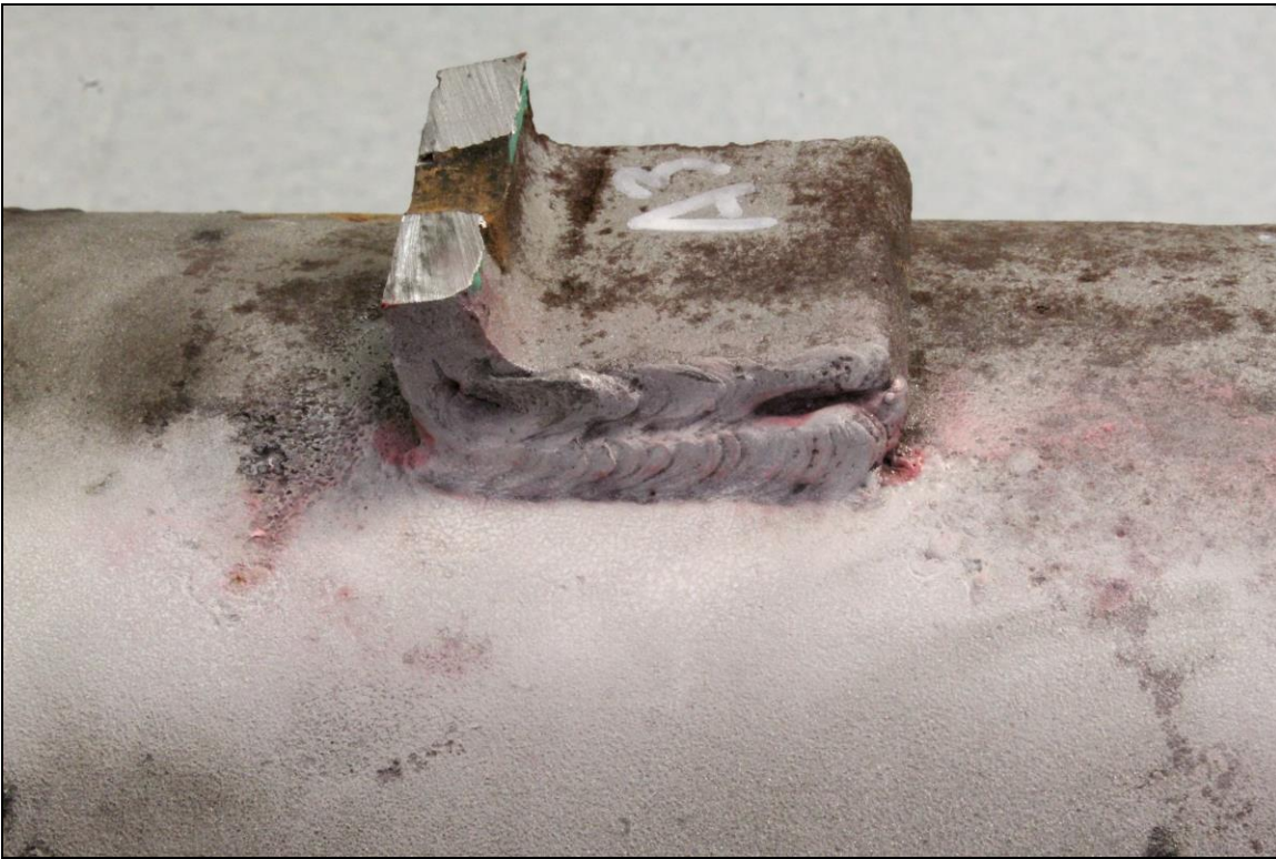
Figure 14. Image of the Lug A3 exterior top welds after dye penetrant media had been used during inspection.
