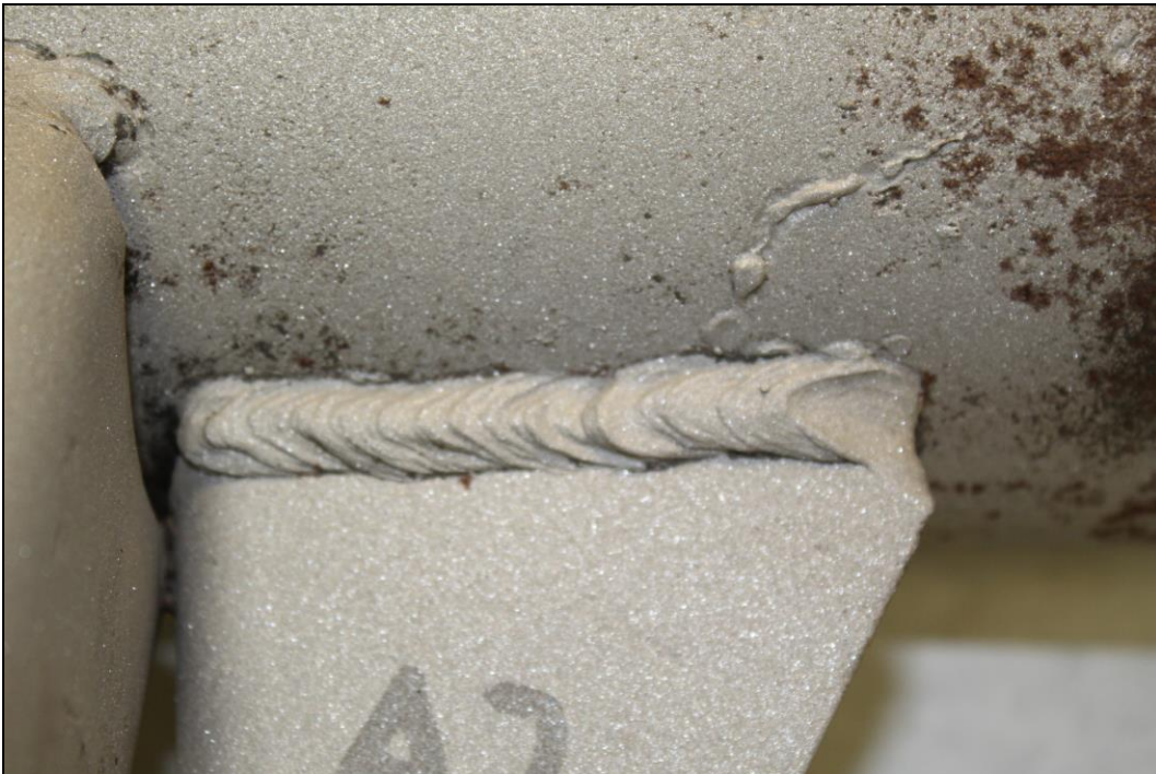
Figure 6. Image of the Lug A2 exterior top weld which exhibited substantial fusion except for some arc burn, and undercut.
