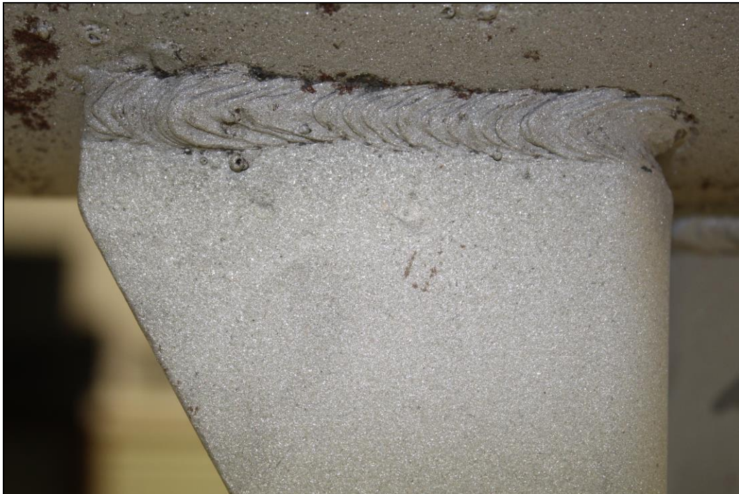
Figure 7. Image of the Lug B2 exterior top weld which exhibited substantial fusion except for some arc burn, spatter, porosity and undercut.
