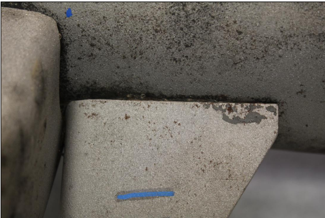
Figure 5. Image of the Lug A1 exterior bottom weld which exhibited no fusion.
