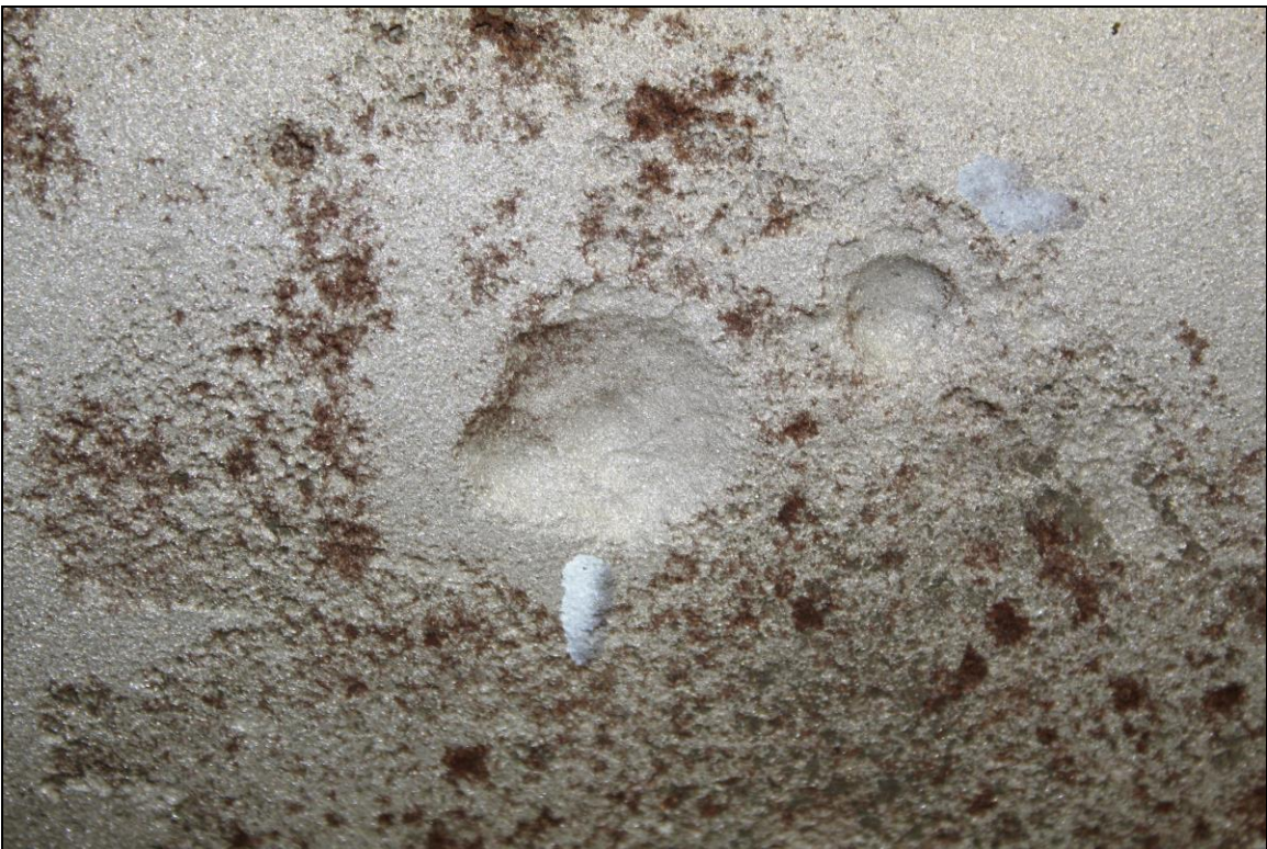
Figure 12. Image of the pipe exterior wall surface which exhibited substantial pitting damage.
