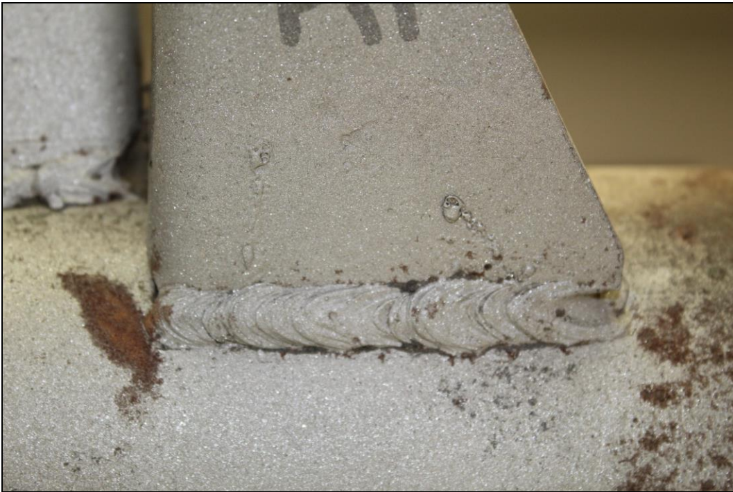
Figure 4. Image of the Lug A1 exterior top weld which exhibited substantial fusion except for some arc burn, porosity, undercut, and spatter.
