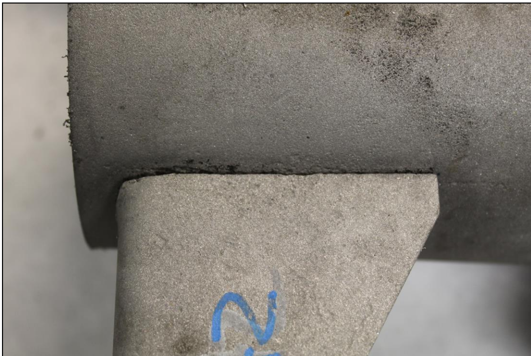
Figure 6. Image of the Lug A2 exterior bottom weld which exhibited no fusion.
