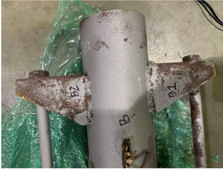
Figure 5 Lugs Pipe B
