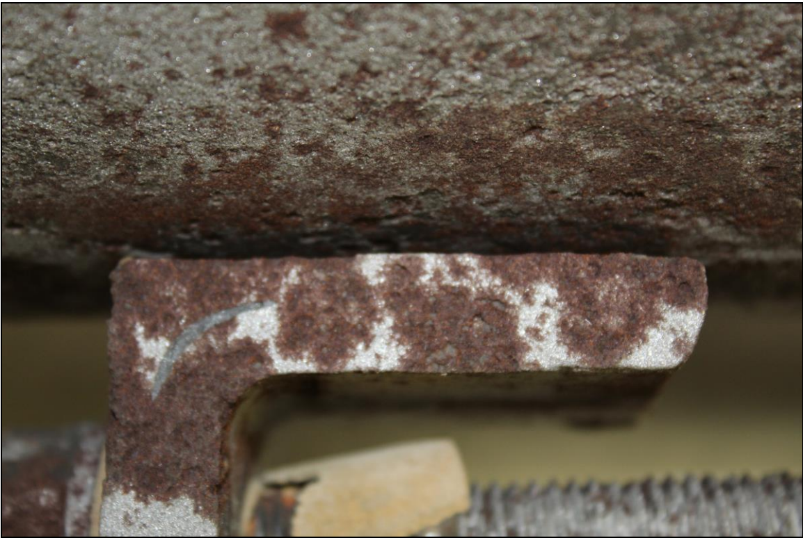
Figure 7. Image of the Lug A5 exterior bottom weld which exhibited no fusion.
