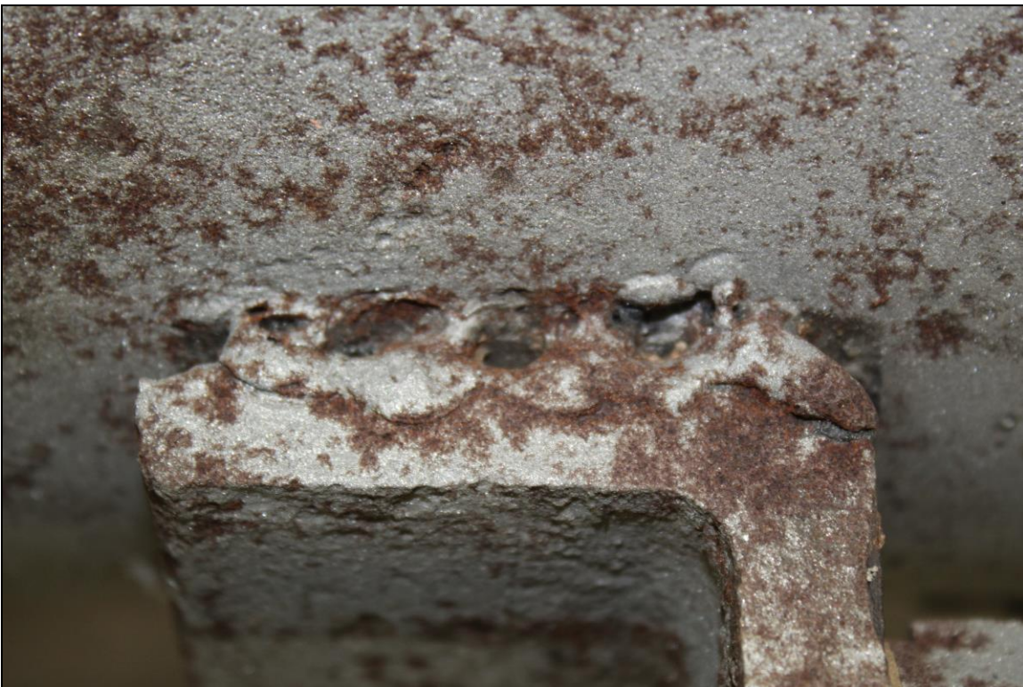
Figure 10. Image of the Lug B5 exterior bottom weld which exhibited minimal fusion.
