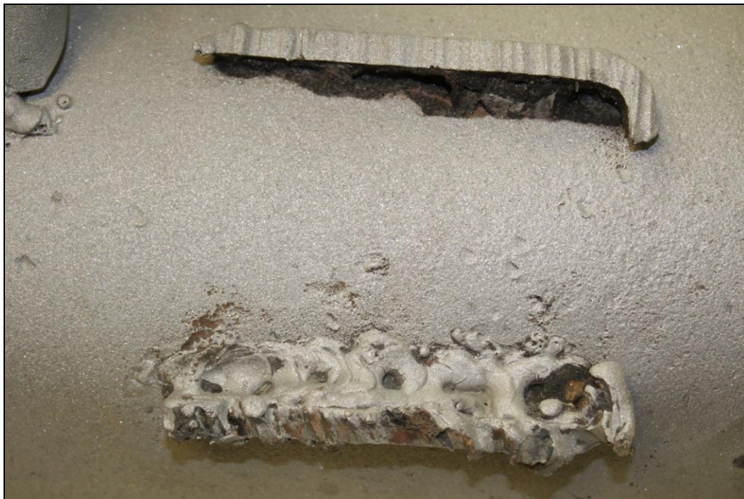
Figure 10. Image of the remainders of additional lugs, which had been welded then cut off, present on Side A of the assembly.
