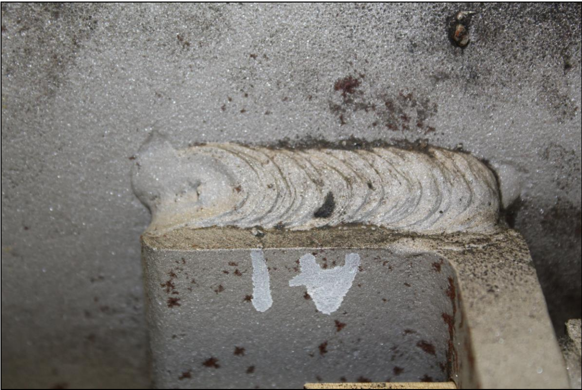
Figure 5. Image of the Lug A1 exterior top weld which exhibited substantial fusion except for some arc burn and undercut.
