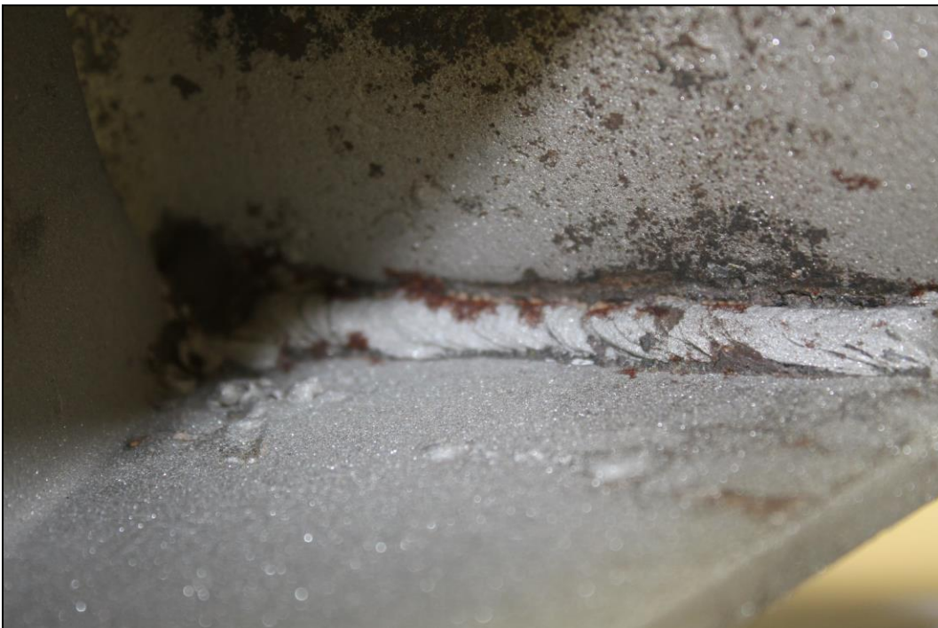
Figure 7. Image of the Lug A2 interior bottom weld which exhibited substantial fusion except for some arc burn and spatter.
