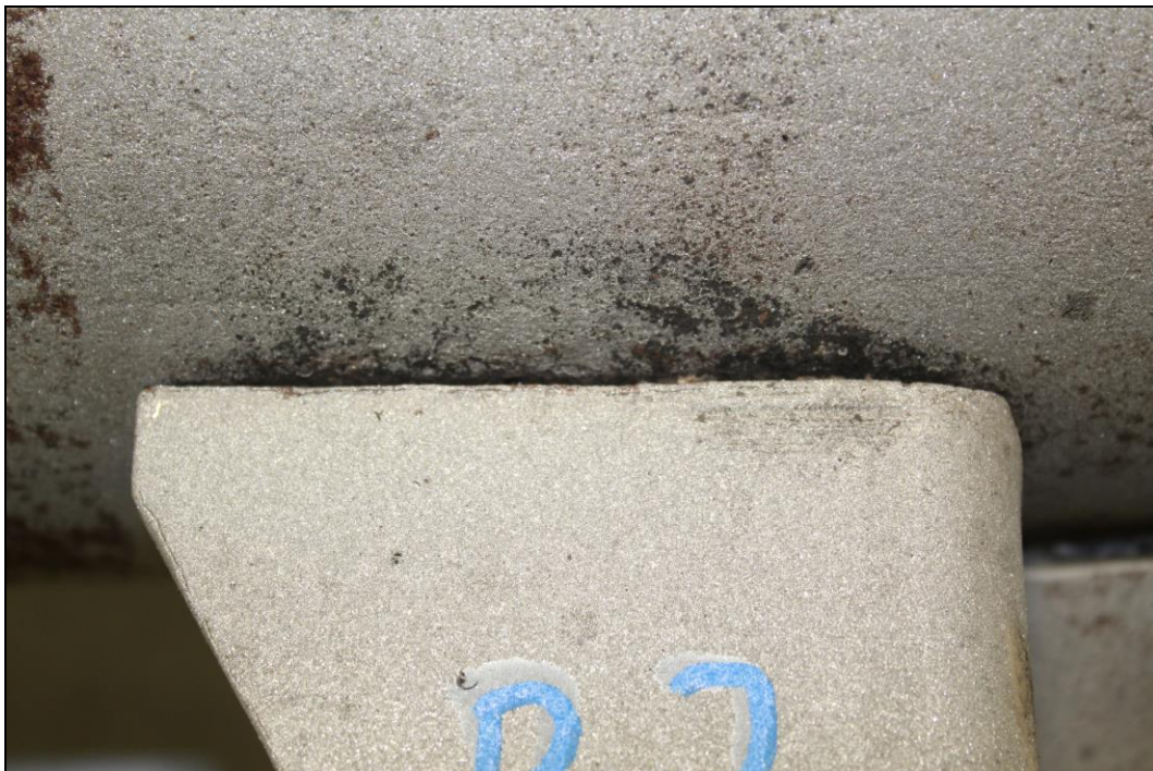
Figure 8. Image of the Lug B2 exterior top weld which exhibited no fusion.
