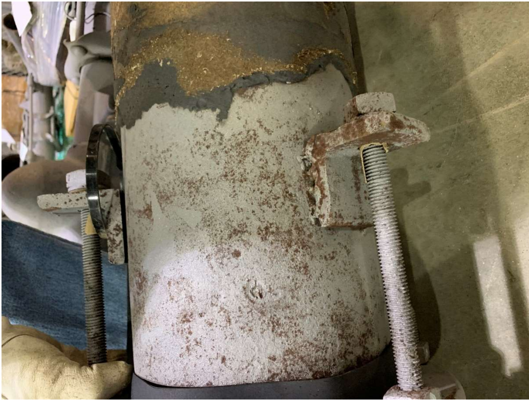
Figure 7 Pipe B, Lug B2 and B3
