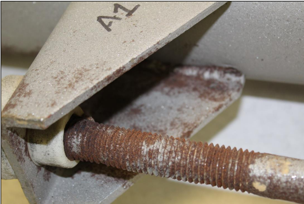
Figure 9. Image of the Lug A1 fastener assembly which exhibited substantial corrosion.
