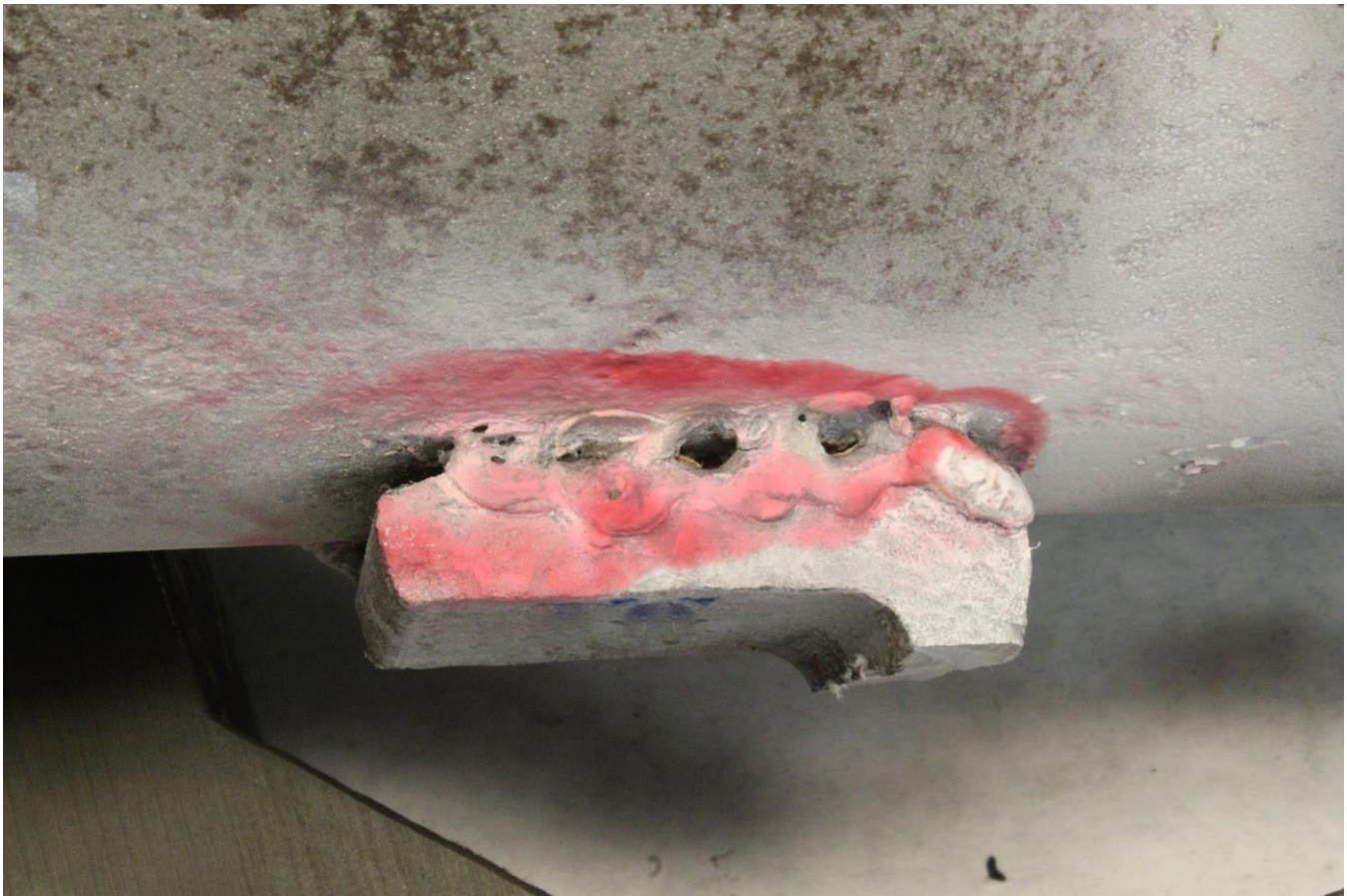
Figure 13. Image of the Lug B5 exterior bottom welds after dye penetrant media had been used during inspection.
