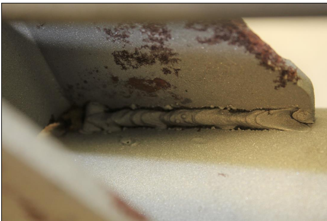
Figure 8. Image of the Lug B2 interior bottom weld which exhibited substantial fusion except for some arc burn, spatter, porosity and undercut.
