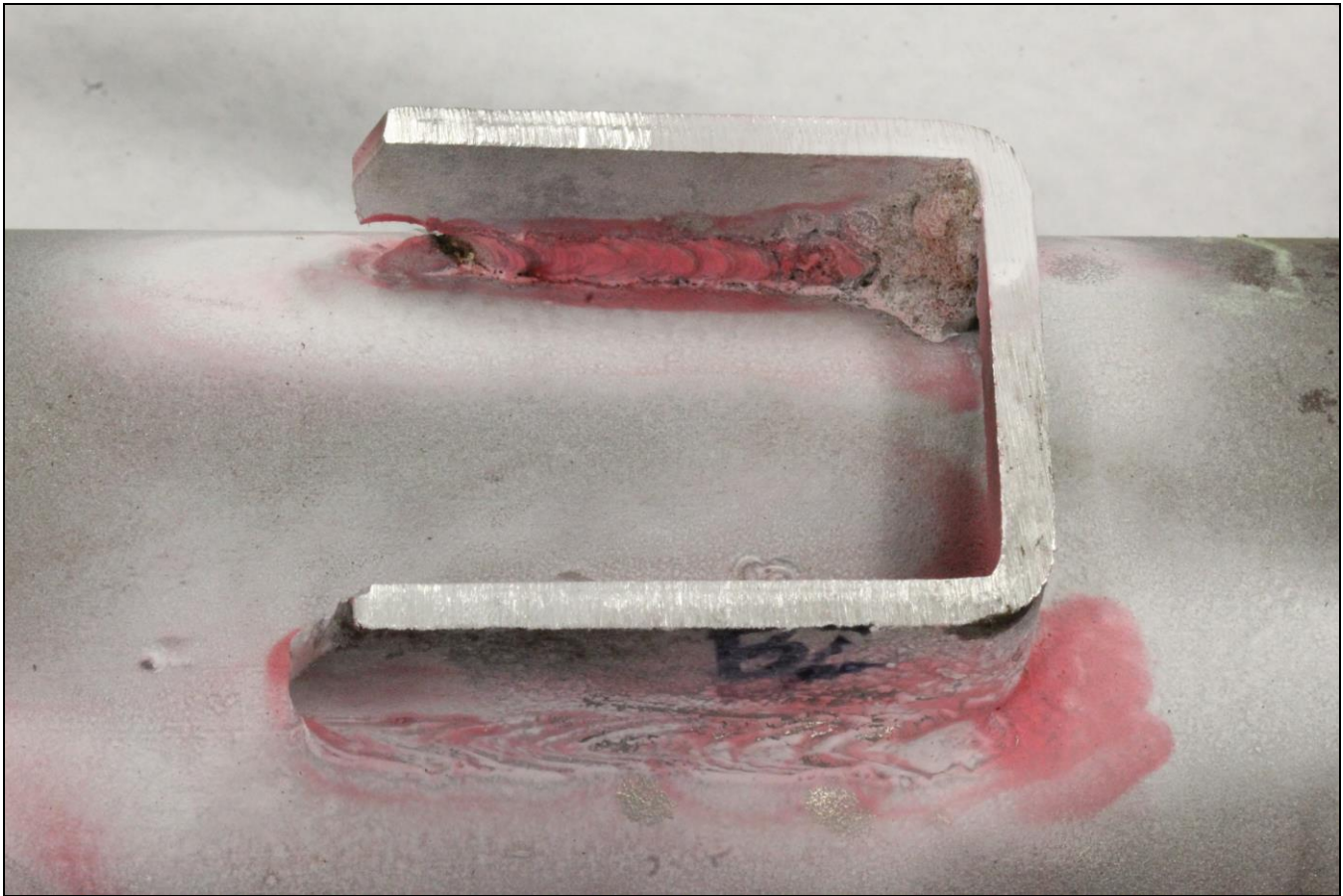
Figure 12. Image of the Lug B2 welds after dye penetrant media had been used during inspection.
