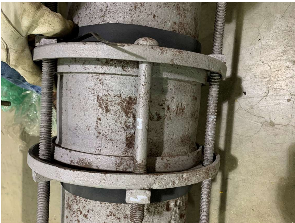
Figure 2 Coupler Body
