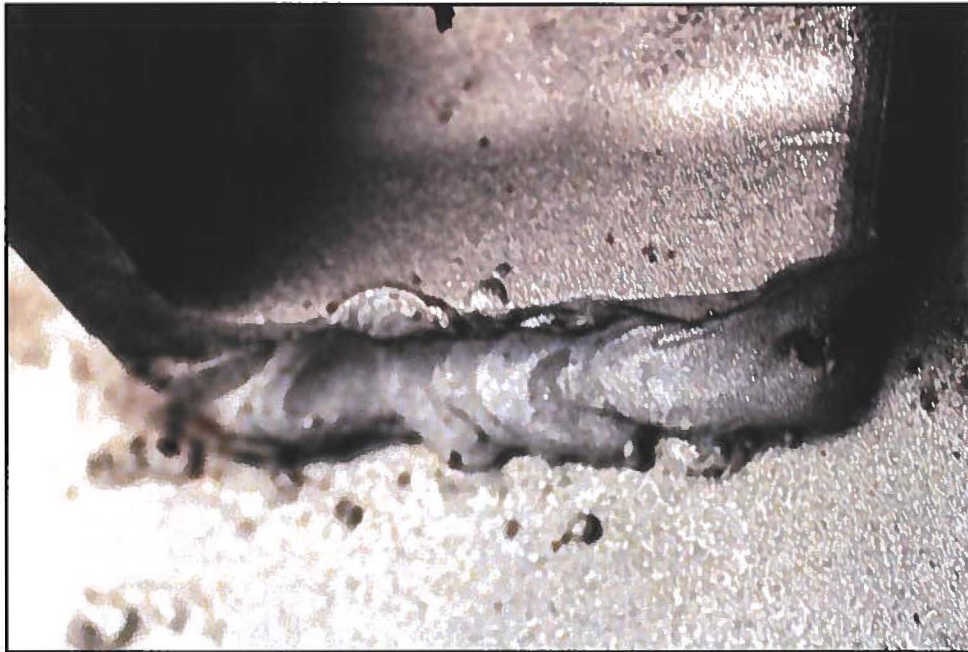
Figure 10. Image of the Lug B6 exterior bottom weld which exhibited substantial fusion except for some arc burn, porosity, spatter and undercut.
