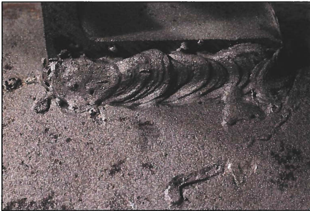
Figure 5. Image of the Lug A4 exterior bottom weld which exhibited substantial fusion except for some arc burn, porosity and spatter.
