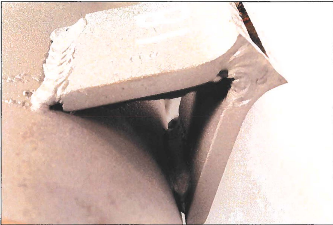
Figure 9. Image of the Lug B1 exterior top and interior bottom welds.
