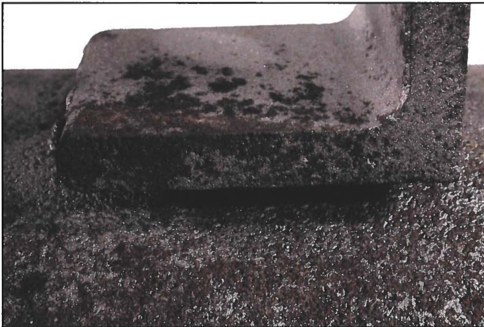
Figure 6. Image of the Lug A4 exterior top weld which exhibited no fusion.
