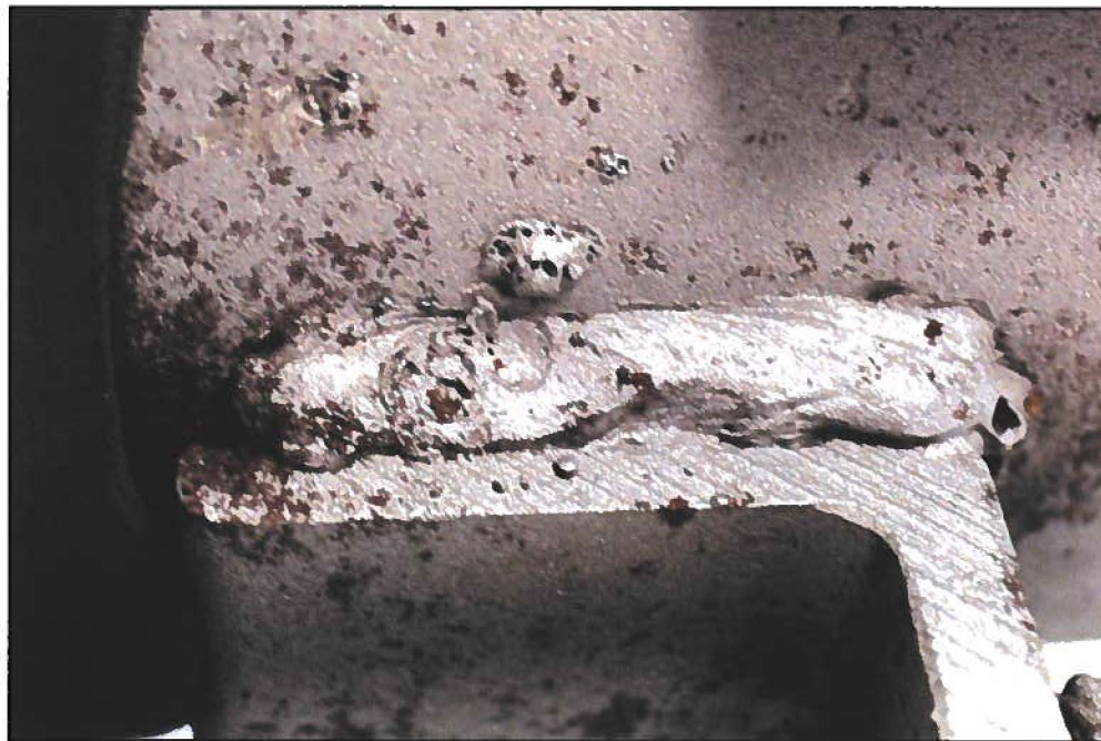
Figure 8. Image of the Lug B2 exterior bottom weld which exhibited substantial fusion except for some arc burn, spatter, porosity and undercut.
