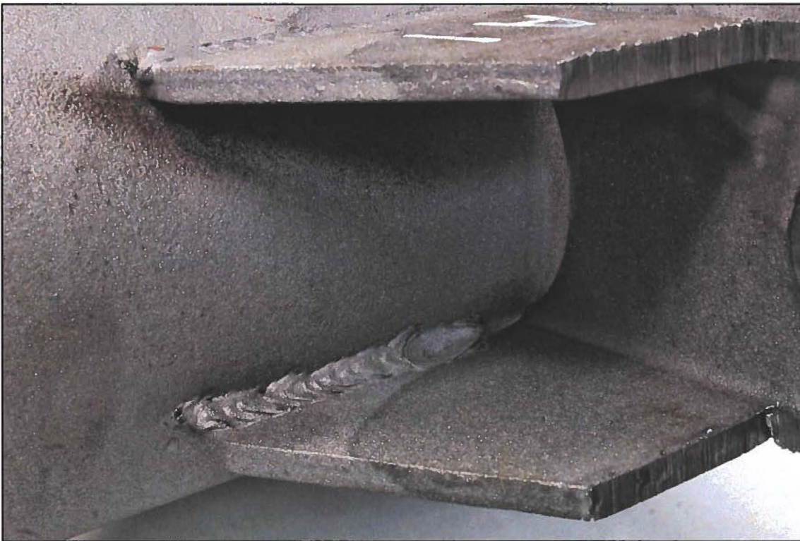
Figure 8. Image of the Lug A1 interior bottom weld.
