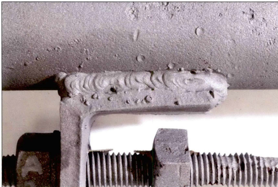
Figure 6. Image of the Lug A2 exterior top weld which exhibited substantial fusion except for some underfill, undercut and spatter.
