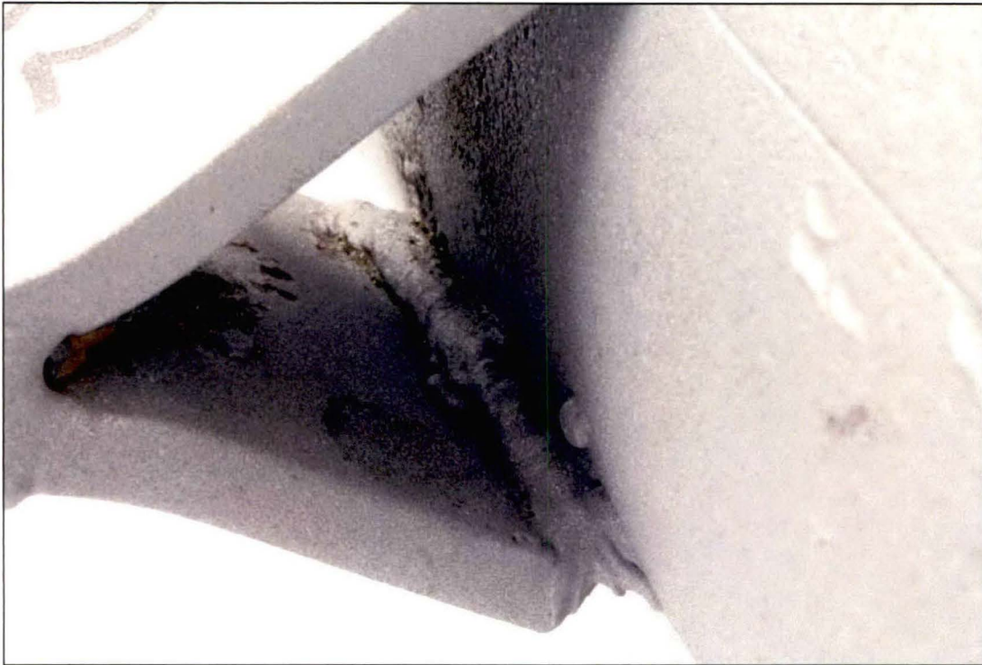
Figure 11. Image of the Lug A2 interior bottom weld which exhibited substantial fusion except for some overlap and spatter.
