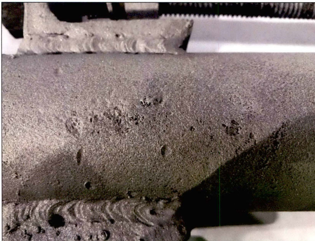
Figure 8- Corrosion Pipe A
