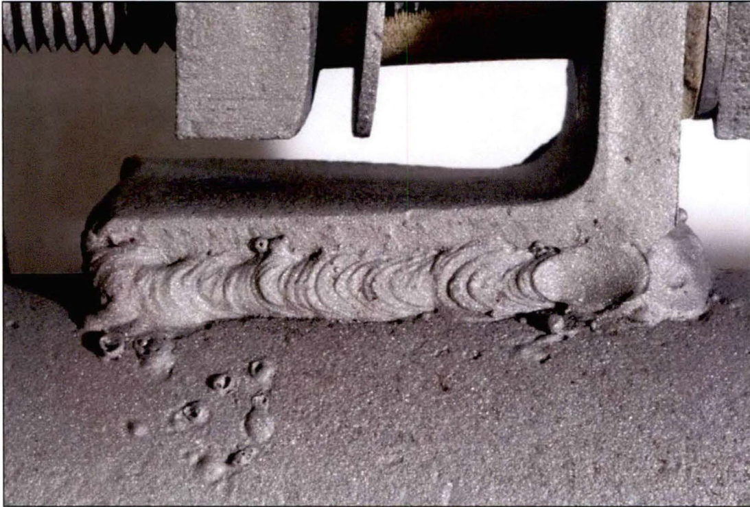
Figure 7. Image of the Lug B1 exterior top weld which exhibited substantial fusion except for some underfill, undercut and spatter.
