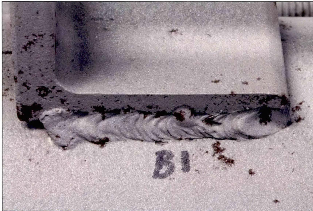
Figure 6. Image of the Lug B1 left weld which exhibited substantial fusion.
