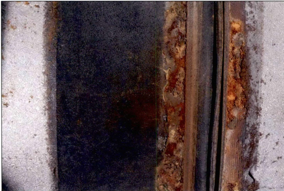
Figure 18. Image of the sleeve on the exterior of the pipe. Some debris was also present.
