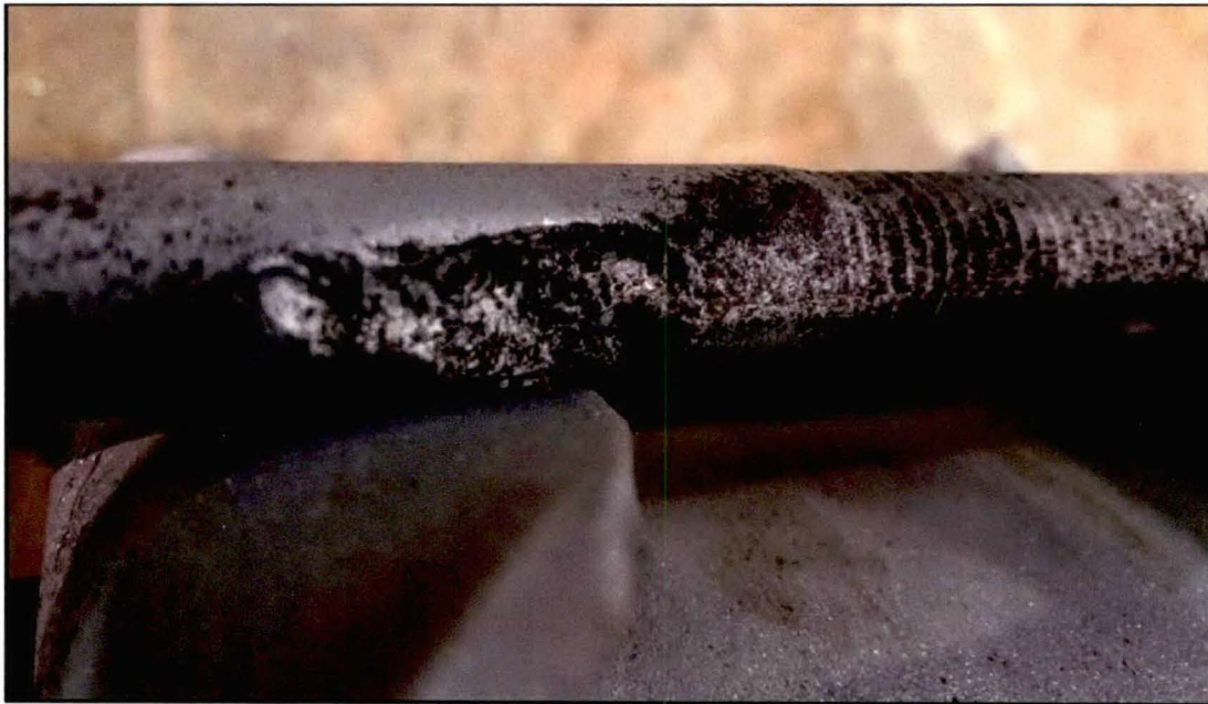
Figure 7- Rod 1 Metal Loss
