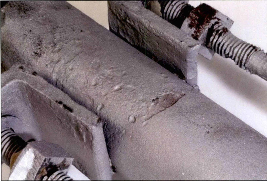
Figure 9. Image of the underside of Lugs A1 and A2 showing that no welding had been performed.
