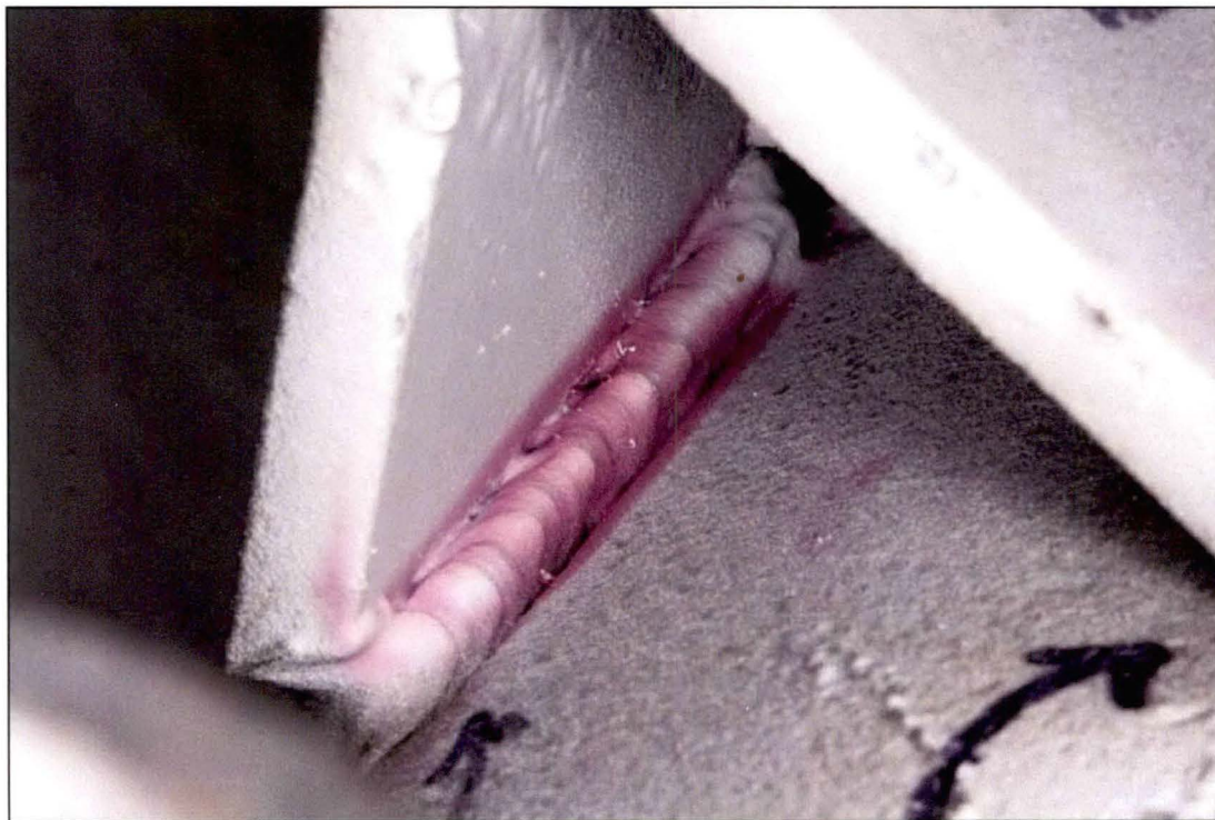
Figure 20. Image of the Lug B1 interior bottom weld after dye penetrant media had been used during inspection.
