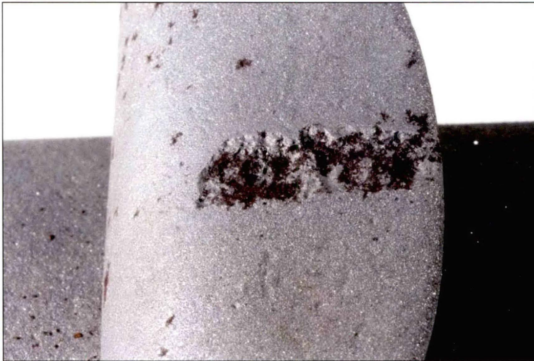
Figure 14. Photograph showing some superficial rust on the coupling surface where a rod had been in close proximity.
