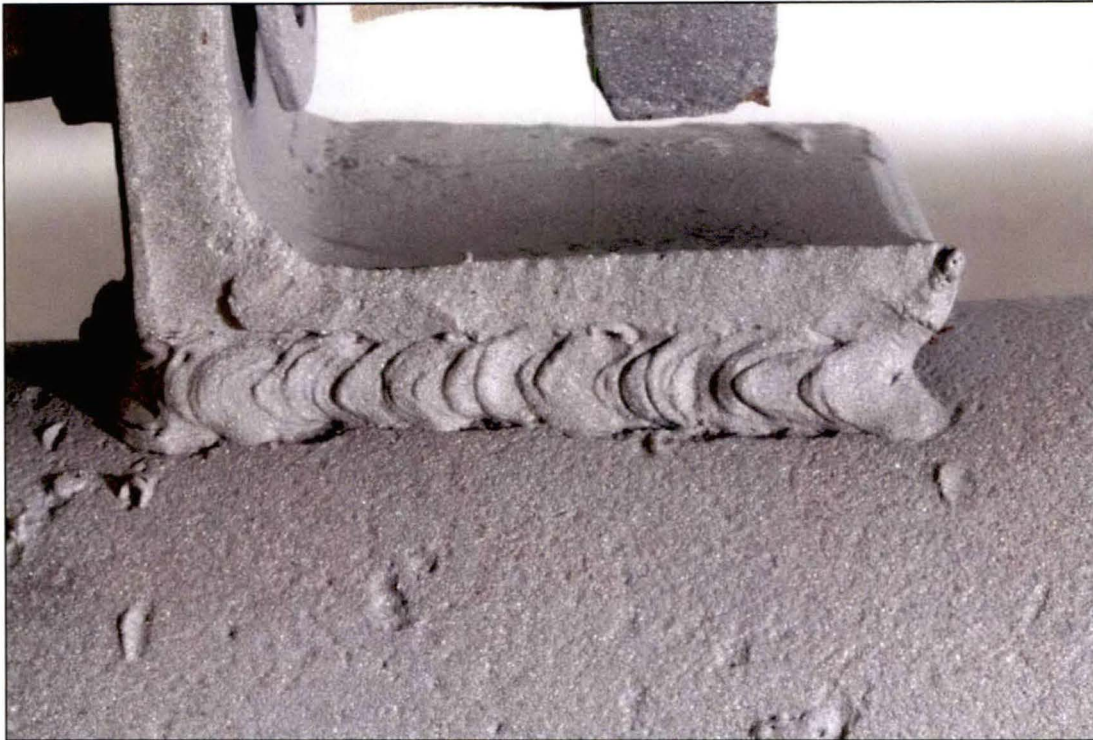
Figure 5. Image of the Lug A1 exterior top weld which exhibited substantial fusion except for some underfill, and undercut.
