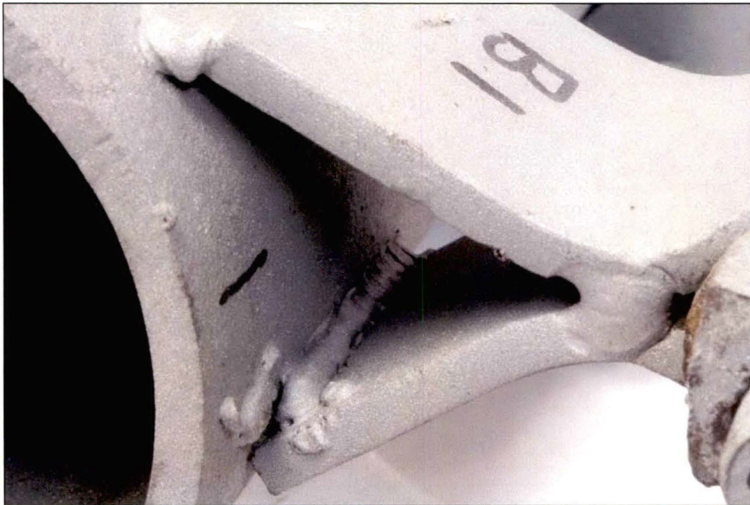
Figure 12. Image of the Lug B1 interior bottom weld which exhibited some fusion.
