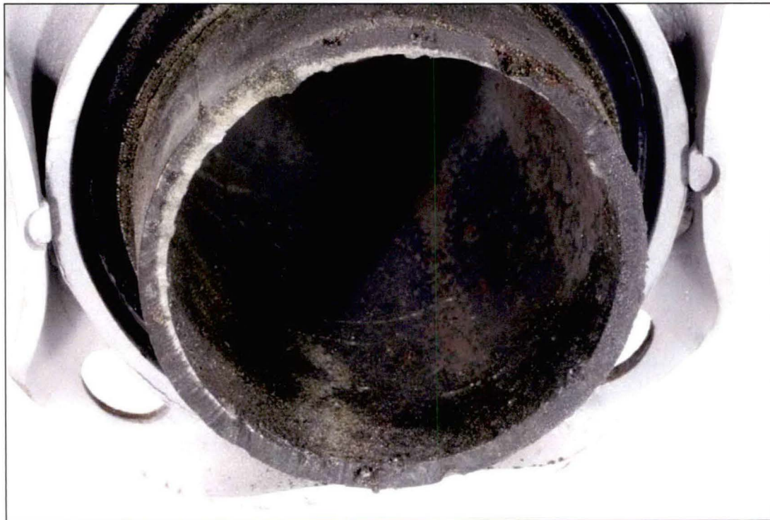
Figure 16. Photograph of the end of the End B pipe section.
