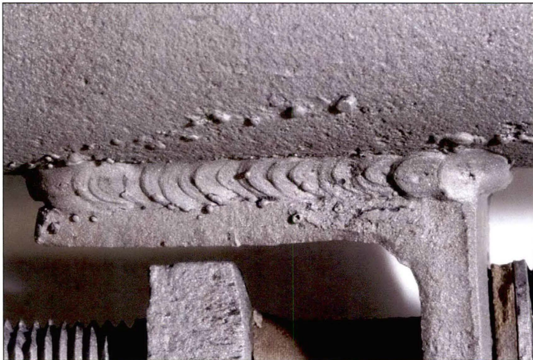
Figure 8. Image of the Lug B2 exterior top weld which exhibited substantial fusion except for some underfill, undercut and spatter.
