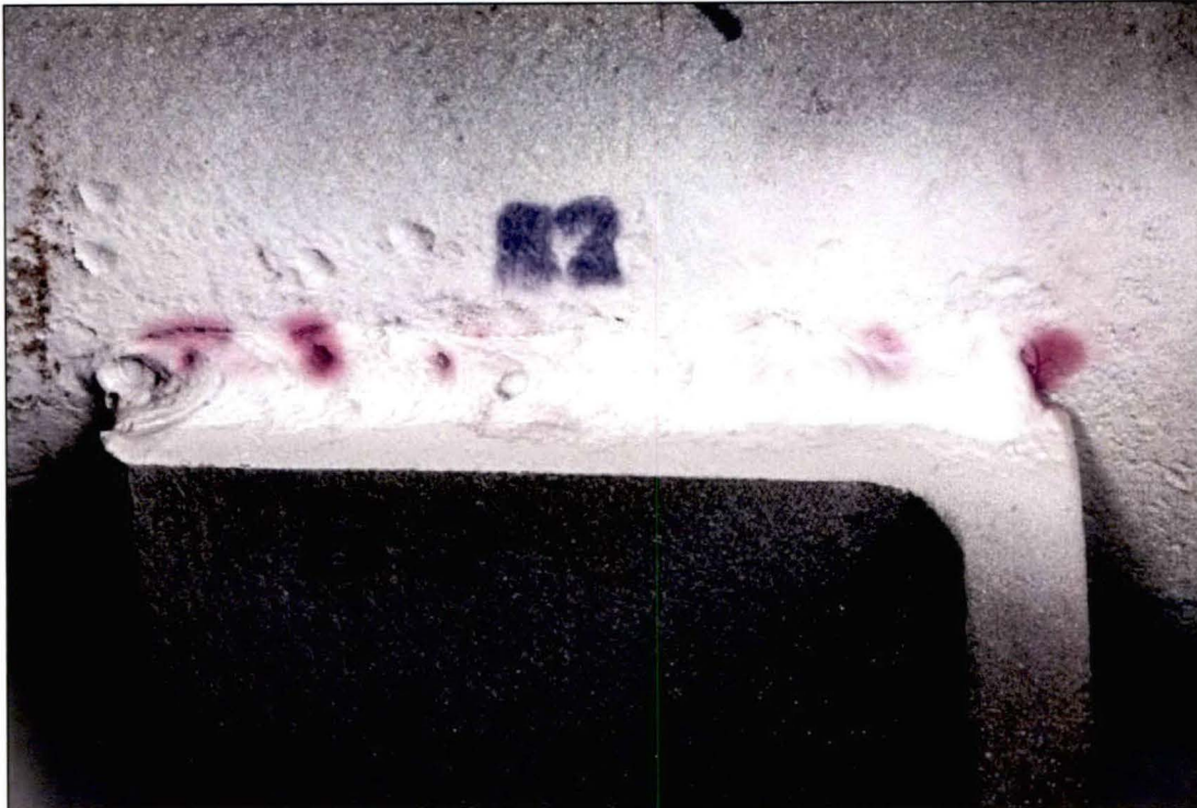
Figure 20. Image of the Lug B2 top weld which exhibited numerous pores.
