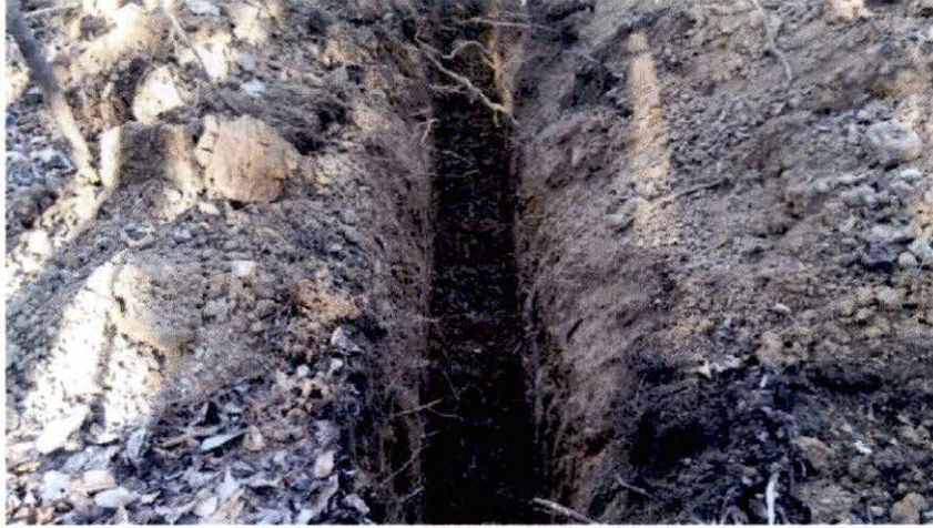
Trench At Site
