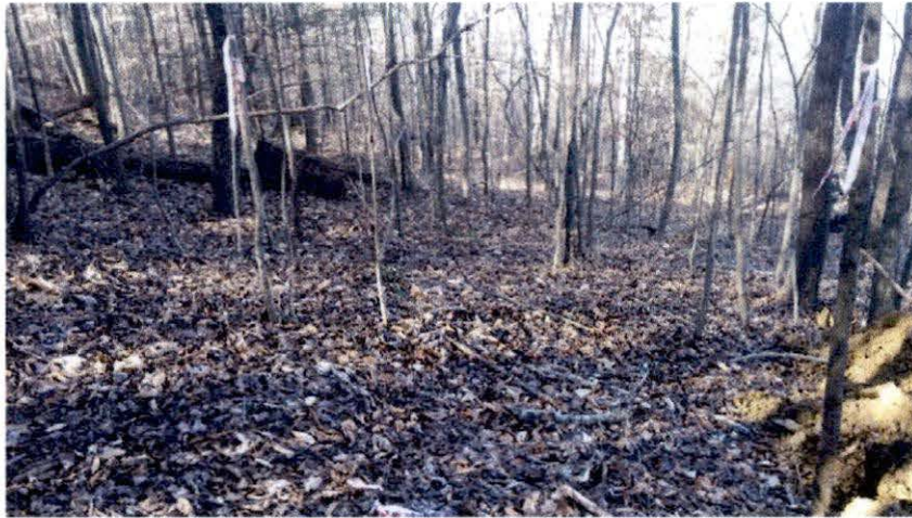
Site Before Trenching
