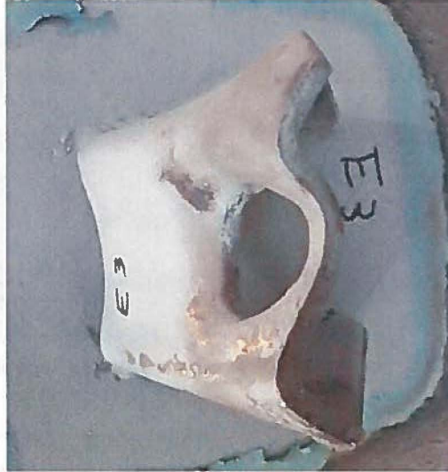
Figure 24. E side bracket #3 compression overload
