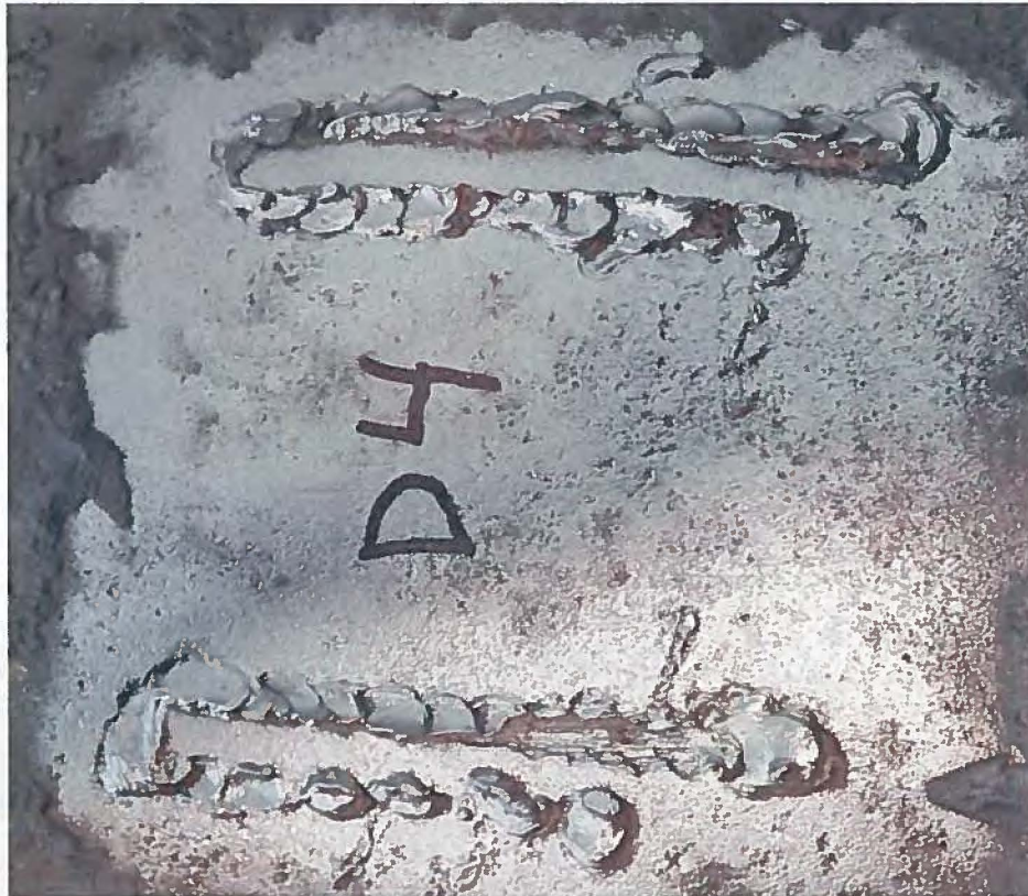
Figure 18. Pipe D bracket #4 weld bead on surface
