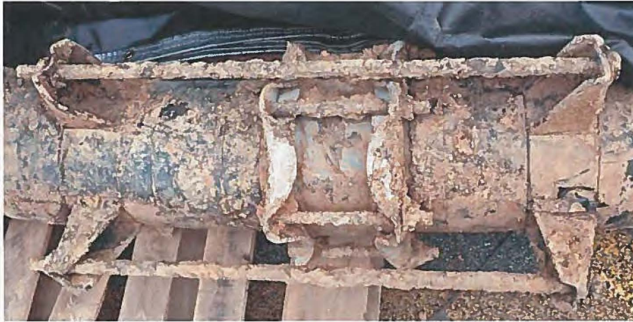
Figure 34. 8" coupling on pipe segment B-C
