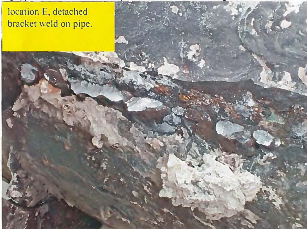
Figure 20. E side Bracket #4, close-up of weld fracture (Elder Park Side)
