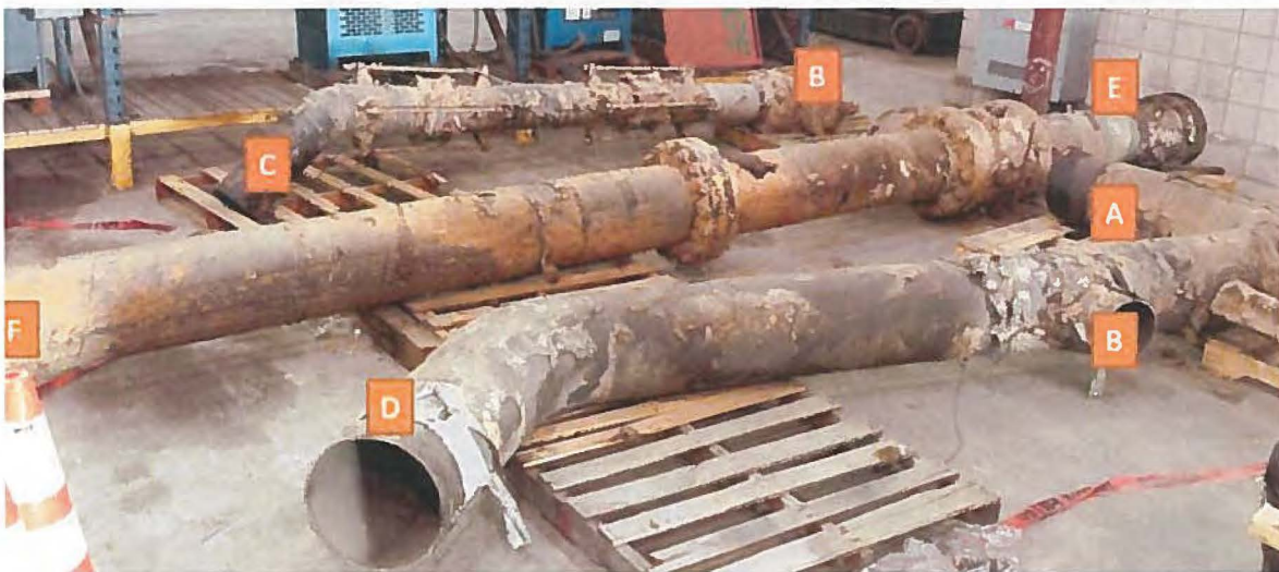
Figure 2. Pipes removed from Goshen Intersection as photographed by LG&E
