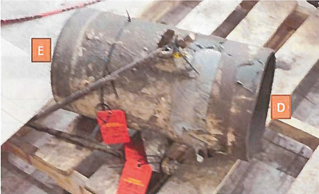
Figure 3. End segment D-E, pipe was cut by LG&E at D after incident
