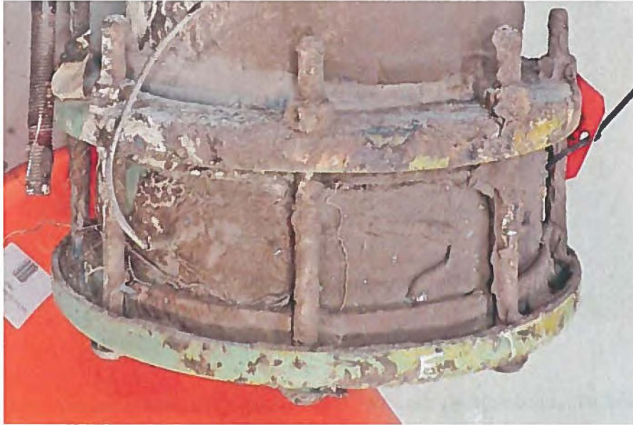
Figure 4. Failed 12" gas pipe coupling
