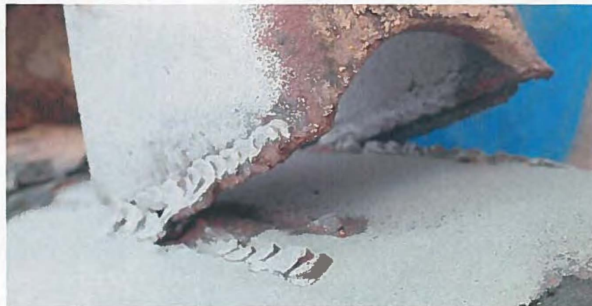
Figure 37. 8" pipe fractured weld bead after cleaning
