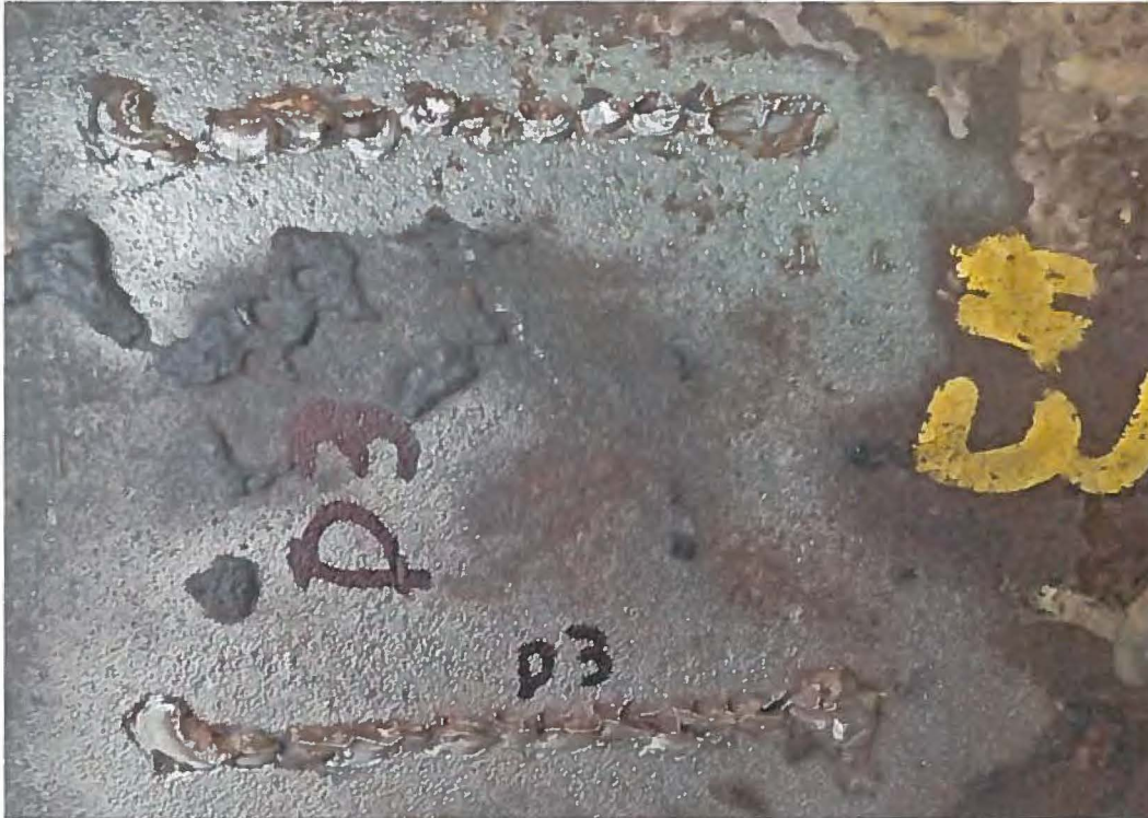
Figure 13 Weld beads for bracket #3 on pipe D surface after bead blasting
