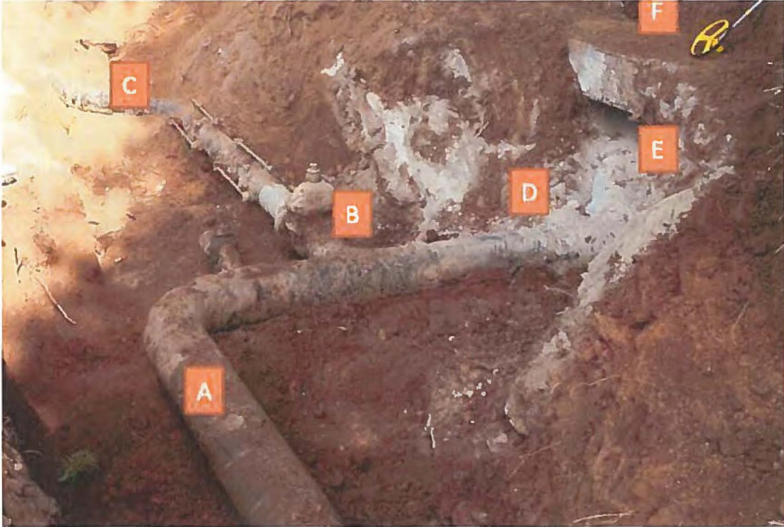
Figure 1. Highway 42 Goshen KY intersection excavation prior to pipe separation
