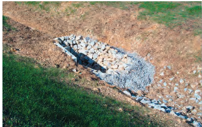
This is a good example of using smaller stone to face off ponding berm built of larger stone. The small rock ensures long ponding times, which maximizes sediment settling and removal.
