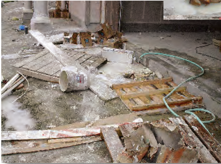
Polluted runoff from construction sites can result in fines up to $27,500 per day per violation. Stop work orders can cause construction delays of days, weeks, or even months.
