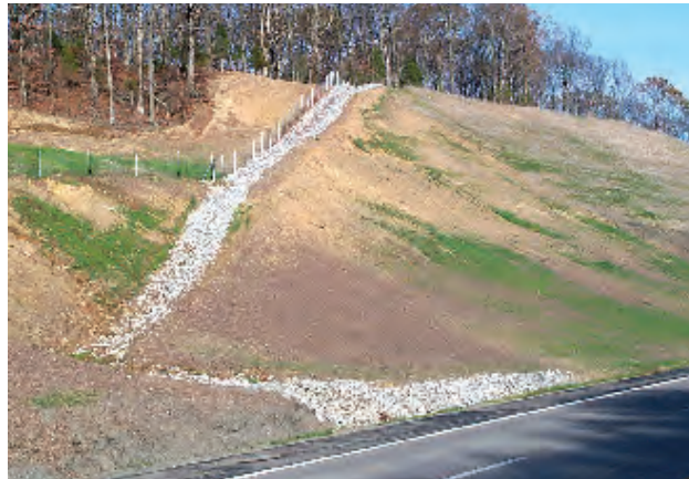
Stable diversion ditch protects slope during excavation and afterwards. Note spreader configuration of ditch discharge point, which helps dissipate flows.
