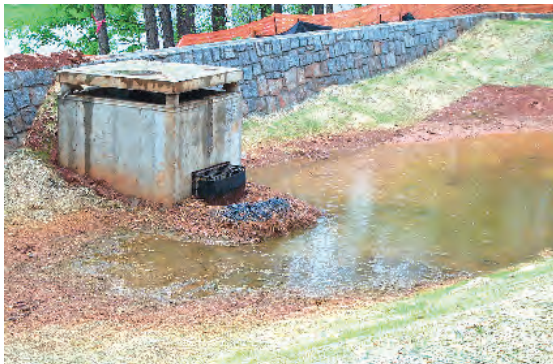
This outlet riser intake hole has been modified with a “half round” section of pipe with 1-inch holes on 6-inch centers and rock berm. This temporary dike provides additional detention during the construction phase, which improves soil removal.
