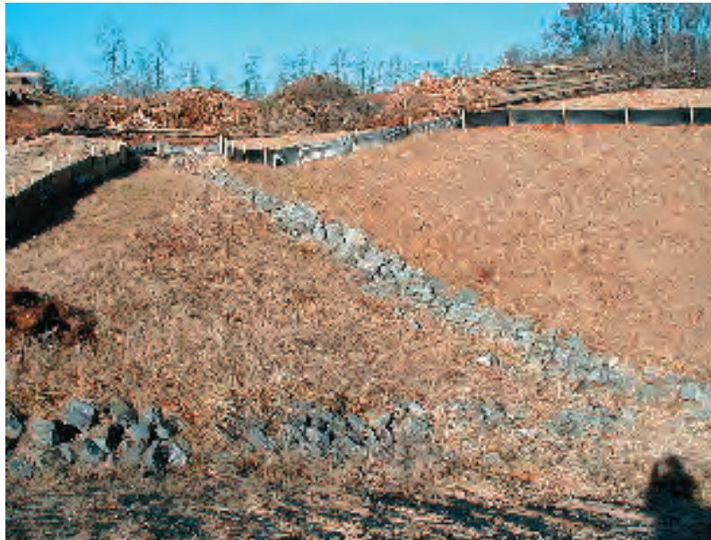
Install silt fencing, sediment traps, and stabilize ditches before clearing and grading. Make sure stakes are on the downhill side of the silt fence!
