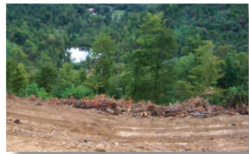
Brush cleared from the site used as a temporary downslope sediment barrier. Make sure barrier intercepts and ponds up muddy runoff. Remove when grass is established.
