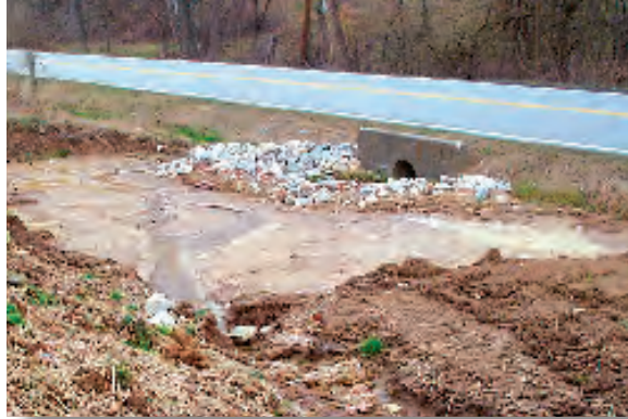
Stone berms placed in front of culvert inlets can trap large volumes of sediment. Make sure sediment is removed as it accumulates to preserve storage capacity for the next storm.
