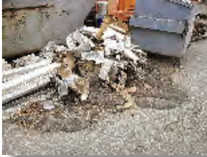
Here is an example of poor waste management. Construction contractors should provide appropriate waste disposal containers, and employees should be instructed to use them.
