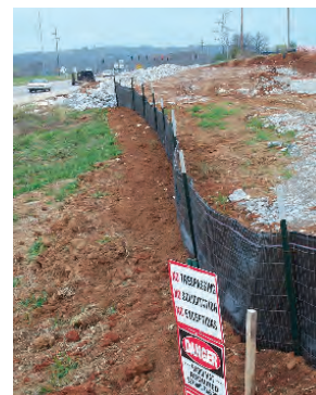
Super (wire reinforced) silt fence in the foreground, supplemented by rock sediment barrier (background). Use rock or other sediment barriers when appropriate.
