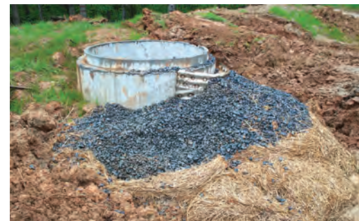
Side slot in drop inlet protected by half-round section of corrugated metal pipe with one-inch holes, held in place by stone berm. This modification can also be used on sediment basin outlet risers.
