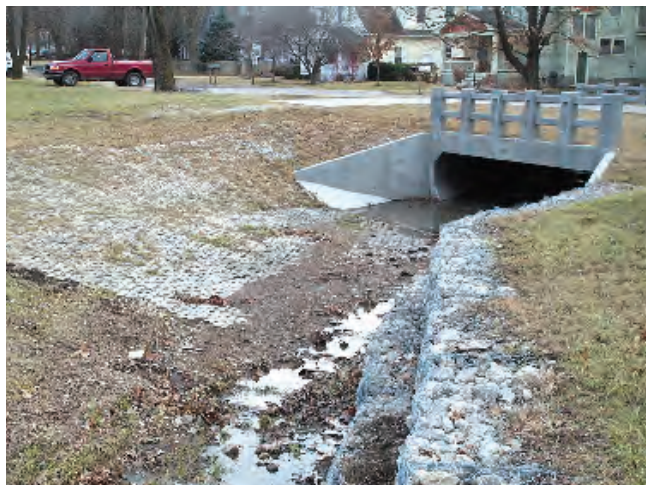
Cellular concrete mat used to stabilize banks in a highly erodible silty loam soil. Double- or triple-seed these applications immediately after installation. Mulch might be needed to support seeded areas until grass is established.
