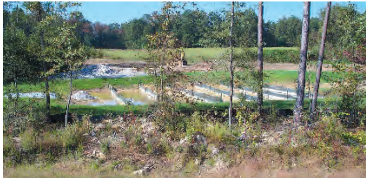
For best results, seed basin sidewalls and upland drainage areas as soon as possible. Make sure outlet structure does not allow rapid flow through the basin—use a rock berm, filter fabric, or other means to maximize ponding and detention time.
