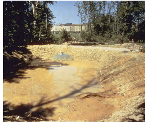
This is a well-constructed sediment basin. Note the rock flow restrictor around outlet riser, which filters and detains inflows. Basin sidewalls should be seeded immediately after construction.
