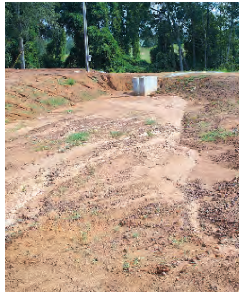
This shows a very well designed detention basin, featuring long flow path between inlet and outlet and V-notched outlet riser, which provides longer detention times for low flow events while still accommodating larger storms. Operation of this basin during the construction phase, however, is very poor. Note the lack of grass on sidewalls; no temporary dike in front of the outlet. This basin appears to be filling rapidly and requires sediment removal. For best results, seed and mulch basins immediately after construction, and modify the outlet to achieve 1 to 2 days of drain-down time after storm events.
