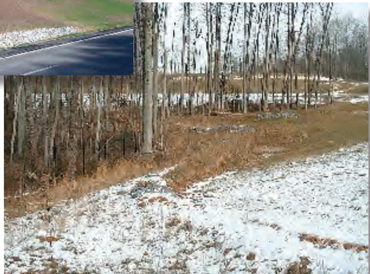
Diversion berm directing runoff toward sediment trap: Controlling sheet runoff with berms and ditches ensures that flows are managed appropriately and provides the framework for a system of sediment traps and basins on larger sites.
