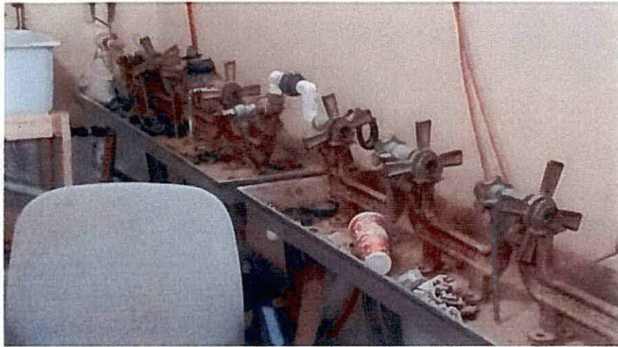
Meter Test Bench
