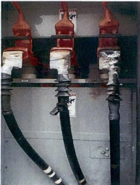
Photo 1. KU Substation initial cable fault on Cir. 45
