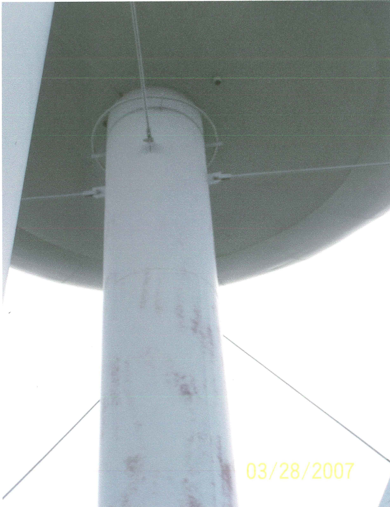
Photo shows the upper section of the riser pipe and the belly rigging rods. There is a rigging ring located at the top of the riser. The surfaces of the bowl are chalky but continue to protect the steel substrate.
