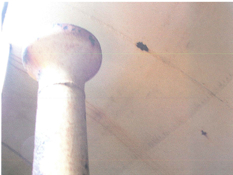
Photo shows the south side of the overflow pipe and the upper section of the roof knuckle just below the roof access hatch. The epoxy coating is mainly failing along the weld seams.
