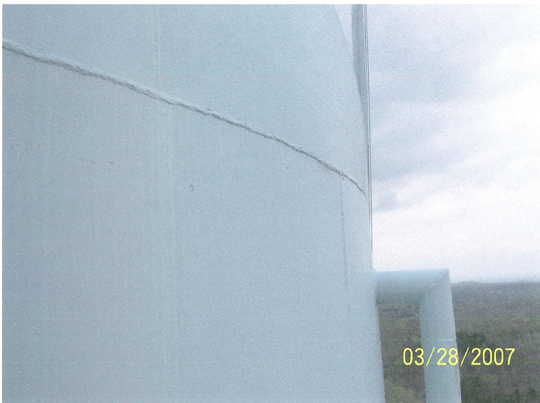
Photo shows the northeast shell. The coating DFT is 4.2 mils in this area. No rust was evident.
