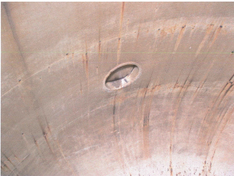
Photo shows the east shell before pressure washing. The majority of the rust nodules are located along the weld seams.
