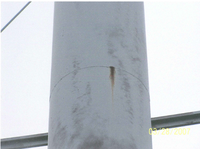
Photo shows what appears to be a small leak in the lower section of the riser pipe. The leak is on the southeast side at a horizontal weld seam.
