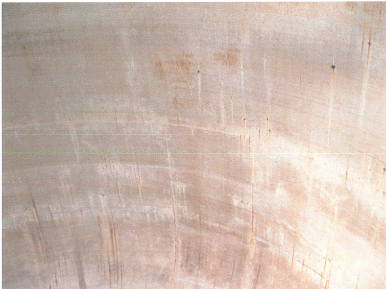
Photo shows the west shell and lower knuckle before pressure washing. Pinpoint rust was noted in the middle section of the shell.
