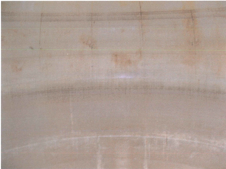
Photo shows the south shell and upper knuckle. Areas of pinpoint rust and blotchy corrosion were noted.
