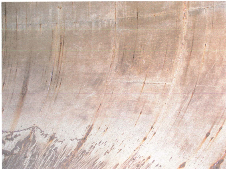
Photo shows the east lower knuckle before pressure washing. Scattered rust nodules were noted.
