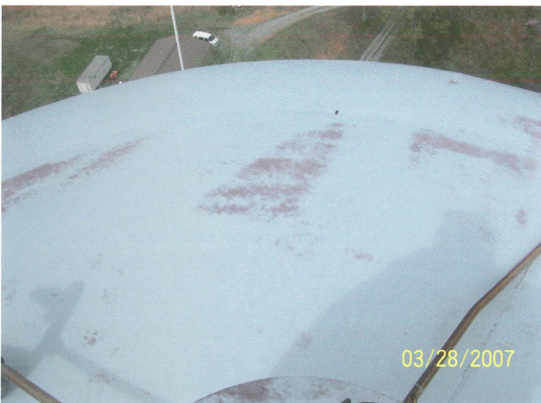
Photo shows the northwest section of the tank roof. All surfaces are chalky.
