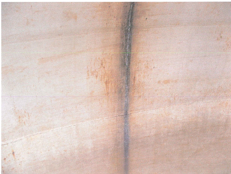
Photo shows another weld seam where the coating no longer exists. The seams that were welded in the field do not appear to have been properly sand blasted and coated.
