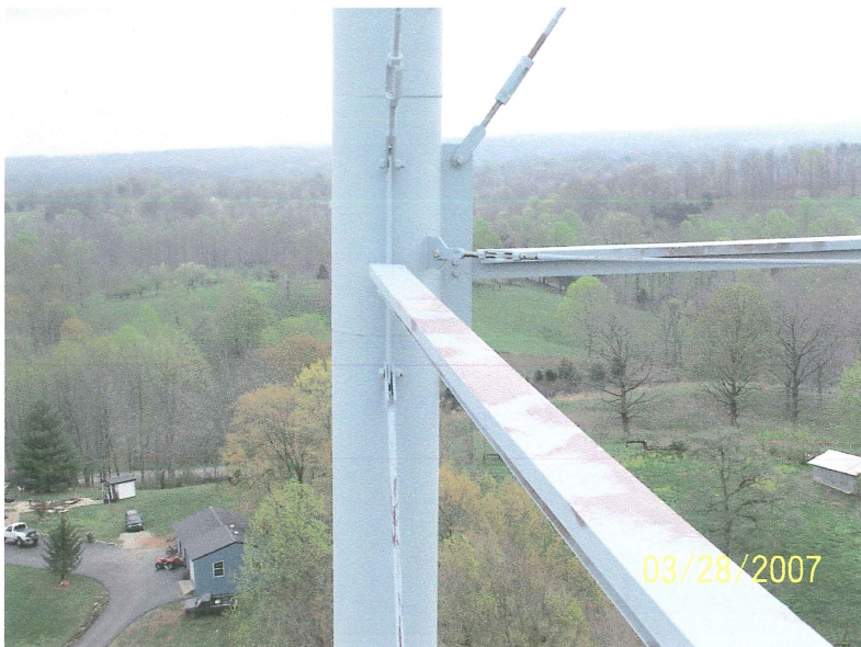
Photo shows the northeast leg at the upper strut level. The average DFT in this area was 3.9 mils. The top strut as well as the middle strut are constructed of 6" channels over 5" channels.
