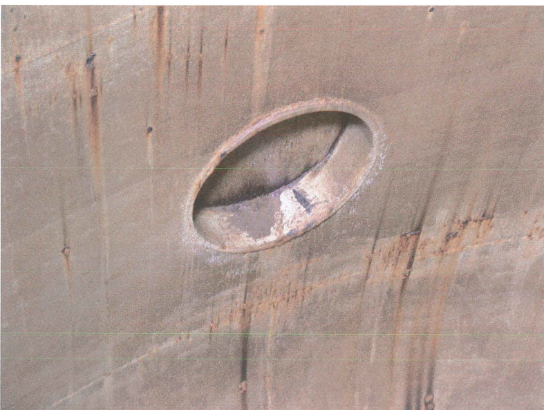
Photo shows a close-up of the 24" diameter shell manway. The gasket should be replaced when the tank is painted.
