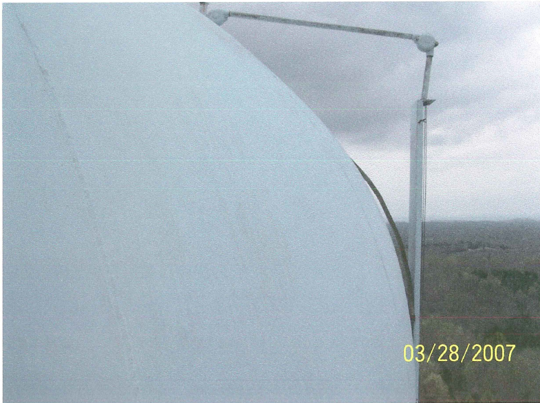
Photo shows the northeast section of the roof knuckle. The average DFT in this area was 3.7 mils. The obsolete level indicator hardware is shown in the background.
