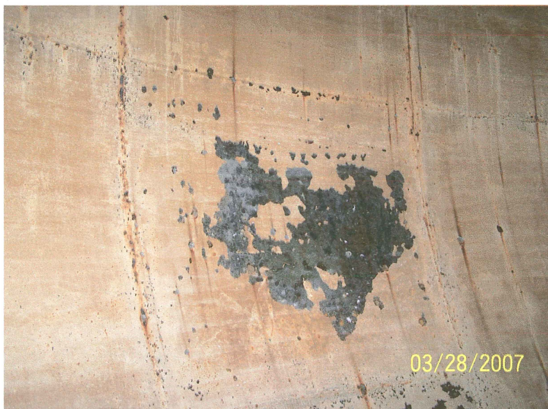
Photo shows the lower shell and upper section of the bottom knuckle. Active corrosion was noted along the weld seams. The tank builder does not appear to have removed the mill scale before applying the coating. The mill scale is hard and smooth and can lead to premature coating failure.
