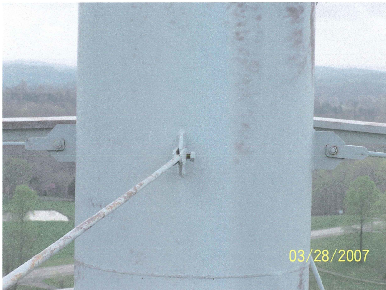
Photo shows the riser pipe at the upper strut level. The connection of the riser stay rods appears to be sound. The blue finish coats have eroded to the red primer on the riser and the rods.
