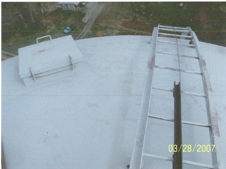
Photo shows the northeast section of the tank roof. the revolving ladder and access hatch are located on this side of the roof.
