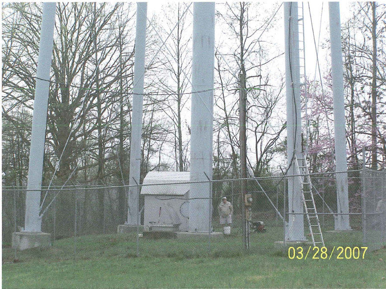
Photo shows the lower sections of all four legs and the 3' riser pipe. A chain link fence encompasses the tank site. The coating shows signs of erosion.
