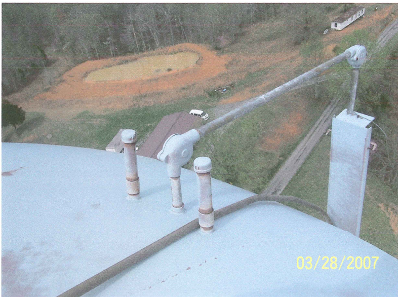
Photo shows the inoperable level indicator hardware. If a telemetry or other level control system is installed this hardware should be removed and the holes should be patched.
