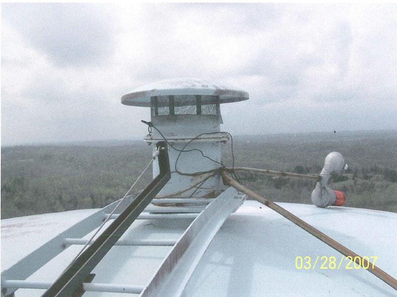
Photo shows the roof vent pipe and the broken aviation light wired to it. A new stand-alone bracket should be welded to the roof to support the aviation light. The small diameter safety cable on the roof ladder should be replaced with a galvanized notch rail.
