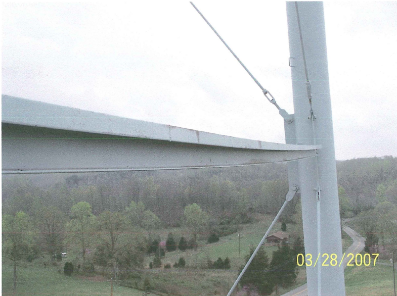
Photo shows the west center strut. The strut is not level. Either the strut was too long and was forced between the legs or the tank has moved since erection causing the strut to bow downward.
