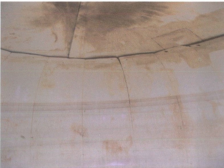
Photo shows the southeast upper knuckle. The white epoxy provides some protection but has reached the end of its life cycle and should be completely removed soon.
