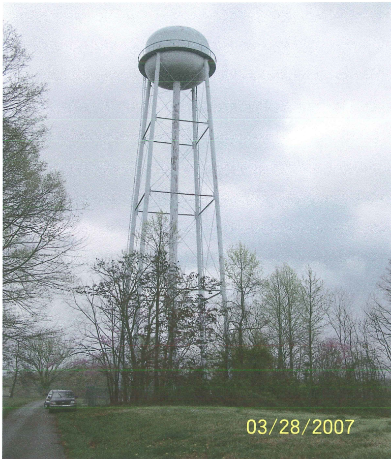
Photo shows an overall view of the southwest side of the tank. The blue finish coat still provides some protection but has lost its gloss and is chalky. Erosion to the red primer was noted on the riser pipe.
