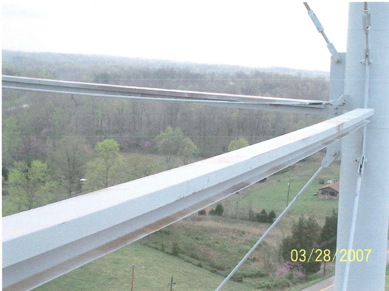
Photo shows the south and west upper level struts. The red primer is visible. The coating is starting to fail on the edges.
