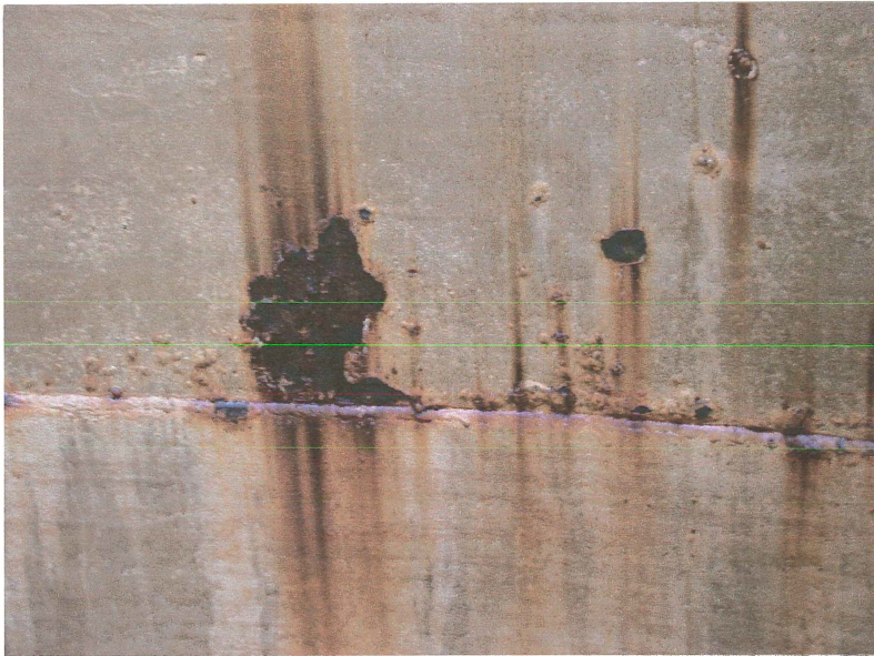
Photo shows a spot on the lower section of the shell where the coating has delaminated to the steel substrate. The white epoxy coating has blistered.
