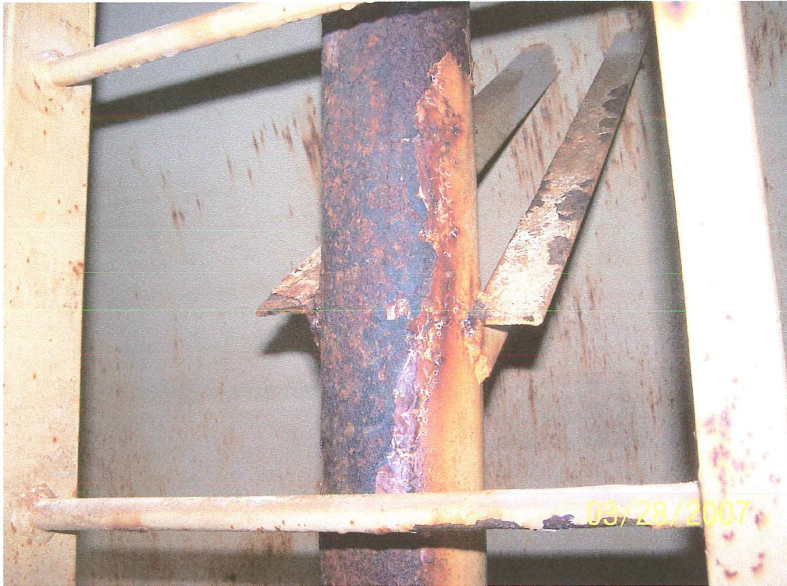
Photo shows total coating failure and heavy rust on the vertical section of the overflow pipe. The angle supports are sound.
