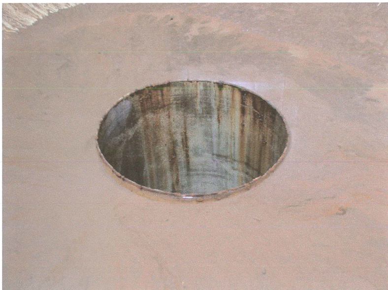
Photo shows the top of the riser pipe and the 2-3" of sludge that covers the floor. A 42" tall handrail with a mid-rail should be installed around the riser opening to protect from a fall.
