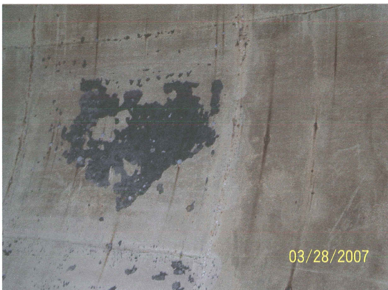
Photo shows the northwest lower knuckle partially pressure washed. The coating is completely delaminating to the steel in numerous locations.
