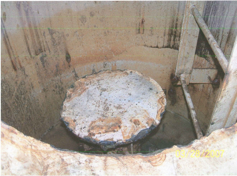
Photo shows the lower section of the 3' diameter riser pipe. The riser has a ladder that is rusty but is in sound condition.
