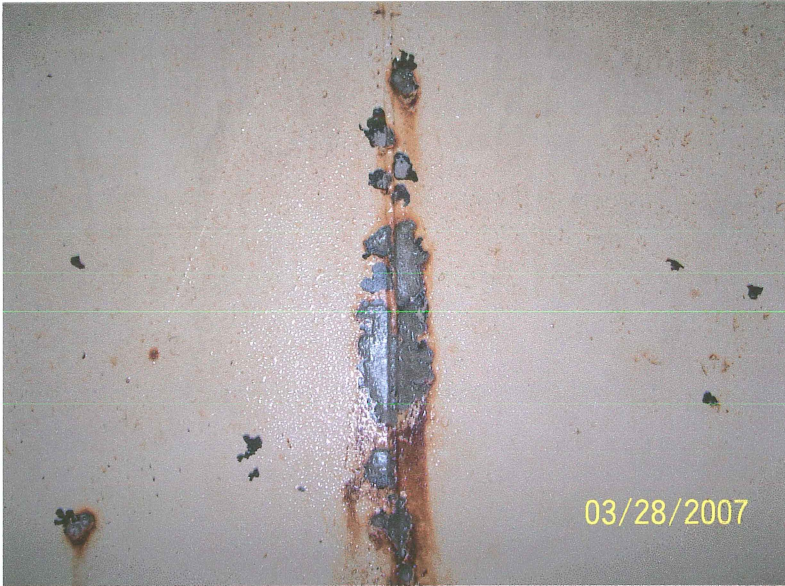
Photo shows blotchy corrosion along a vertical shell seam. Small blisters are evident in the white epoxy coating.
