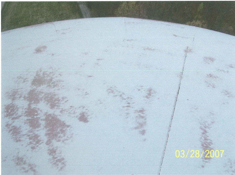
Photo shows the south section of the tank roof. The average DFT is 3.2 mils. Finish coat erosion is widespread.
