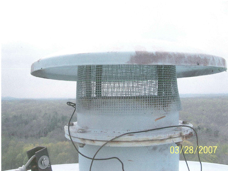
Photo shows the 12" roof vent pipe and protective cover. The vent cover can be removed from the bolted flange. The joint between flanges is rusty. A new stainless steel insect screen should be installed.
