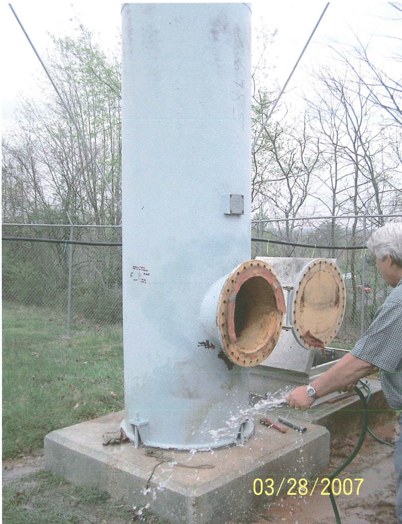
Photo shows the base of the 3' diameter riser pipe. The concrete foundation is in good condition. The coating is heavily chalked. The gasket for the 24" bolted flange access hatch should be replaced.
