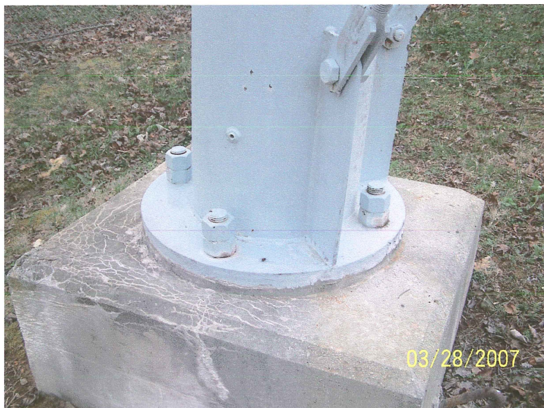
Photo shows the column flanges of the southeast leg. Minor rust was noted on the anchor bolt threads and nuts. The concrete has numerous spider cracks and is starting to spall. Unsound concrete should be removed.
