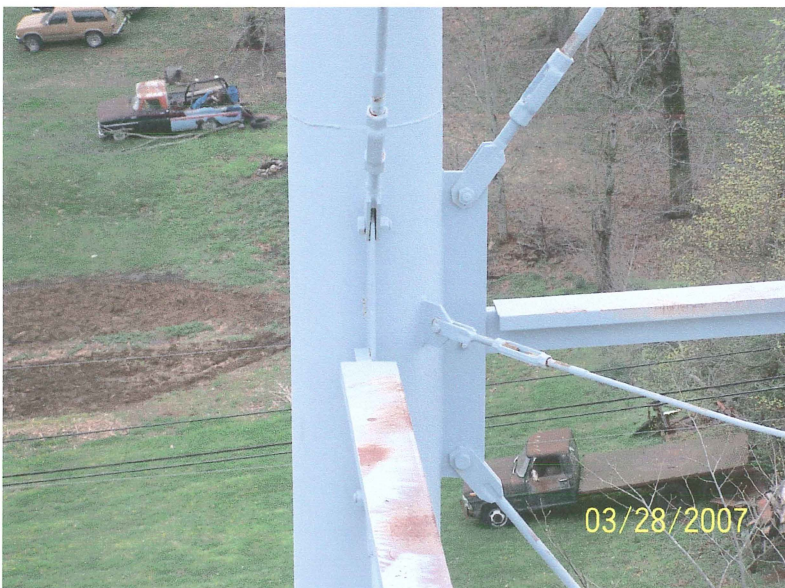
Photo shows the northeast leg at the middle strut connection. The coating on the horizontal surfaces has eroded to the red primer. Minor rust was noted at the turnbuckles.
