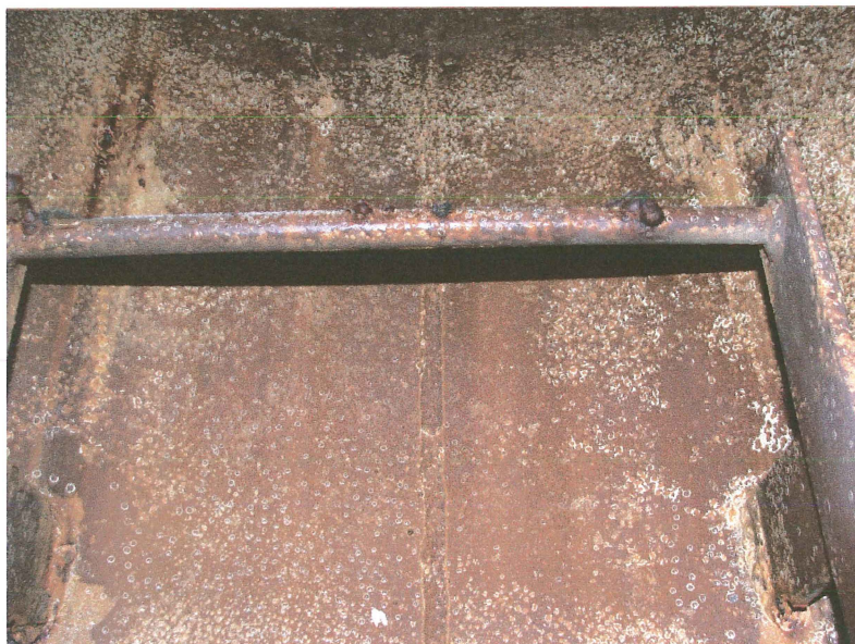
Photo shows the upper end of the riser ladder. The ladder should be extended approximately 3' to allow for safer access.
