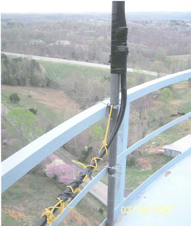
Photo shows an antenna attached to the north side of the balcony handrail. The antenna cables should be placed inside rigid conduit. The antennas should be mounted to stand alone brackets on the tank roof.
