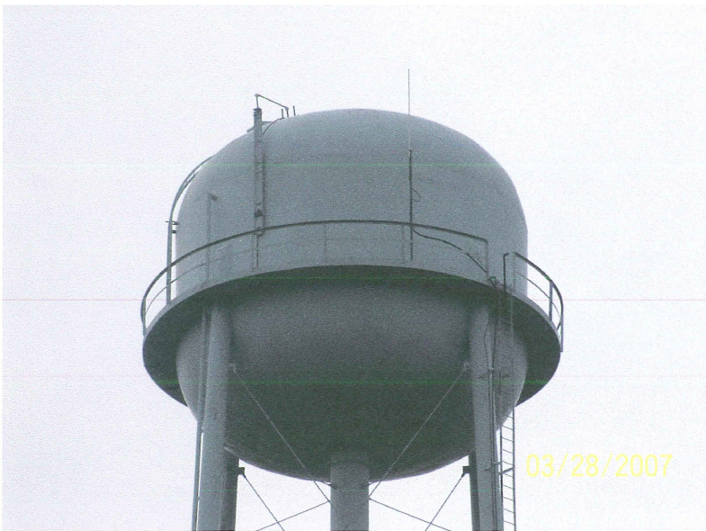
Photo shows the north side of the water-bearing portion of the tank. The level indicator and overflow pipe are visible.
