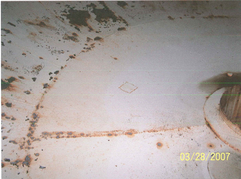
Photo shows the southeast section of the tank bowl after pressure washing and debris removal.
