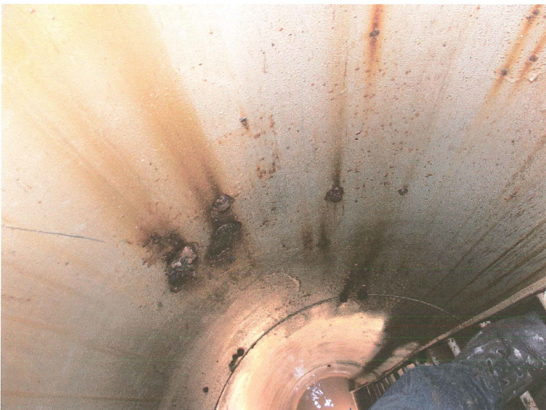
Photo shows the lower 15' of the riser pipe. Scattered areas of blotchy corrosion were noted. The average DFT was 10.8 mils.
