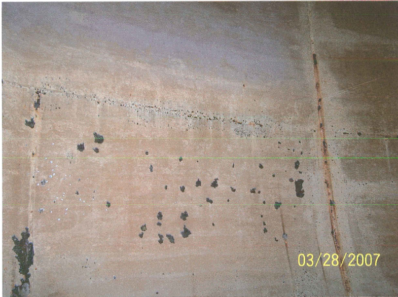
Photo shows the east shell and upper section of the lower knuckle after pressure washing. The dark spots are where the coating delaminated to the steel substrate.
