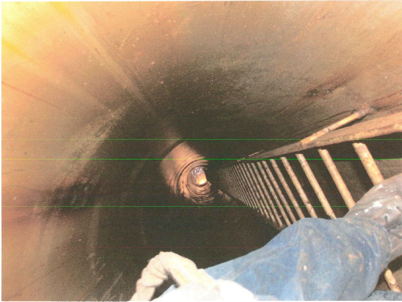
Photo shows the lower 50' of the riser pipe. The white epoxy coating is stained but continues to protect most surfaces. However, active corrosion cells were noted.
