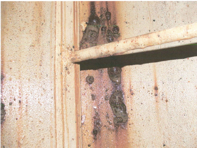
Photo shows rust nodules in the lower section of the riser pipe. Metal loss is active. Some pits area deep enough to require filling with Tnemec series 63-1500 solventless epoxy caulk.
