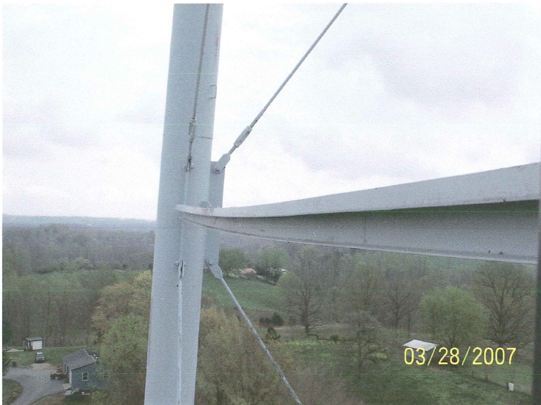
Photo shows the north middle strut. This strut also has a downward bow. The coating is starting to fail along the edges.
