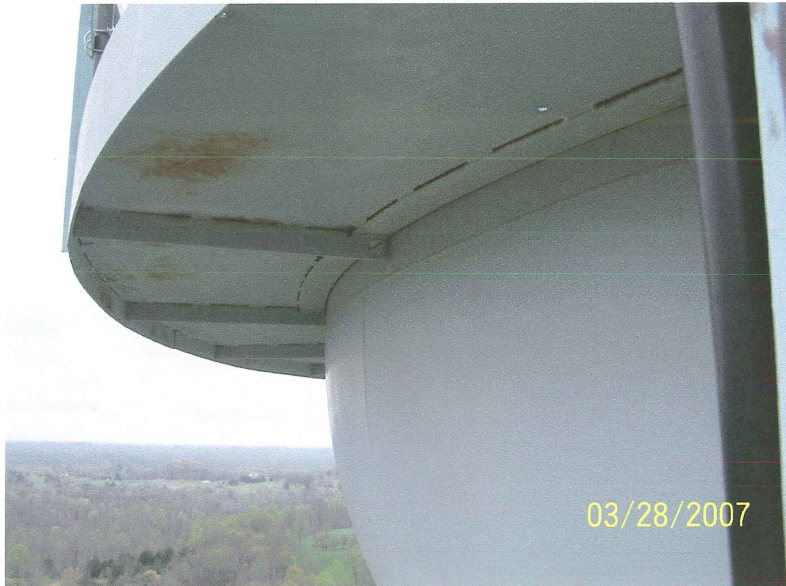
Photo shows blotchy corrosion on the underside of the north section of the balcony.
