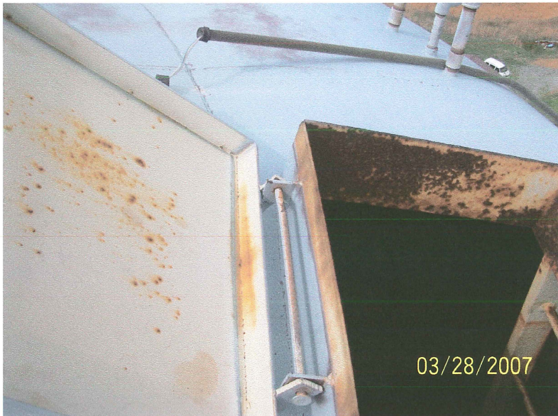
Photo shows rust on the inside of the hatch cover and frame. The hinge is in working order but is not structurally significant. Two new hinges with \frac{3}{4} " stainless steel bolts should be installed.
