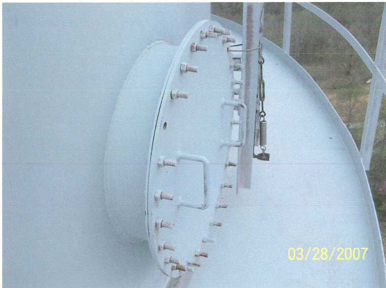
Photo shows the 24" diameter shell access hatch cover. Two bolts are missing from the hatch. A new gasket should be installed.
