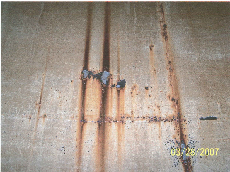
Photo shows white metal where the pressure washer removed the rust nodules. Metal loss is active. These spots will soon become leaks if no repaired.
