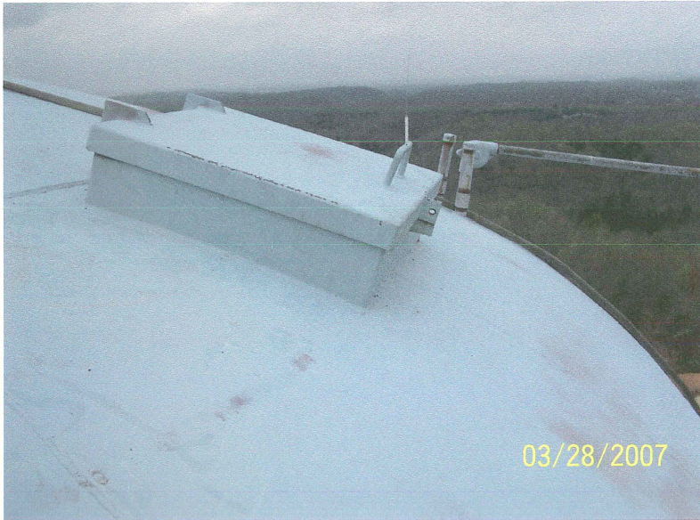
Photo shows the 24" square roof access hatch. The hatch meets current AWWA D100 requirements. The hatch has a lockable hasp but was not locked.
