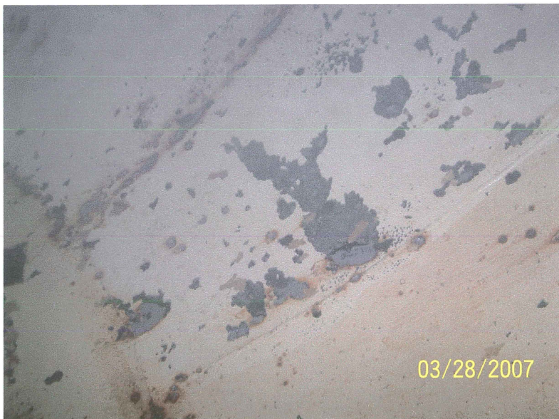
Photo shows the partially cleaned southwest lower knuckle. The coating has delaminated to the steel in large areas.
