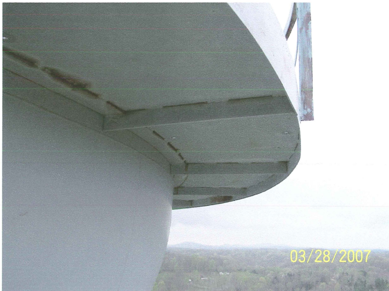
Photo shows the west underside of the balcony. Corrosion was noted along the edges.
