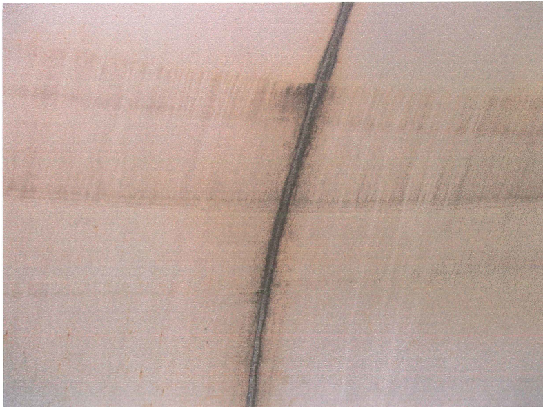
Photo shows total coating failure along a vertical upper knuckle weld seam.
