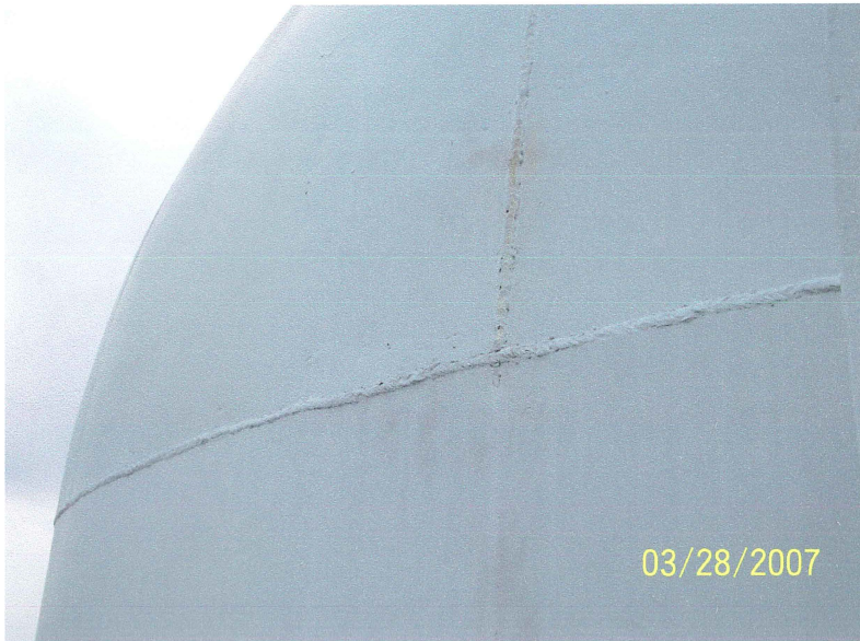
Photo shows minor rust and top coat erosion on the east upper shell and lower section of the upper knuckle.
