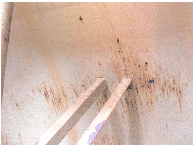
Photo shows active corrosion in the middle section of the northeast upper knuckle where the overflow pipe braces attach.
