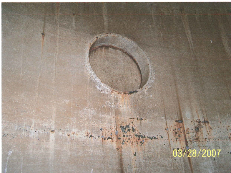
Photo shows the east shell and the 24" diameter shell manway after water blasting. The white epoxy is stained but continues to protect most surfaces. The average DFT is 12.3 mils.
