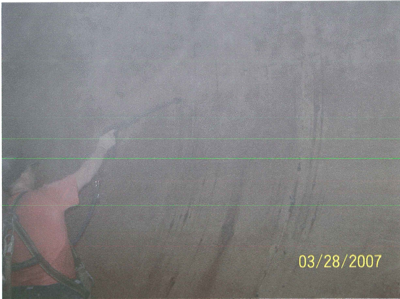
Photo shows the inspector using a 4,00-psi water blaster to clean the shell and lower knuckle.
