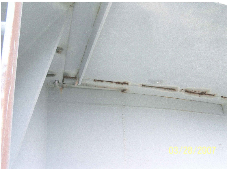
Photo shows crevice corrosion along the skip welded balcony floor seams. These seams should be sealed with caulk.
