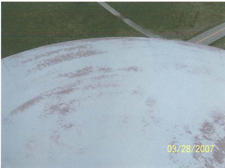
Photo shows the southeast section of the tank roof. All surfaces are eroded and chalky.
