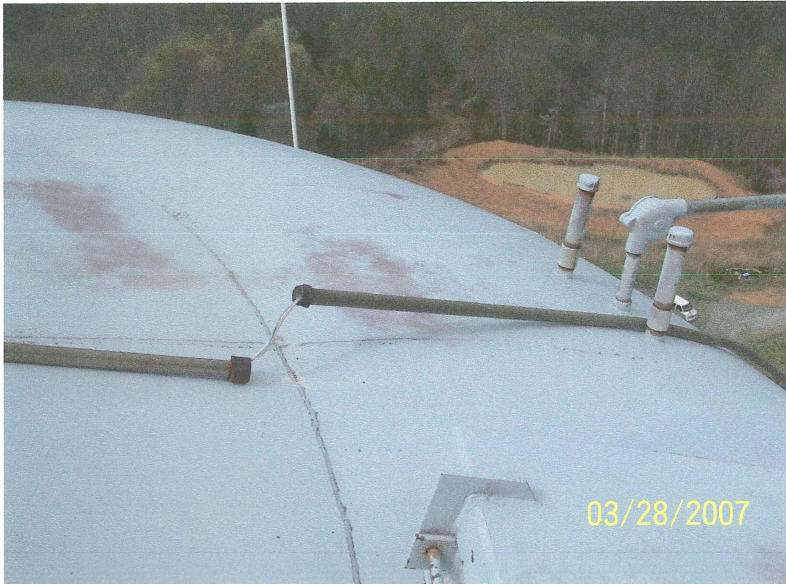
Photo shows another broken conduit coupling for the wiring leading to the aviation light.
