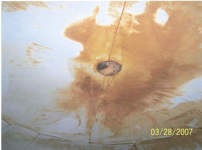
Photo shows and overall view of the roof cap plate. The inside of the 12" diameter vent pipe is heavily rusted. Light orange rust covers the majority of the roof cap plate.
