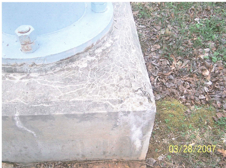
Photo shows an additional area of deteriorated concrete on a leg base. New high strength grout should be placed to replace the unsound concrete removed. All concrete surfaces should be sweep blasted and coated with two coats of epoxy.
