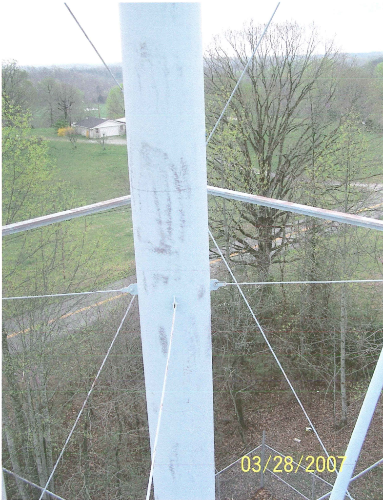
Photo shows the riser pipe at the lower strut level. The connection of the riser stay rods appears to be sound. The blue finish coats have eroded to the red primer. All surfaces are chalky.
