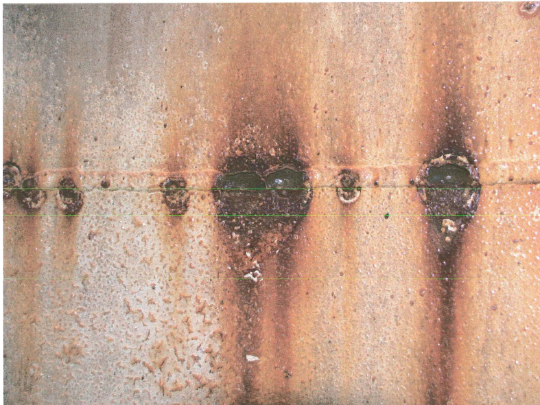
Photo shows active corrosion along a horizontal weld in the middle section of the riser pipe. Pitting is shallow.
