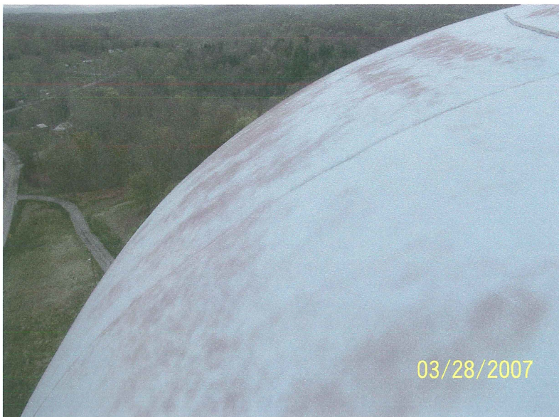
Photo shows wide spread erosion of the blue finish coat to the red primer on the southeast upper knuckle. The coating is less than 3 mils thick in most areas.
