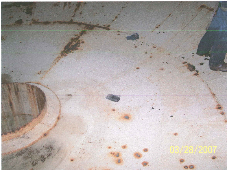
Photo shows the west section of the bowl after pressure washing. Scattered rust nodules were noted but were heaviest along the weld seams. A 42" tall handrail should be installed around the riser opening to prevent an accidental fall.
