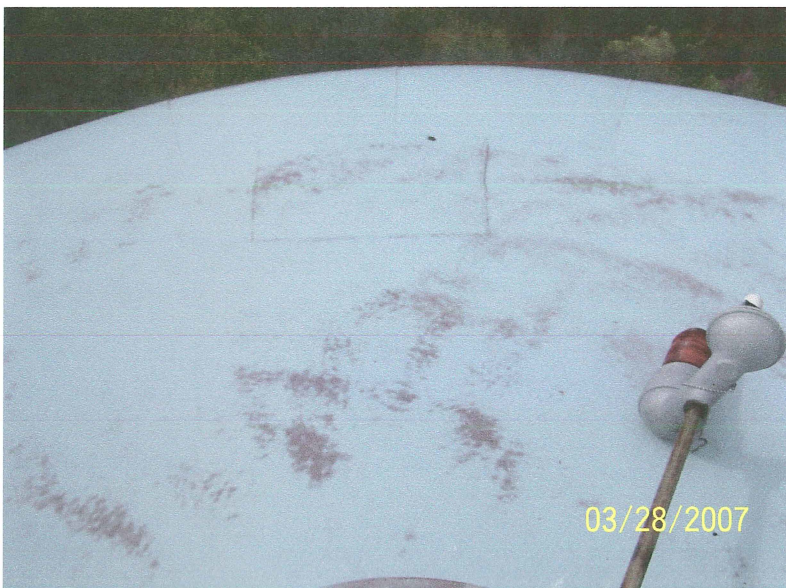
Photo shows the west section of the tank roof. Erosion has allowed the red primer to be exposed. The broken aviation light is laying on the roof.
