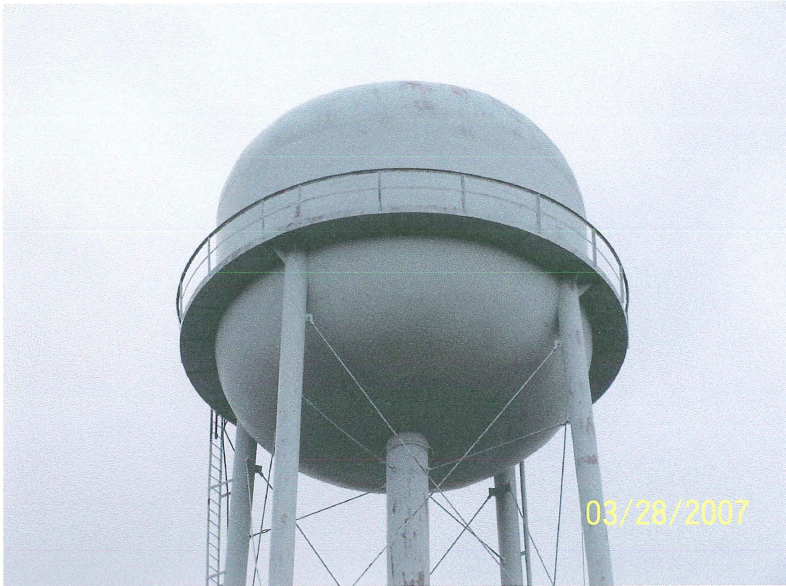
Photo shows the south side of the water-bearing portion of the tank. Erosion to the red primer is visible on the south upper knuckle.
