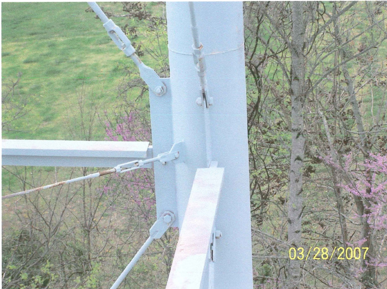
Photo shows the southwest leg at the lower strut level. The windage rods, riser stay rod and struts connect to the leg at this point. The coating is failing on the riser stay rod and has eroded to the red primer on the horizontal surface of the strut.
