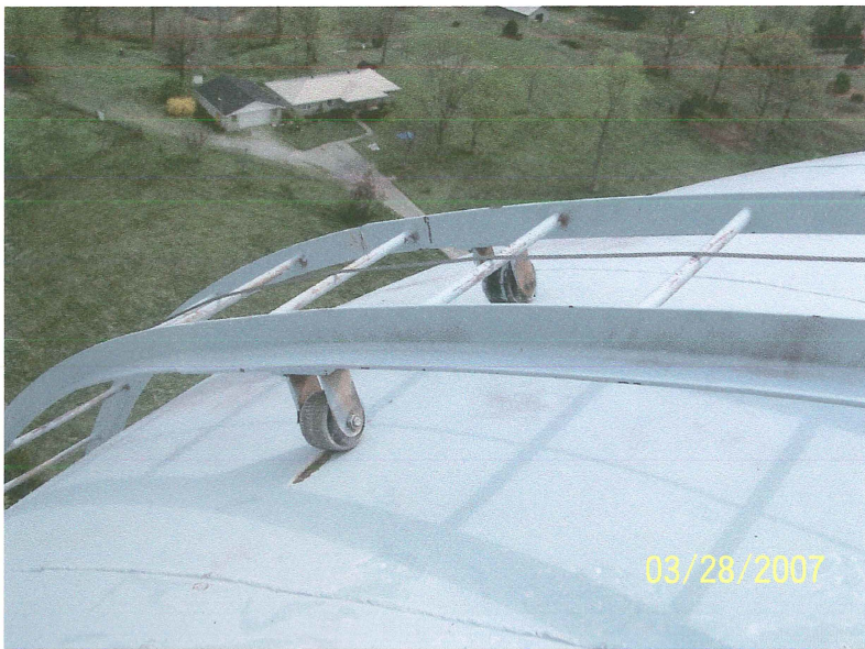
Photo shows the revolving roof ladder. The wheels should be removed and the ladder should be secured to the roof by welding.
