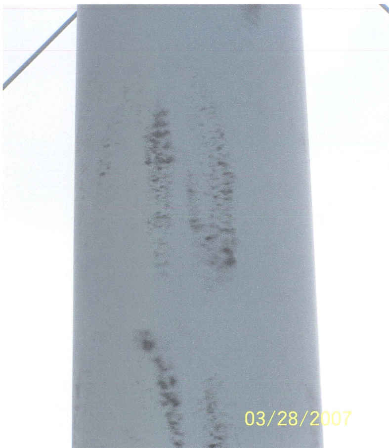
Photo shows a close-up of the eroded riser pipe surfaces. The coating that remains is less than three mils thick in many areas.
