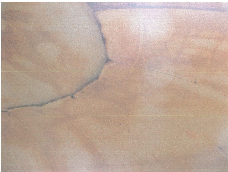
Photo shows pinpoint rust covering all surfaces of the northwest upper knuckle.
