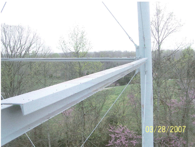
Photo shows the lower west side channel strut. The strut has a 7" channel on top and a vertical 5" channel beneath. The blue finish coat has eroded to the red primer.
