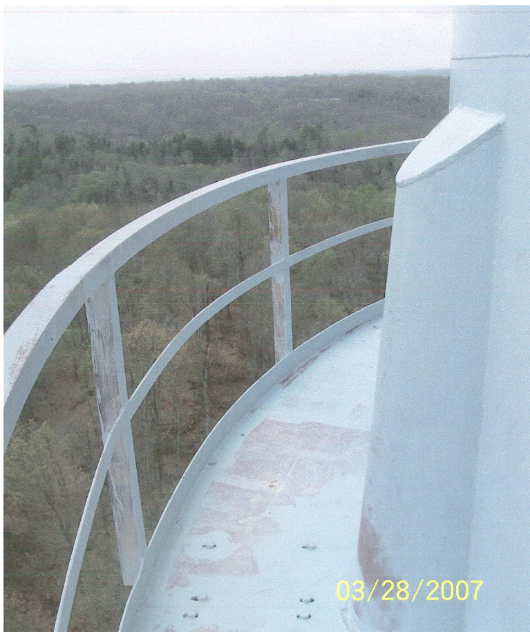
Photo shows the southwest section of the balcony. The balcony is 31" wide and has a 42" tall handrail. The red primer is visible on most surfaces.
