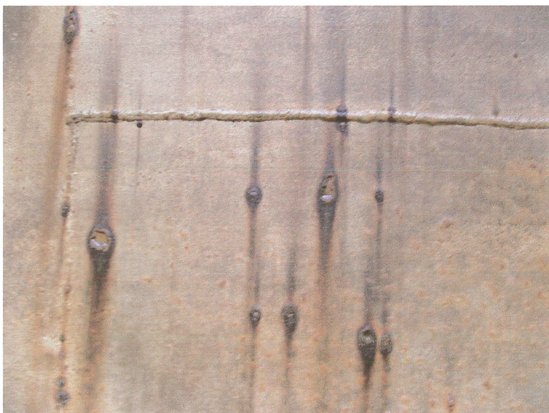
Photo shows rust nodules on the lower knuckle before pressure washing.
