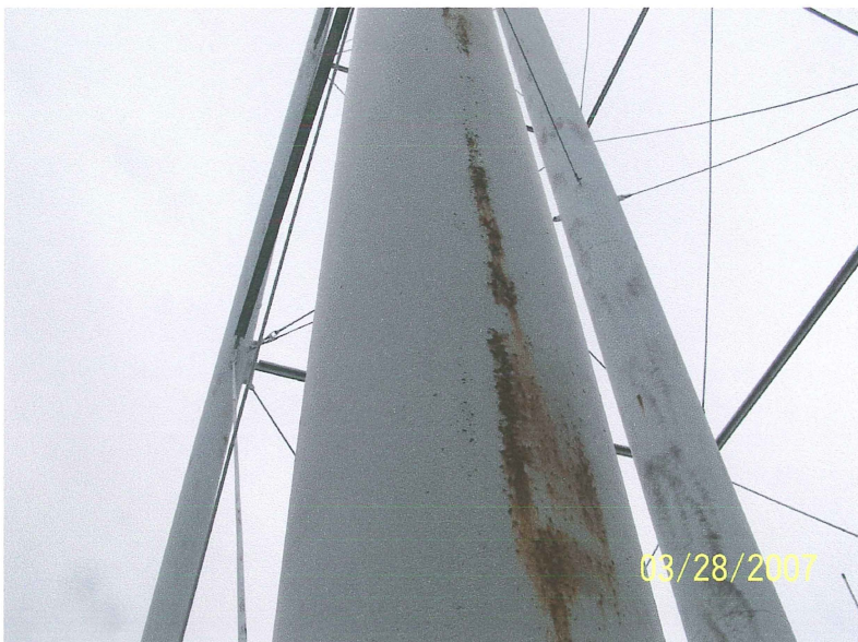
Photo shows blotchy corrosion on the east side of the lower section of the southeast leg.
