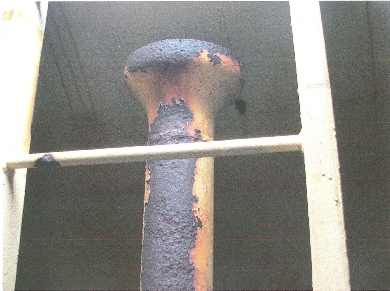
Photo shows the upper west side of the overflow pipe and the top section of the tank ladder. The pipe is pitted and may require some pit filling. The ladder is in good condition.
