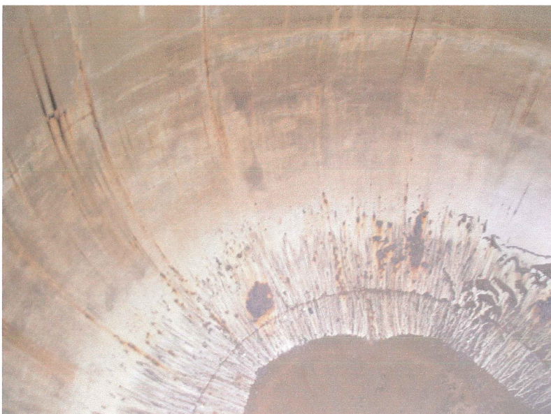
Photo shows an overall view of the northeast lower knuckle before pressure washing. Active corrosion cells were noted on all surfaces.
