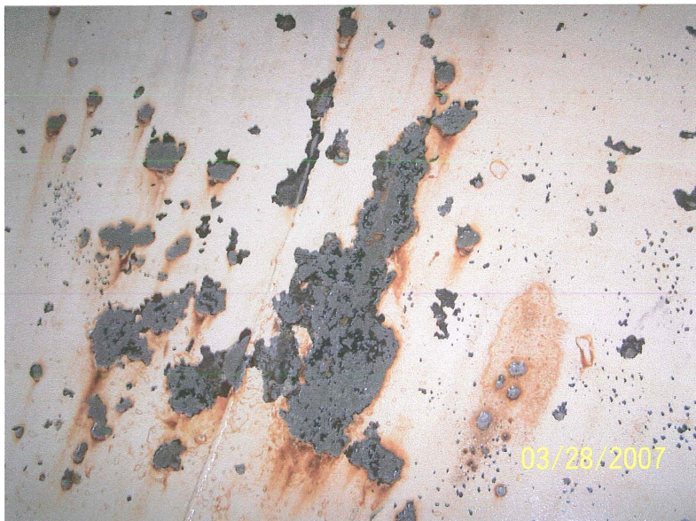
Photo shows the middle section of the northwest lower knuckle. The white epoxy has blistered and is delaminating to the steel. The remaining coating should be removed by blasting per SSPC-SP10.
