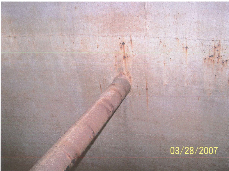
Photo shows the vertical section of the overflow pipe where it exits through the northeast section of the upper shell. Blotchy corrosion was noted on most surfaces.
