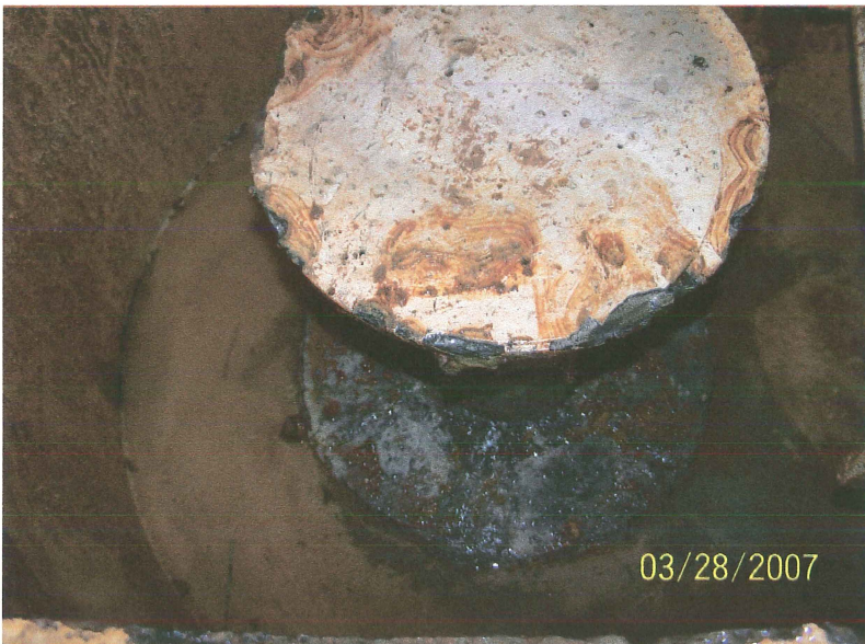
Photo shows the fill pipe and floor of the riser pipe after sludge was removed. The coating has failed on the edges of the fill pipe's protective cover.
