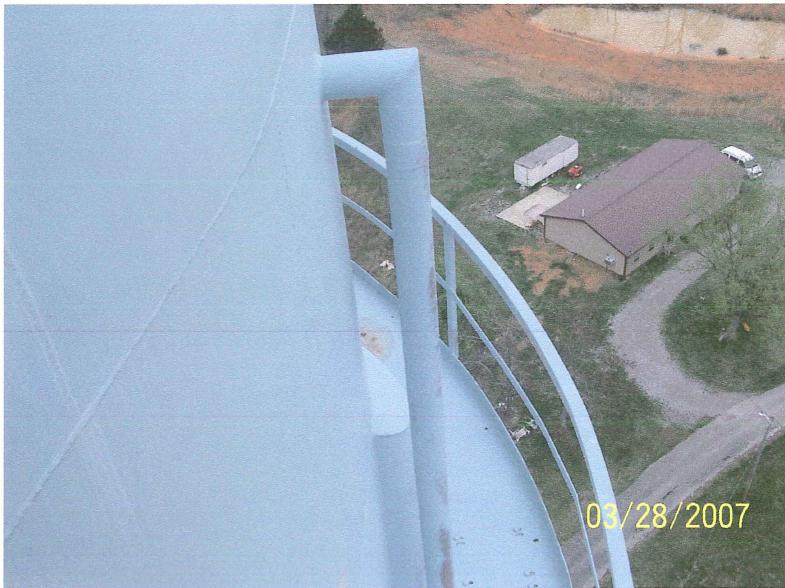
Photo shows the overflow pipe where it exits through the upper shell and runs down through the balcony. The coating on the shell is chalky but continues to provide some protection.
