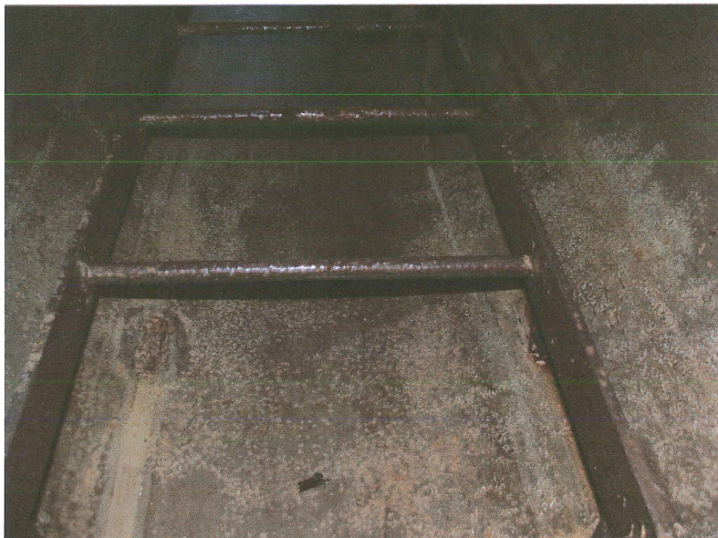
Photo shows the condition of the ladder in the upper middle section. The ladder is structurally sound but does not have a fall prevention device.
