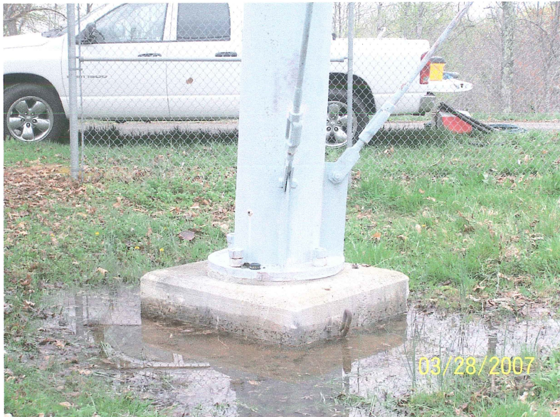
Photo shows the base of the southwest leg and the concrete foundation. The earth around this leg has settled. Fill dirt should be added.
