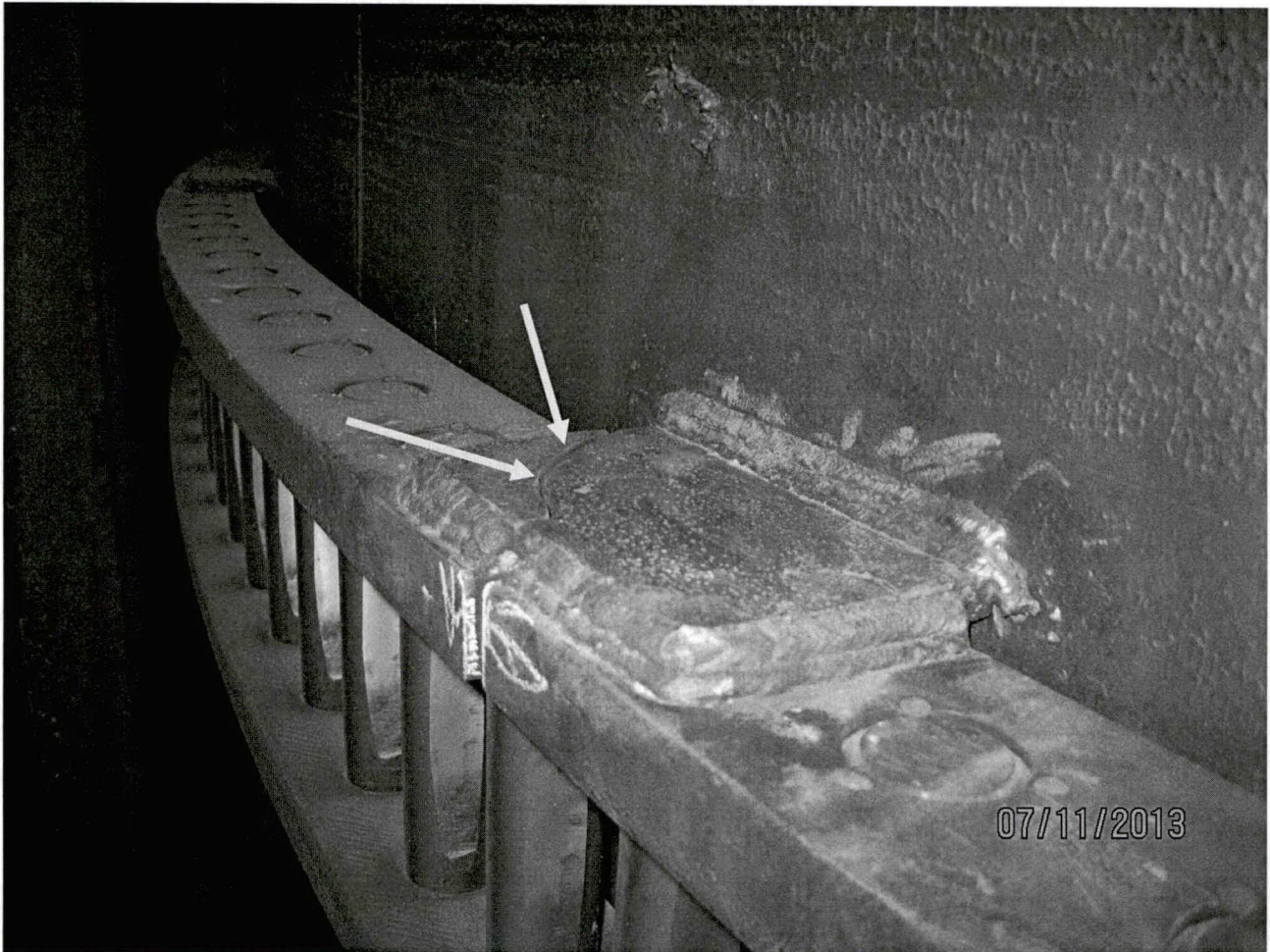
Picture taken during 1A Air Heater inspection showing cracked splice plate on rack drive portion.
