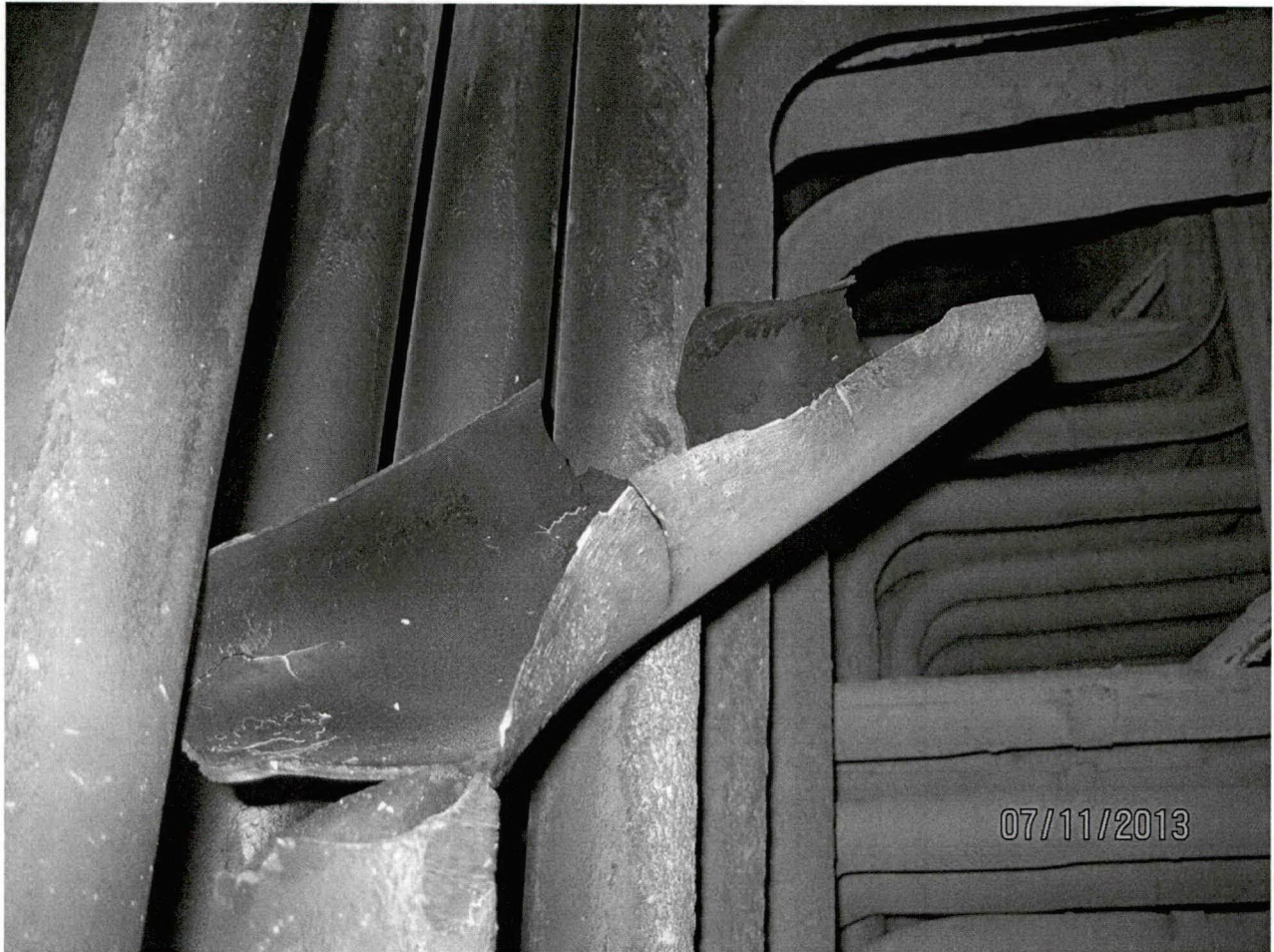
Picture showing tube leak at Reheat Intermediate Bank Lead 21 st bundle from West, 1 st tube from South.
