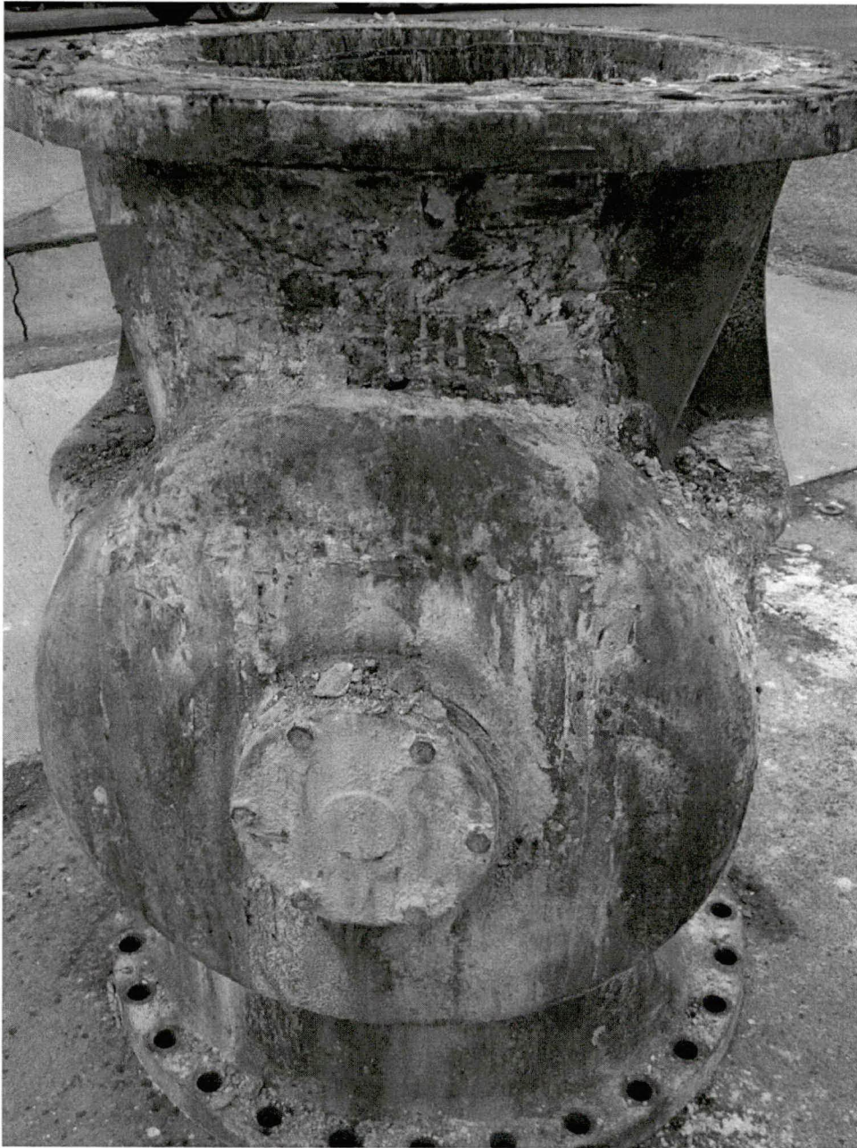
2B Recycle Pump Discharge Valve after removal.
