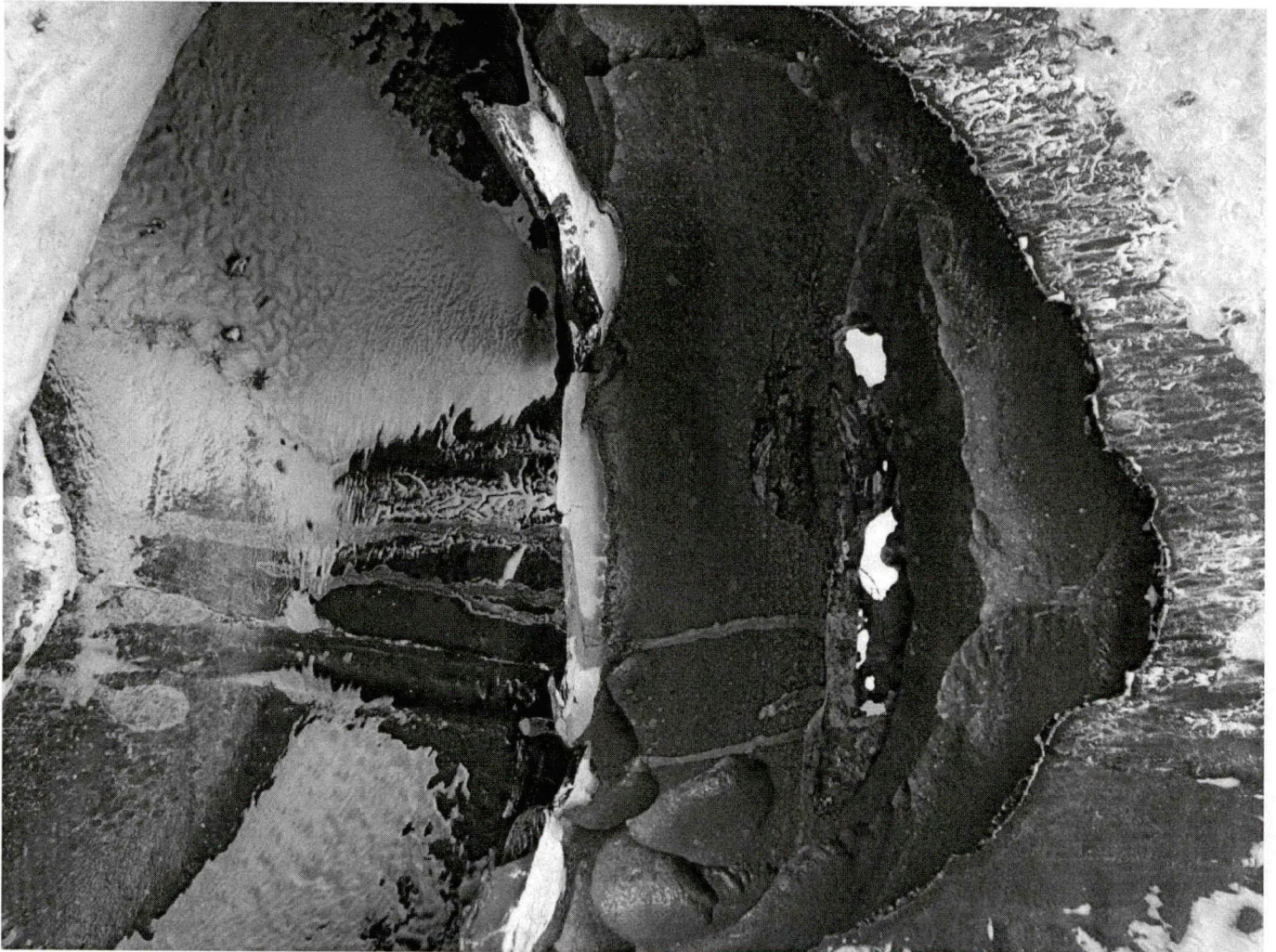
Inside view of valve shows erosion and wear of liner with multiple holes.
