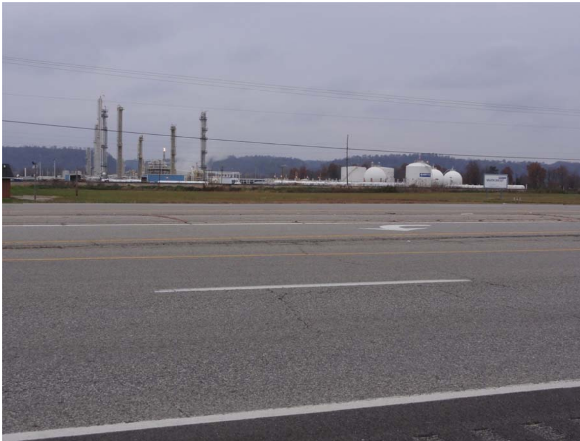
Figure C-2. MarkWest Siloam Kentucky Plant
