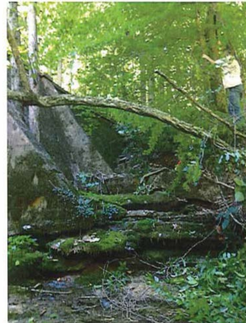
Buttresses and Toe of Rio Verde Dam
