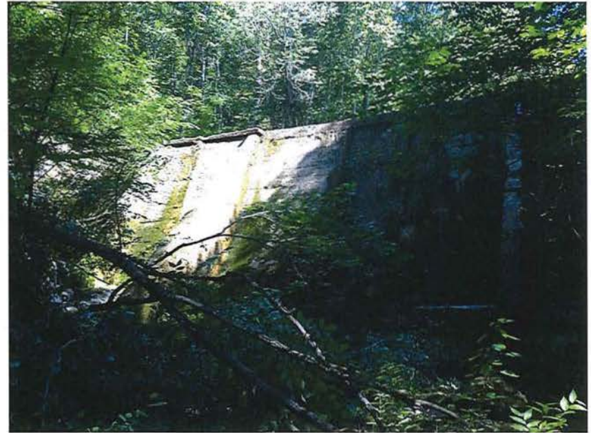
Downstream View of Rio Verde Dam
