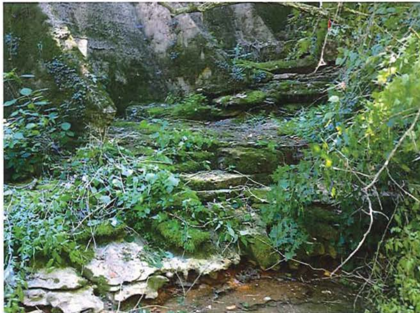
Buttresses and Toe of Rio Verde Dam
