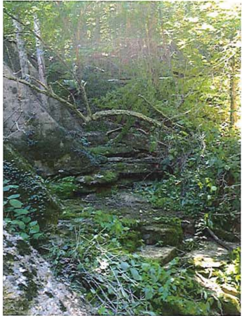
Buttresses and Toe of Rio Verde Dam
