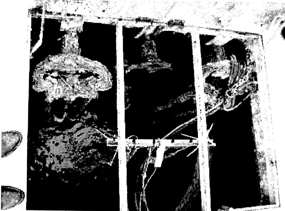
Wet Well - Guide rails and signs of severe corrosion
