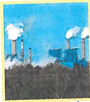
Sebree Station Green Units 1 & 2 Reid Unit 1 Reid Combustion Turbine HMP&L Station Two - Units 1 & 2
