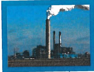
B Coleman Plant Units 1,2,3
