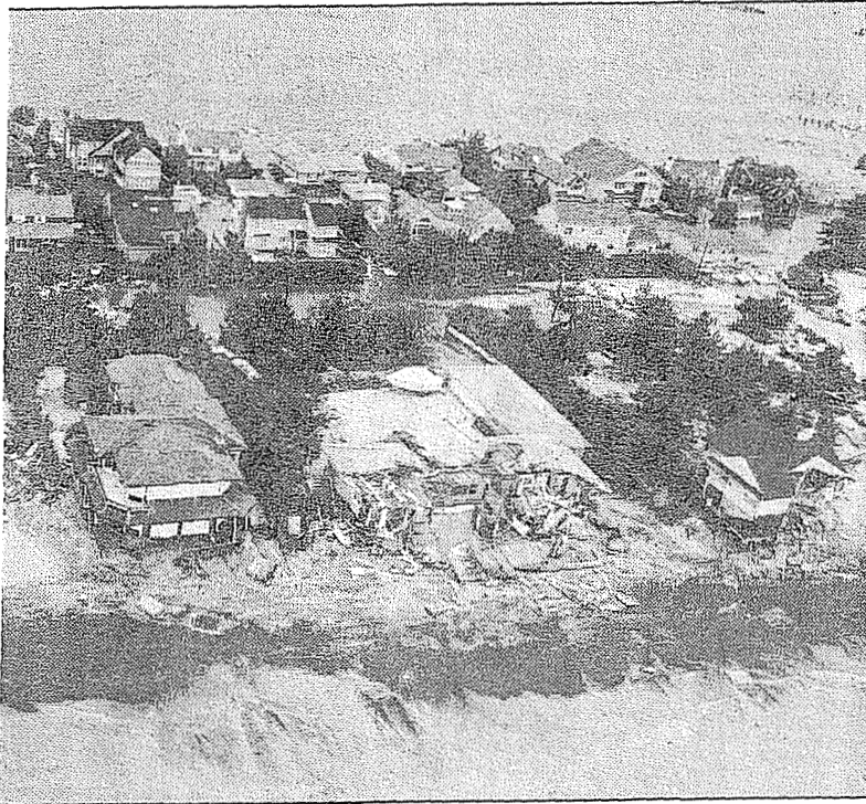
This photo provided by the U.S. Air Force shows an aerial view of damage to the New Jersey shoreline following Superstorm Sandy. A rising number of homes damaged by Sandy are hitting the real estate market.
