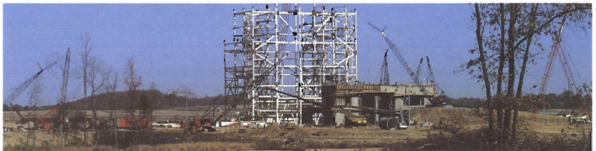
Steelwork went up at the D. B. Wilson plant site this summer. Despite near record rainfall during the spring, construction schedule for Unit No. 1 was two weeks ahead of the timetable at year's end.
