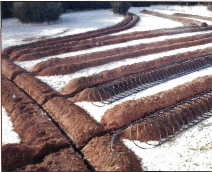
Installation of Geothermal Loop "Slinky"
