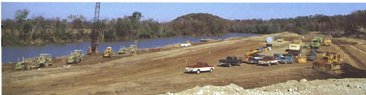
The Green River bank was cleared, and site preparation for the barge unloading dock and related facilities got under way this year at the Wilson plant.
