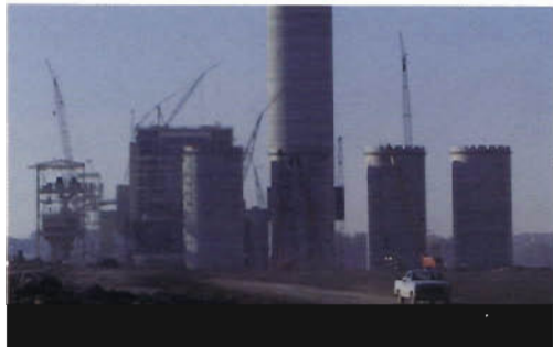
Keeping the air and water clean is expensive. The cost of flue gas desulfurization scrubbers and related environmental facilities (such as the limestone silos pictured above) at the D. B. Wilson Plant will total $152 million, or 23 percent of the Wilson construction cost.
