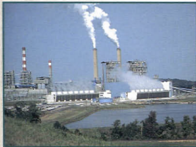
Reid/Green Plant HMP&L Station Two
