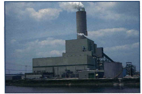
Big Rivers' Wilson Plant located near Centertown, Kentucky 420-MW net capability
