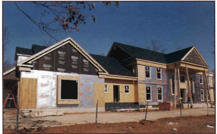
Construction of an All Seasons Comfort Home
