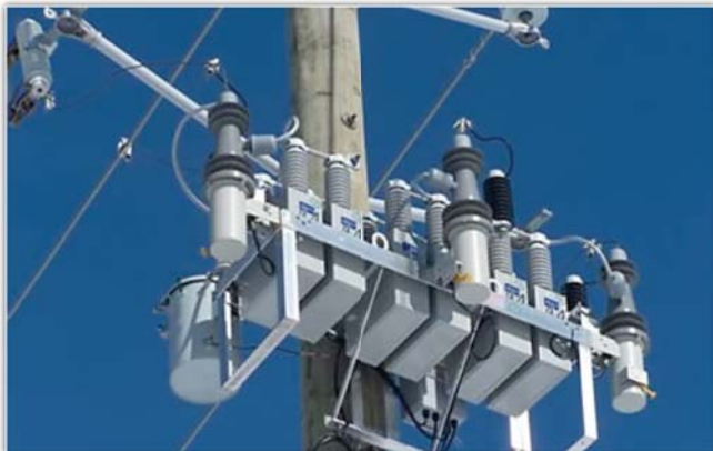
Figure 2: Automated distribution capacitor banks
