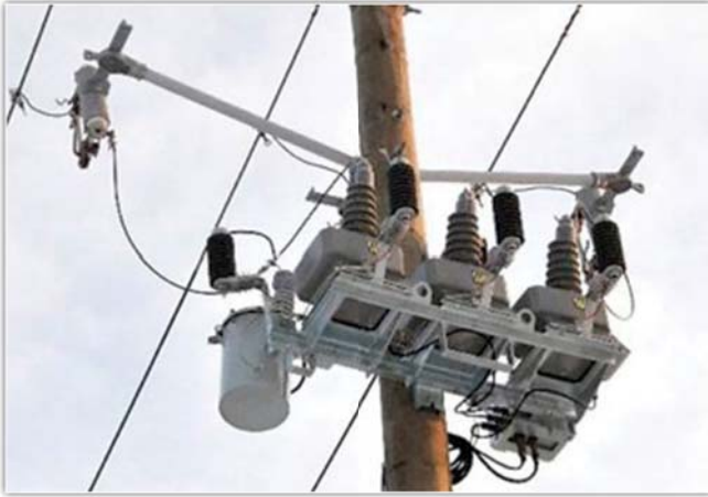
Figure 1: Medium voltage monitoring stations
