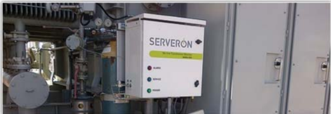
Serveron Transformer Monitor – GE ODU
