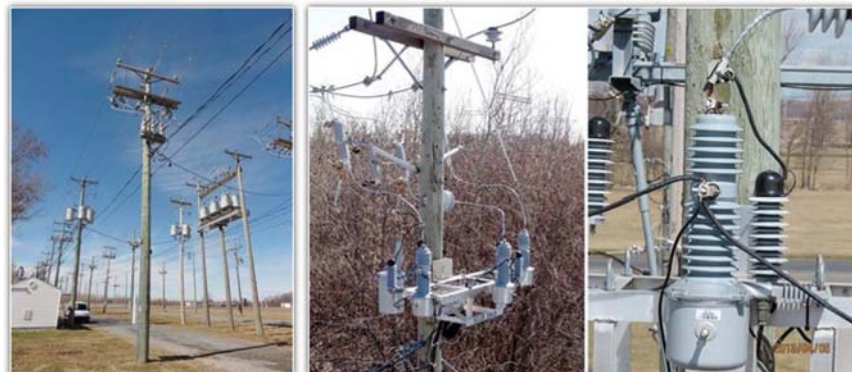
Left is sectionalizing switch; middle and right show autoground switch
