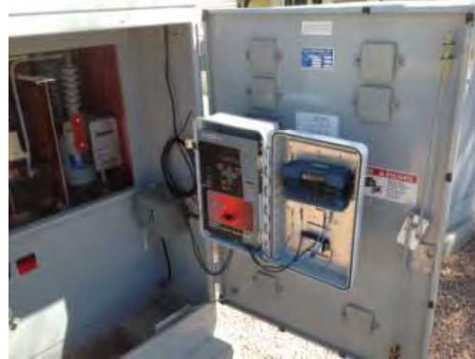
Two-way capacitor bank monitors and controllers, for volt/var control: Control, voltage, temperature
