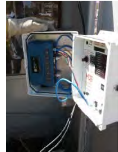
Two-way capacitor bank monitors and controllers, for volt/var control: Control, voltage, temperature
