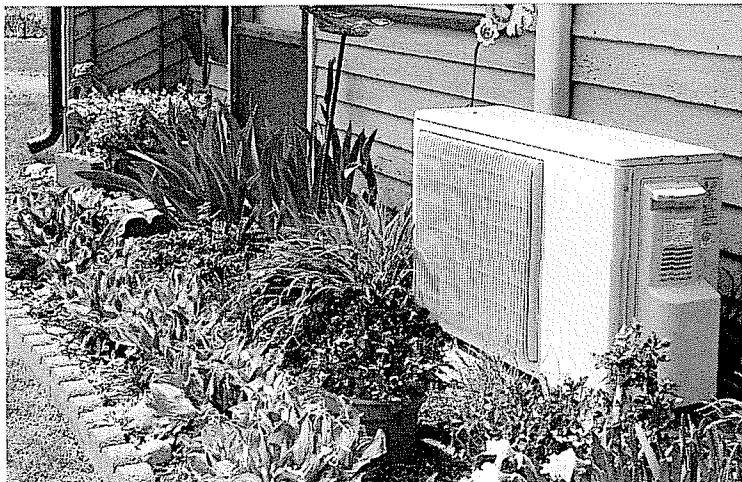
Ductless heat pump outdoor unit
