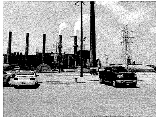
Exiting Plant from employee parking lot
