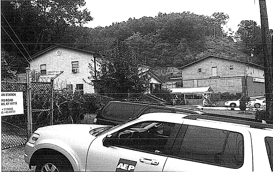
Bonnyman Substation Expansion Site
