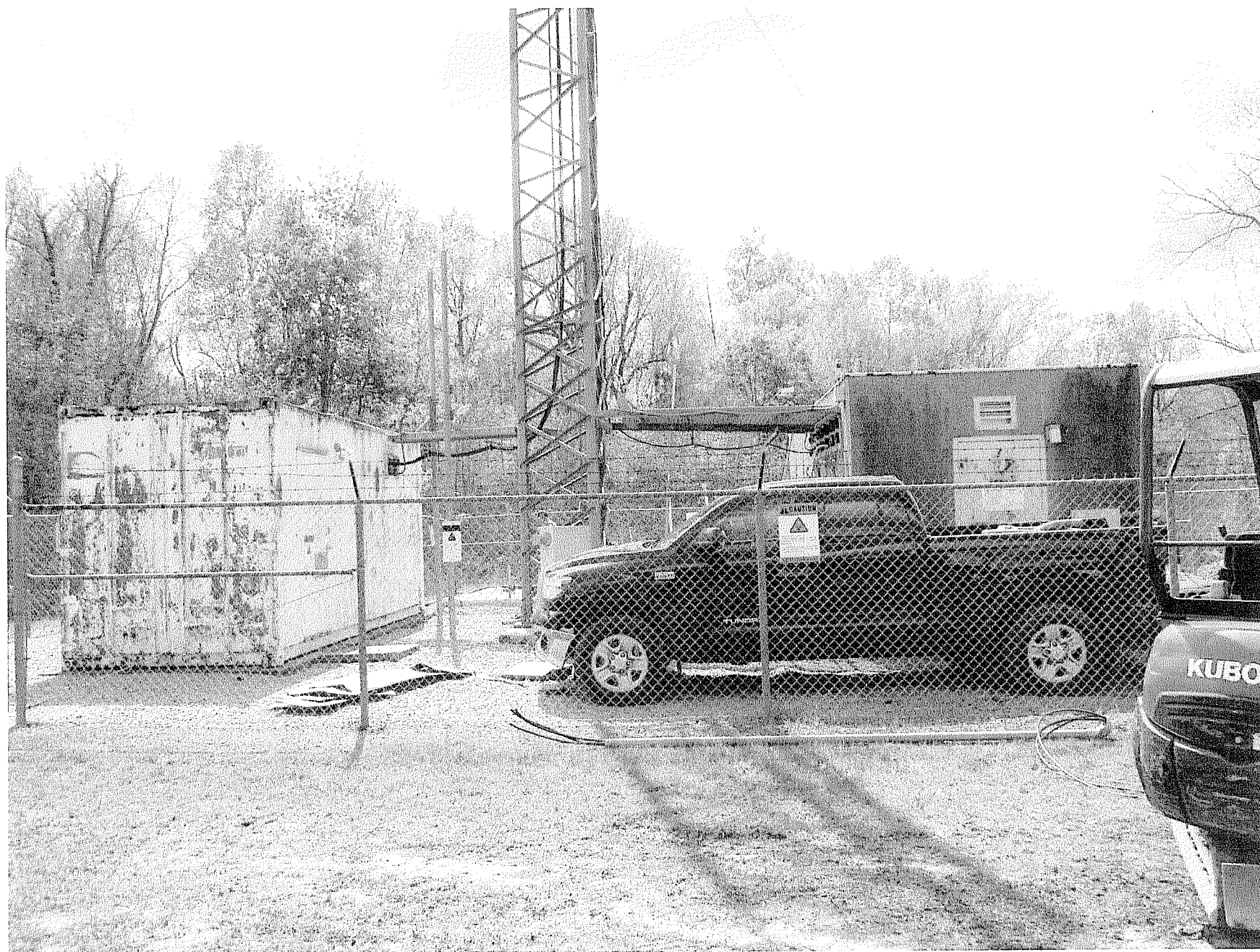
Typical HALO Tower Site
