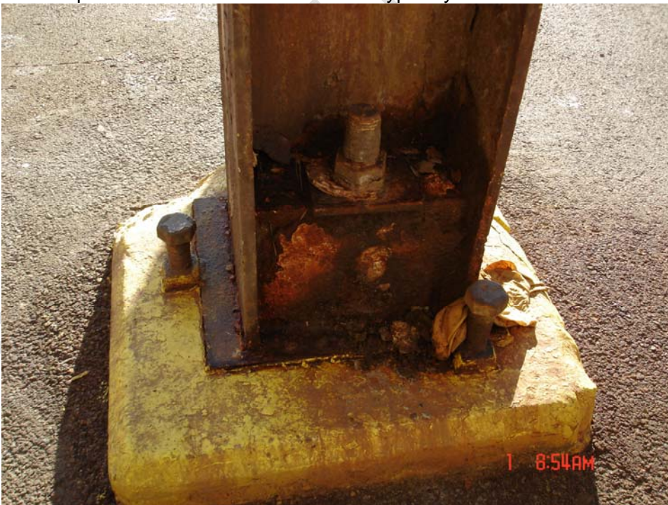
Unit 1 Column Line H-2
