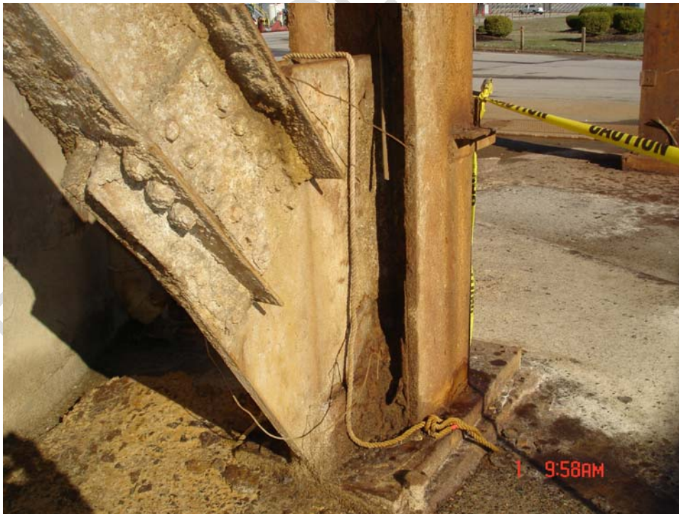
Unit 2 Column Line Gc-24
