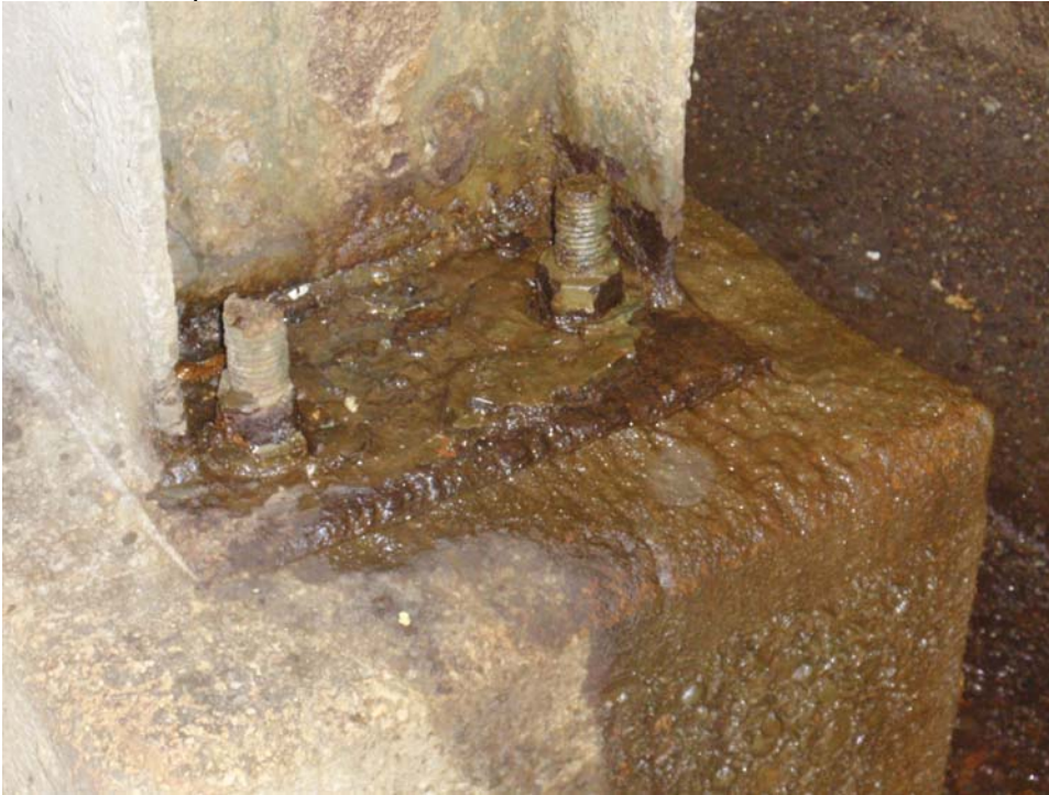
Unit 4 Column Line N-6B
