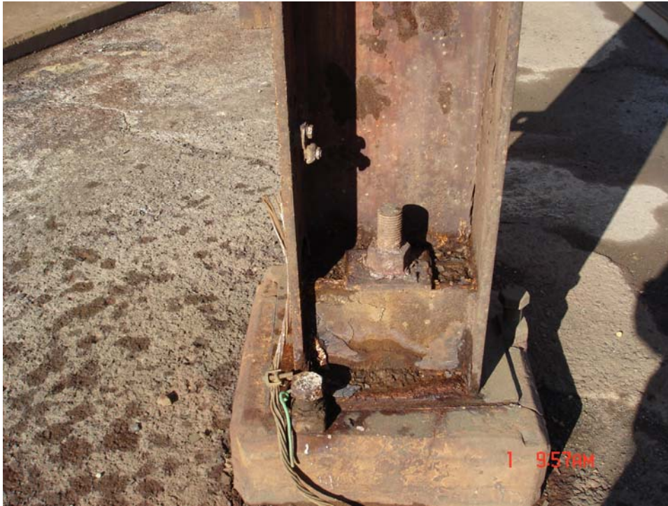
Unit 2 Column Line Gc-25
