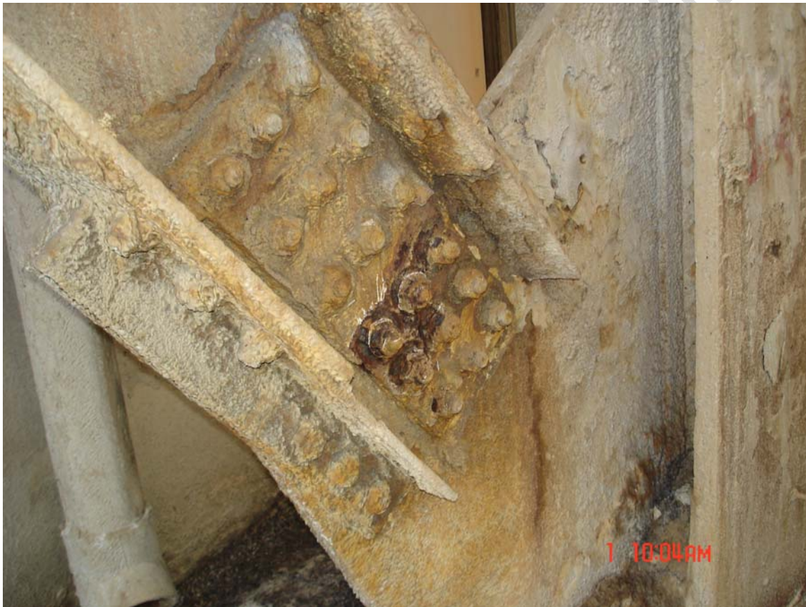
Unit 2 Column Line Ec-19
