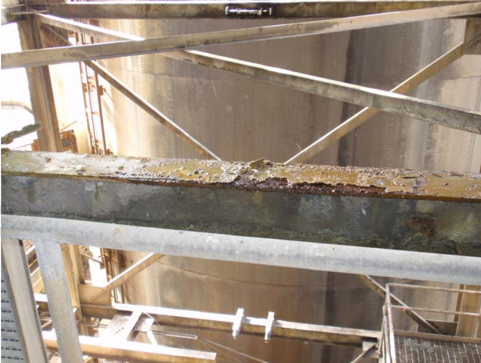
Unit 4 Column Line N about elevation 500
