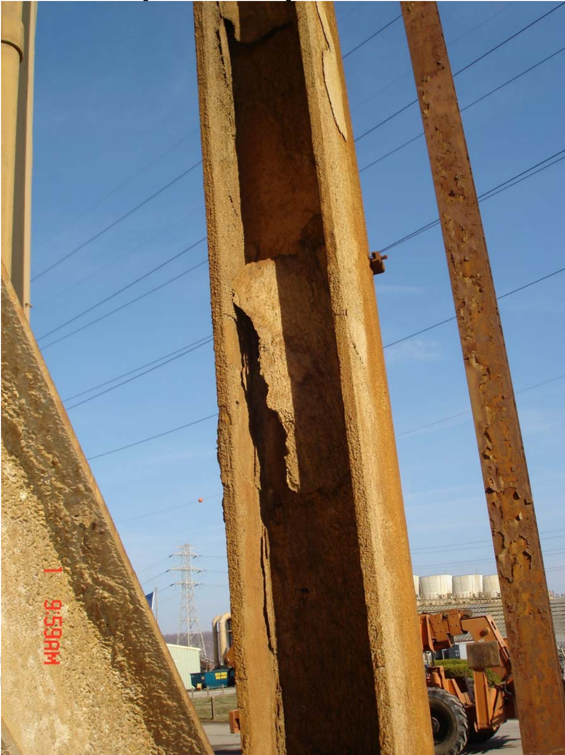
Unit 2 Column Line Gc-24
