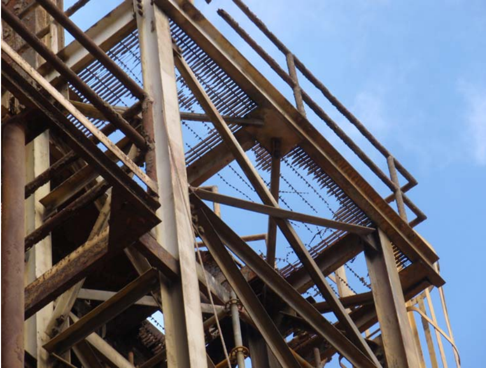
Unit 4 Upper level grating platform.
