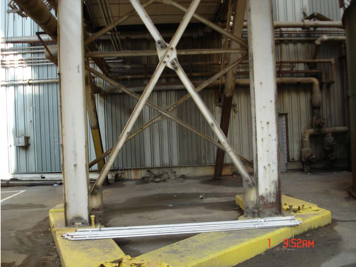
Unit 1 Column Line A-0.1 and A-0.2
