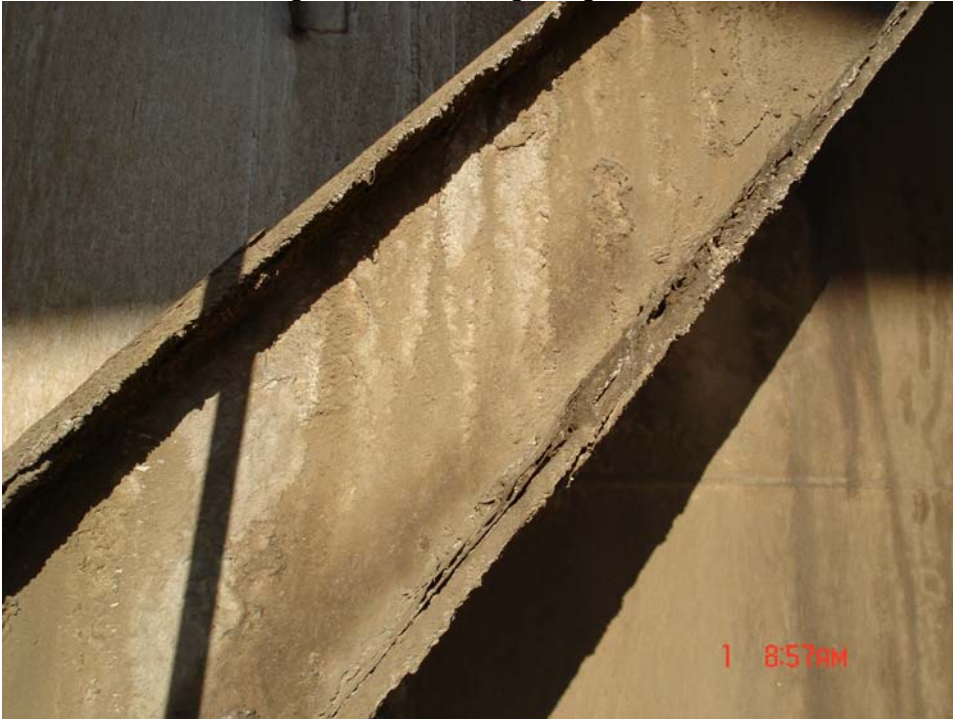
Unit 1 Main Bracing between Column Line H-3 and H-7
