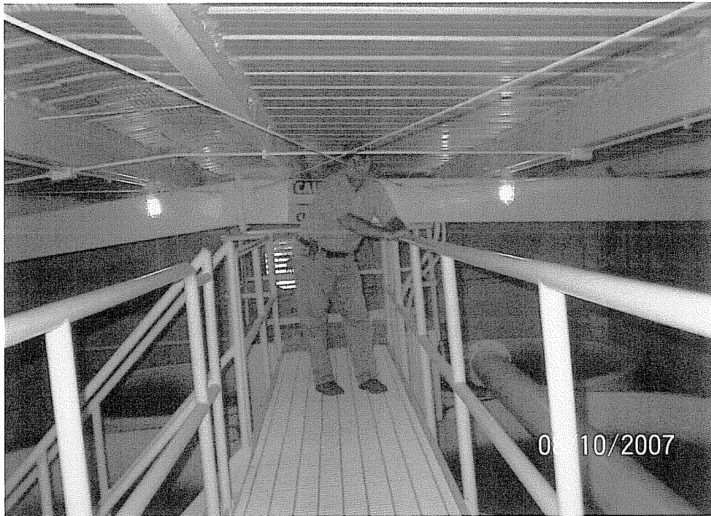
This is catwalk over filter tanks. The building was built with too low a ceiling height . Operators cannot stand up while on catwalk, and must stoop or bend to avoid hitting head on beams and electrical conduit. Lighting over filters is inadequate.
