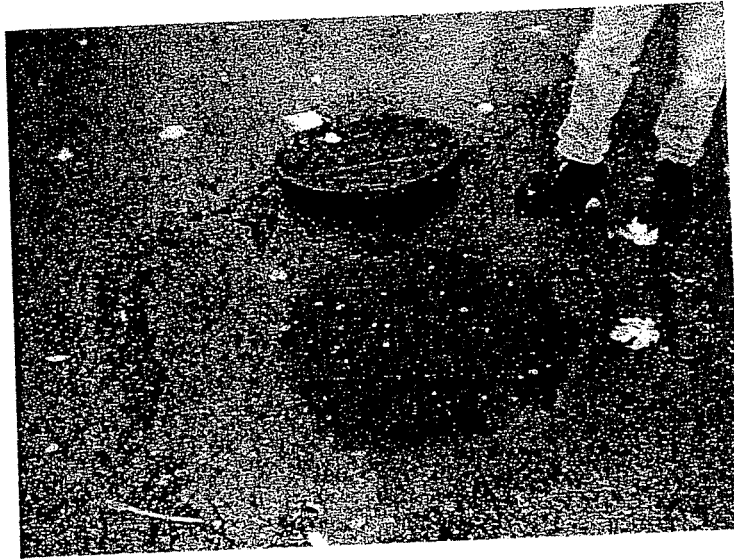
Photo 4 Manhole #2 with Cap in Place
