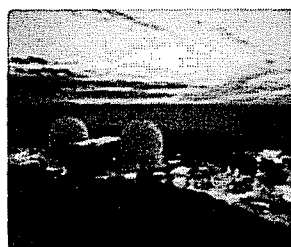
Donald C. Cook Nuclear Power Plant, Michigan
