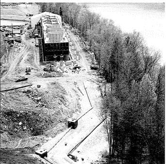
F.E. Moran has completed the installation of the sprinkler piping and the control building for the tower fire protection system. Viking will oversee the installation of the fire protection system in the service building and the supply line from the plant.
