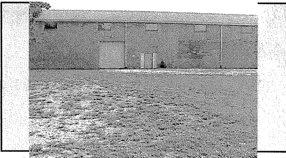
VIEW OF FRONT OF SITE OFF ROAD
